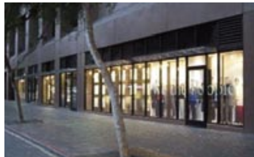
Edward J. Schwartz Federal Building, San Diego, CA, before (top) and after.
