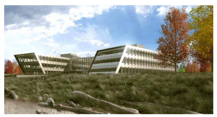
The vertical and horizontal sunshades are tuned to latitude and orientation to increase glazing performance and add an additional layer of texture to the building facade.
