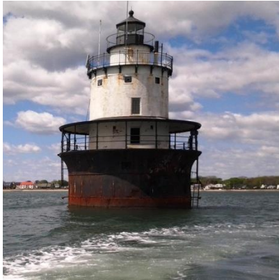
Butler Flats Light, New Bedford, MA Photo: Tiffany Shabanian, GSA
