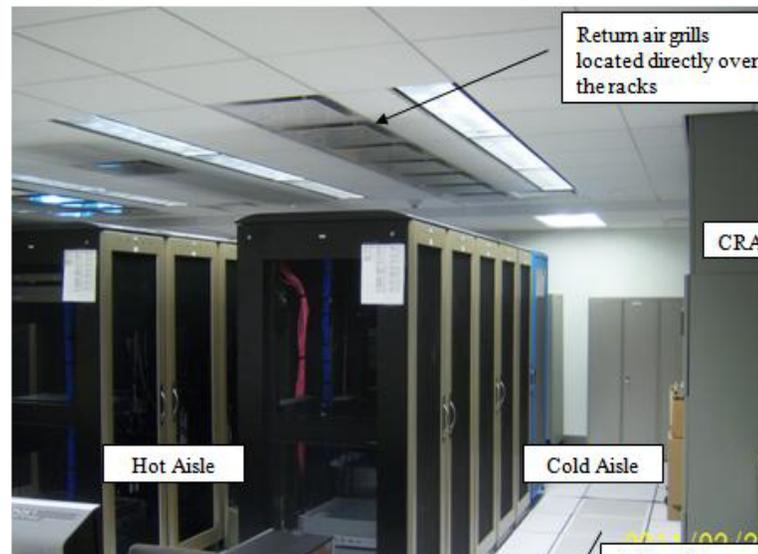
Cold air is generated by two 15-ton capacity Liebert Computer Room Air Conditioning (CRAC) units. Cool air is distributed through an under-floor system and discharged in front of the racks via perforated tiles.
