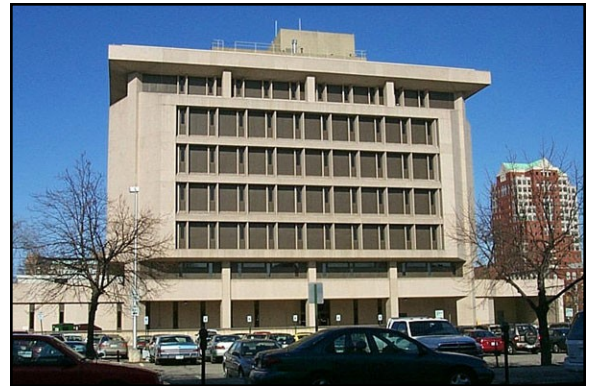
Norris Cotton Building before the window renovations.
