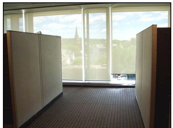
Interior view of the new windows.
