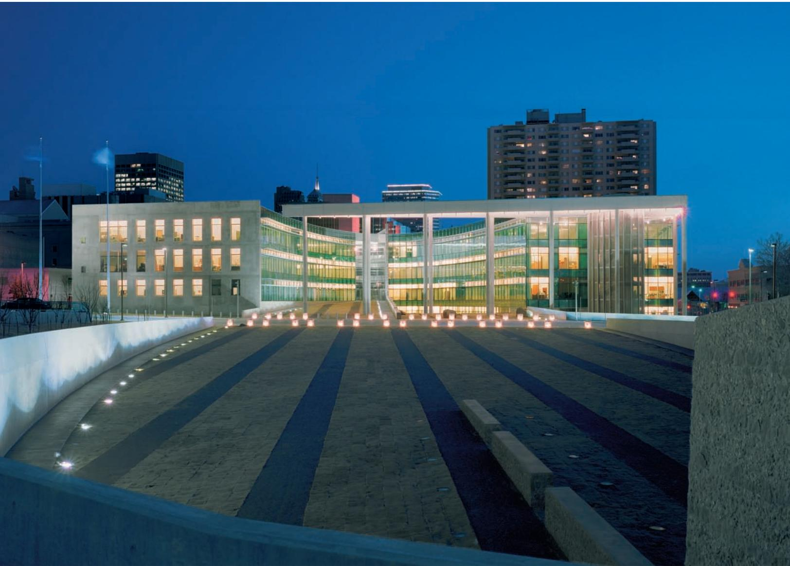
curtain wall is recessed behind a colonnade and deep roof overhang to reduce heat gain. Floor plates are sized to maximize daylighting of office workstations, which are located no more than 59 feet from a window.
