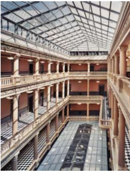
FIGURE 4 Include repair or replication of skylights concealed by previous roof repairs to improve the marketability of windowless workspaces.
