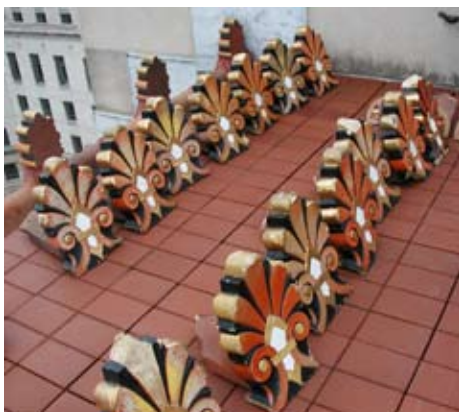
FIGURE 2 Damaged or missing features such as decorative acroteria should be repaired or replicated as part of a major roof project.
