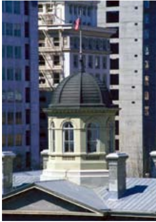
FIGURE 3 Repair and installation of slate, clay tile and metal roofing requires specialized construction skills. Competency of Restoration Specialist requirements reduce GSA risk by limiting competition to firms having successful experience with historic building projects of comparable complexity.
