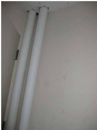
Chilled water pipes in closet, selected location for installing meters
