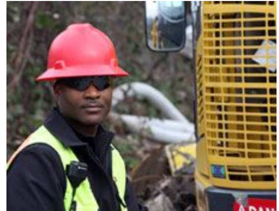
NWI Owner Michael Martin was proud of the clean and efficient work his crew did at EGWW and looks forward to additional work with McKinstry.
