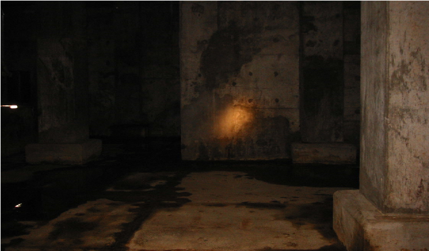
Photograph 37. Building 105 SAFR. Floor post-remediation, September 2002.
