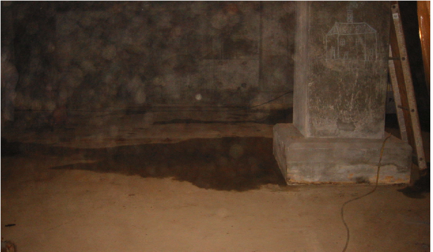
Photograph 29. Building 105 SAFR. After demolition and pressure washing, September 2002.
