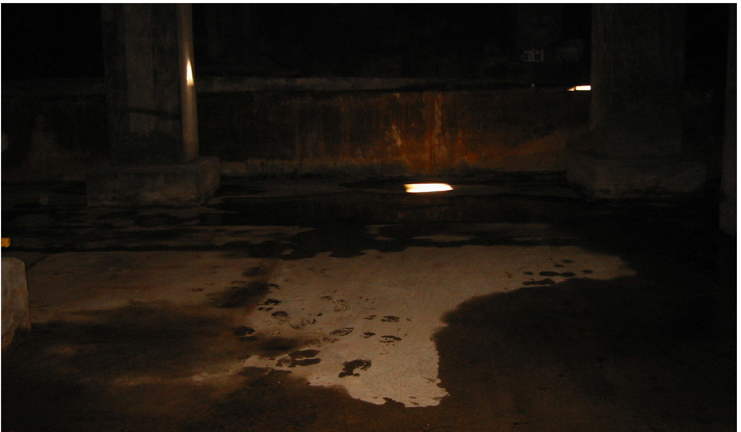
Photograph 36. Building 105 SAFR. SAFR floor post-remediation, September 2002.
