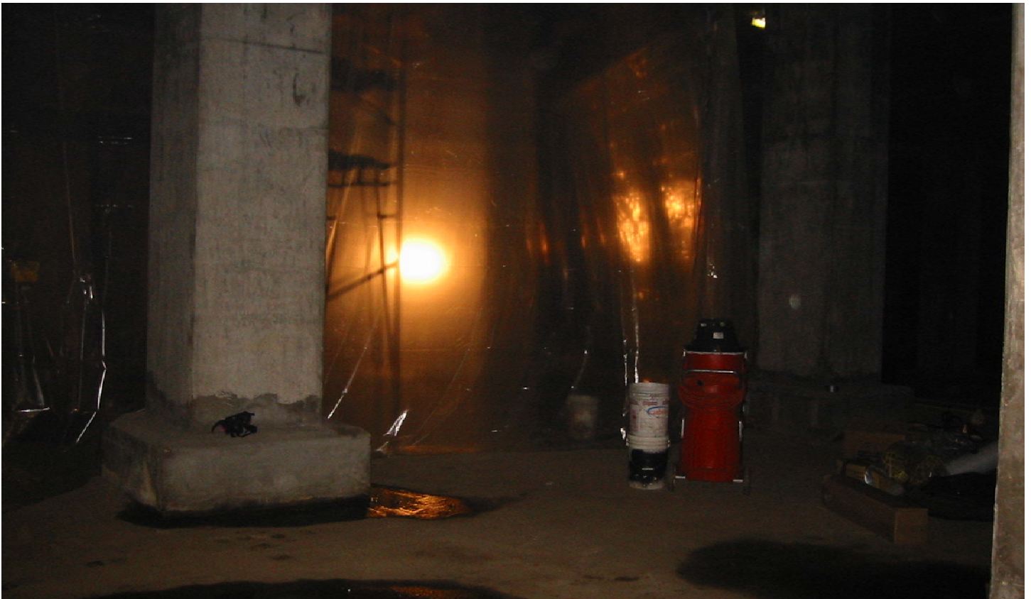
Photograph 30. Building 105 SAFR. Post remediation, after washdown, September 2002.
