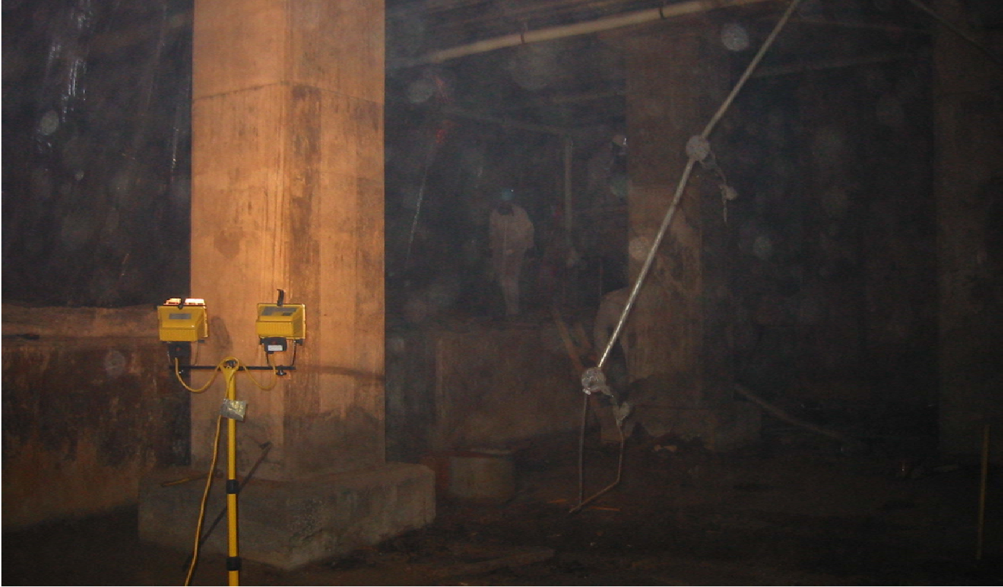
Photograph 26. Building 105 SAFR. Lighting of containment during waste loadout, September 2002.
