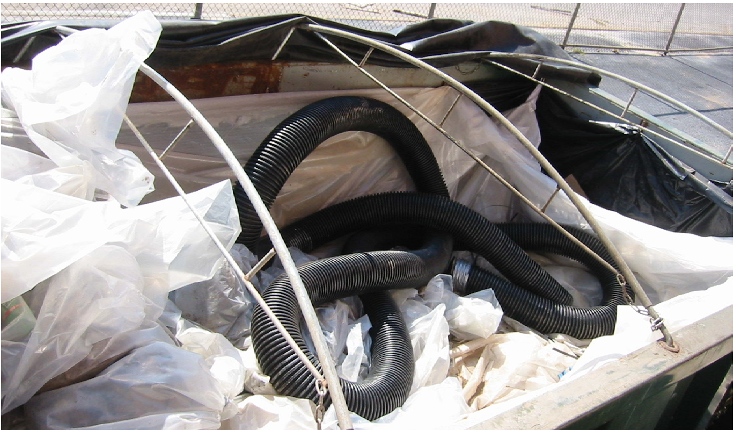
Photograph 20. Building 105 SAFR. Hose used to remove sand from basement; disposed as hazardous wastet, September 2002.
