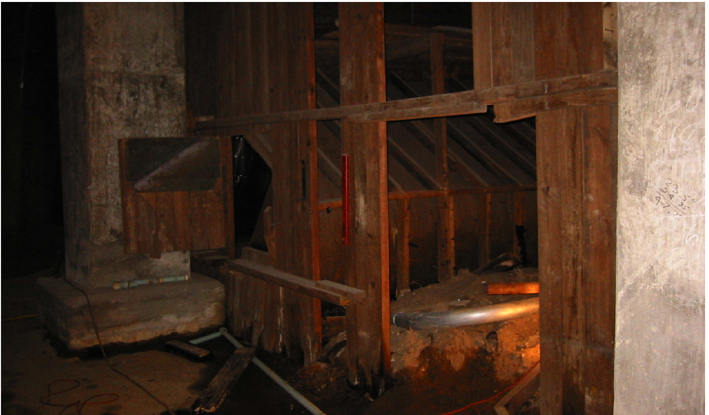
Photograph 13. Building 105 SAFR. Rear of SAFR prior to demolition, September 2002.
