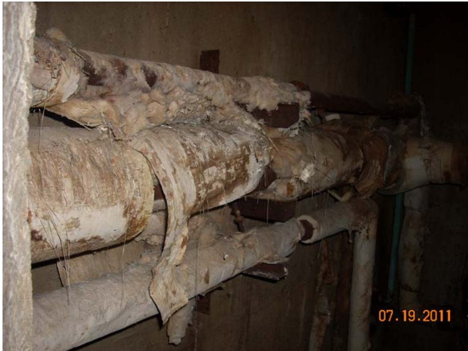
Photo #2: Pre-Abatement – Basement Air Handler Room (Thermal Pipe Insulation)
