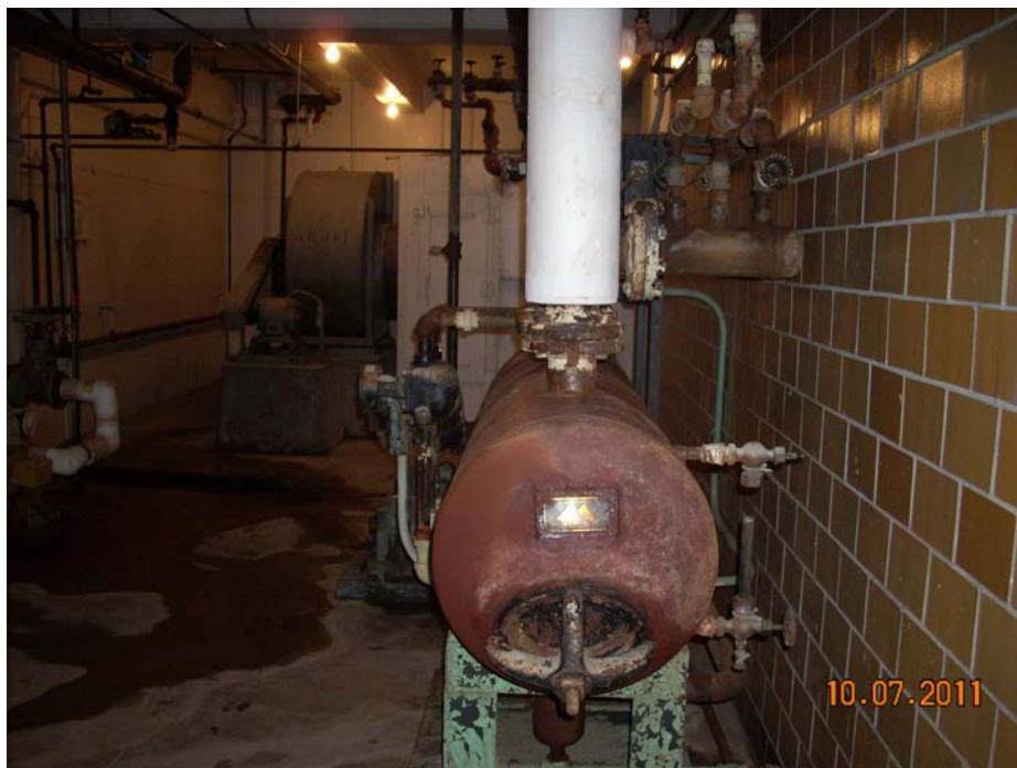
Photo #10: Post-Abatement – Air Handler Room (Tank Insulation Removal)
