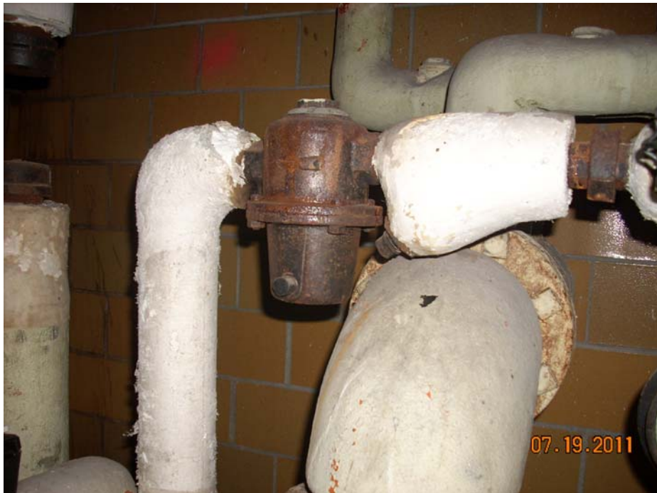
Photo #2: Pre-Abatement – Basement Air Handler Room (Thermal Pipe Insulation)
