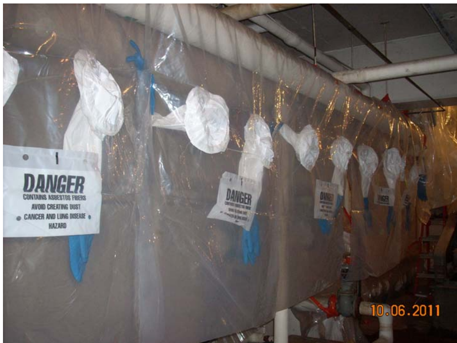
Photo #4: During-Abatement – Air Handler Room (Glovebag Removal)
