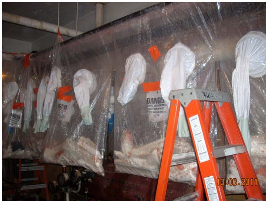
Photo #6: During-Abatement – Air Handler Room (Glovebag Removal)
