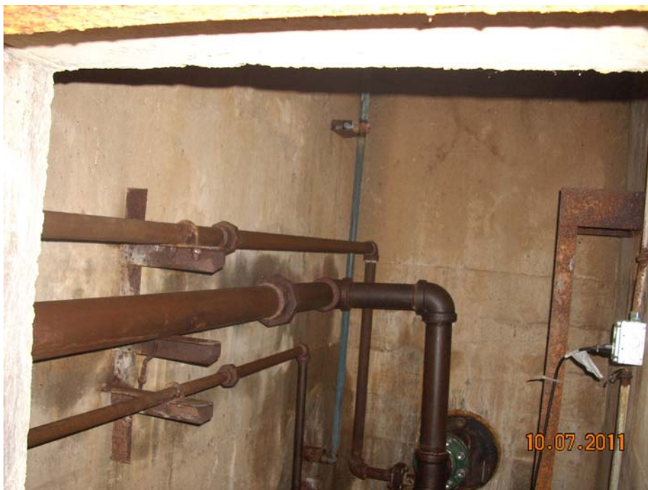
Photo #8: Post-Abatement – Air Handler Room (Glovebag Removal)
