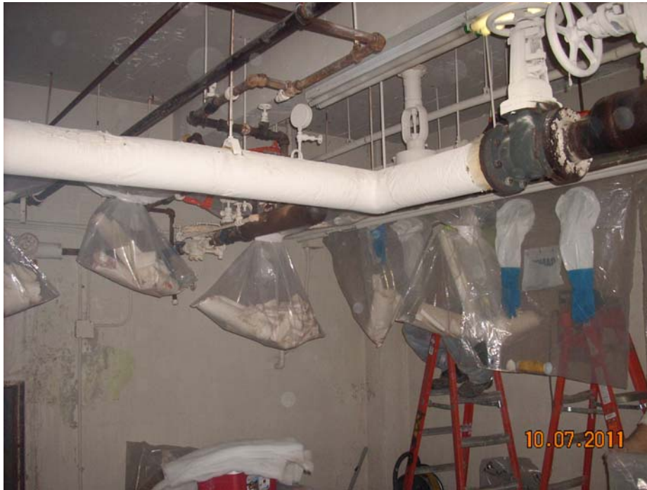
Photo #8: Post-Abatement – Air Handler Room (Glovebag Removal)
