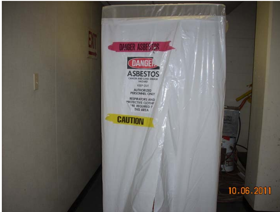
Photo #6: During-Abatement – Air Handler Room (Glovebag Removal)
