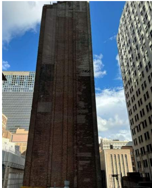
Photo 4. Overall West Elevation
