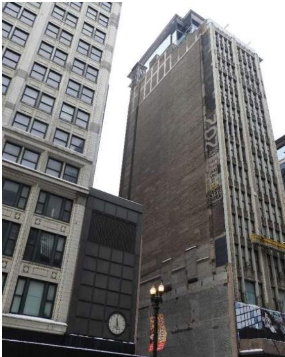
Photo 3. Overall South Elevation
