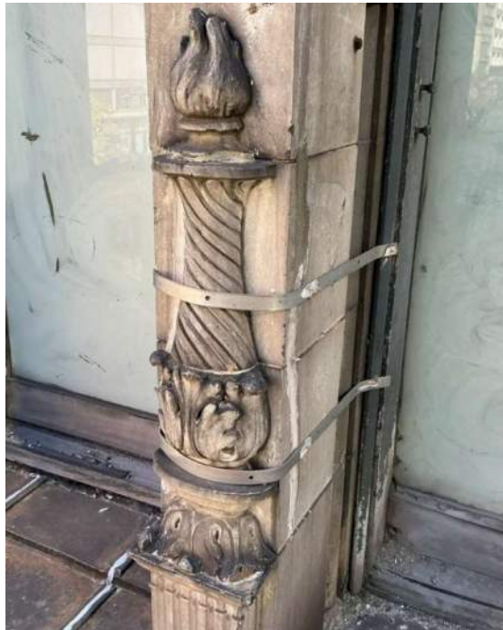
Photo 9. Mullion unit at 3 rd floor with previously installed straps
