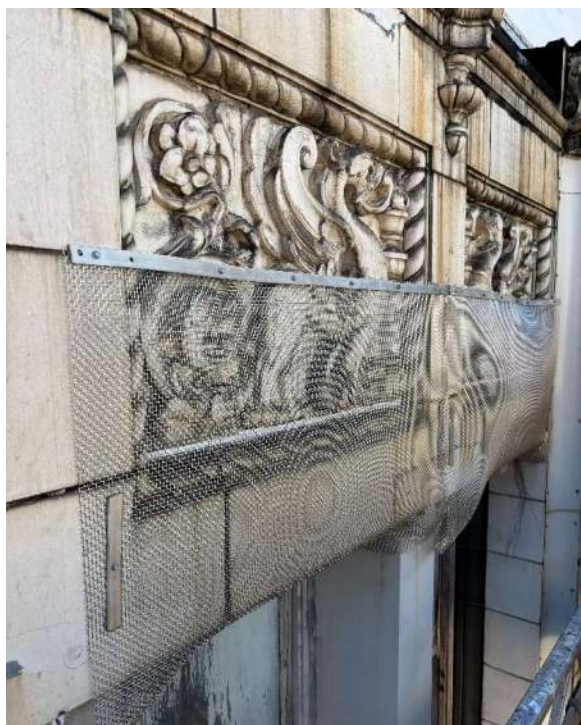
Photo 5. Lower portion of original cornice throughout north and east elevations – now removed.
