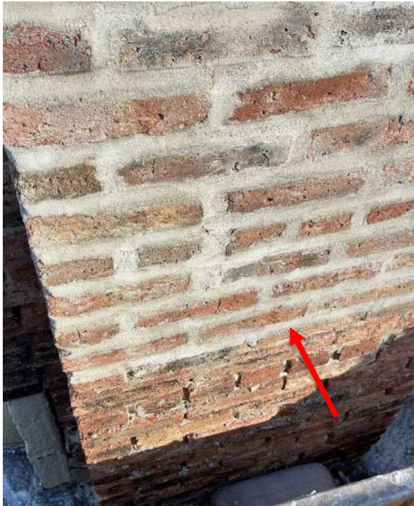
Photo 29. Typical brick repointing at West Elevation
