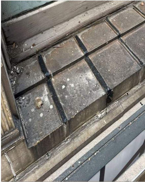
Photo 13. Sealed skyward joints at windows
