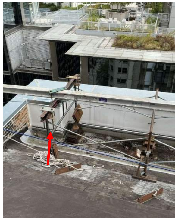
Photo 20. Steel columns encased in newly-constructed parapet wall.
