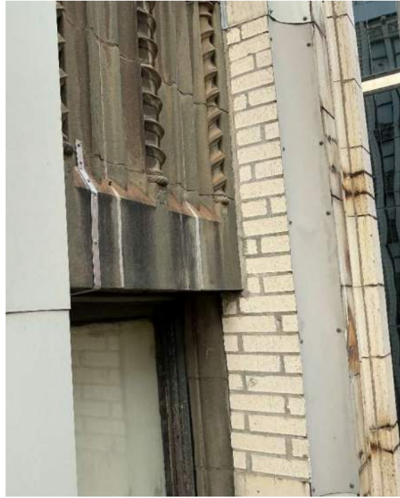
Photo 14. Replacement of terra cotta units with brick masonry
