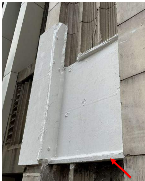
Photo 28. Typical plywood cover replacement
