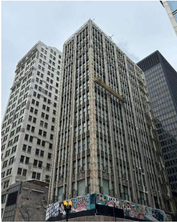
Photo 1. Overall North Elevation
