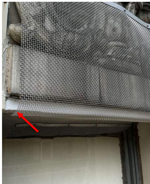
Photo 24. Typical mesh and painted horizontal metal channel repair
