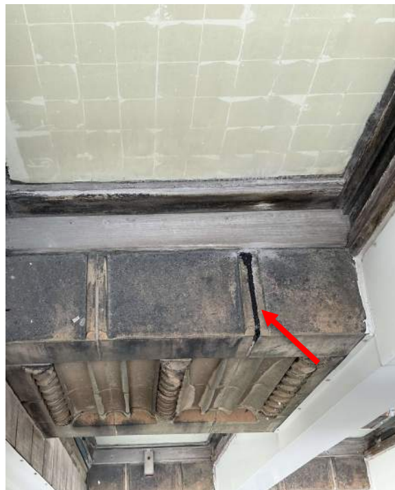
Photo 26. Typical skyward facing joint sealant repair
