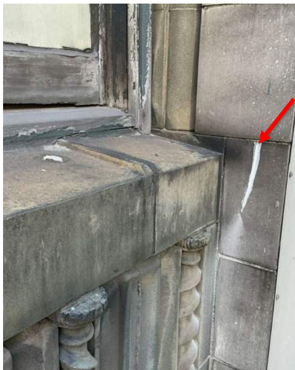
Photo 23. Typical terra cotta rout and seal repair
