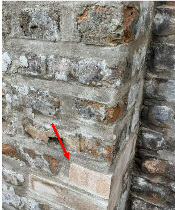
Photo 30. Typical brick replacement at West Elevation.
