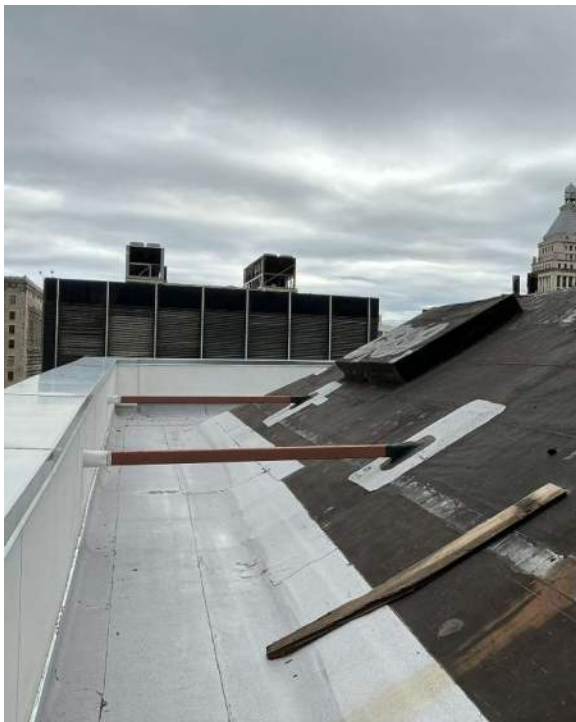
Photo 19. Newly-constructed parapet wall with metal coping and roof flashing.
