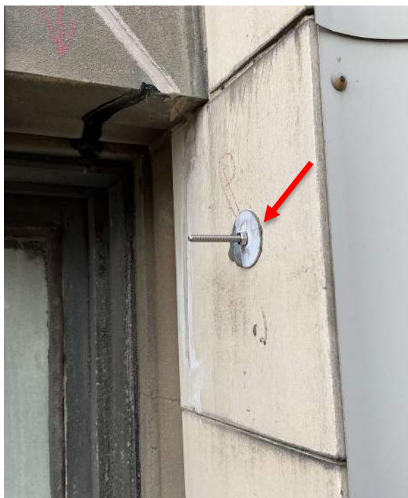
Photo 27. Typical installation of supplemental metal pins
