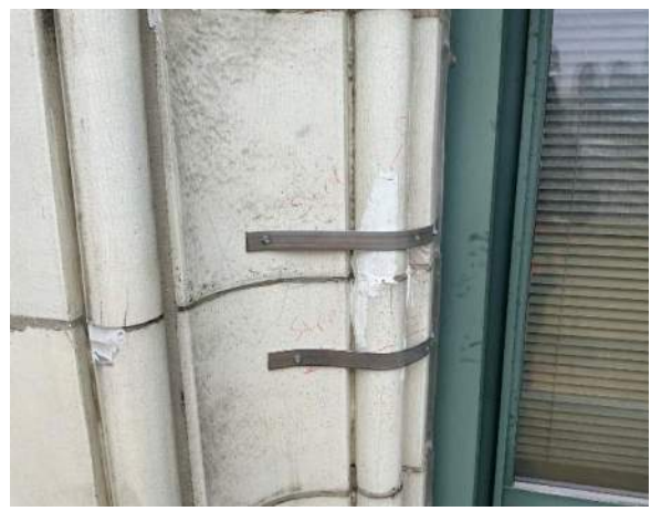
Photo 36. Typical stainless steel strap installation.
