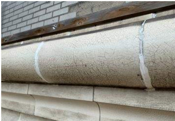
Photo 33. Open mortar joint sealed with polyurethane sealant.
