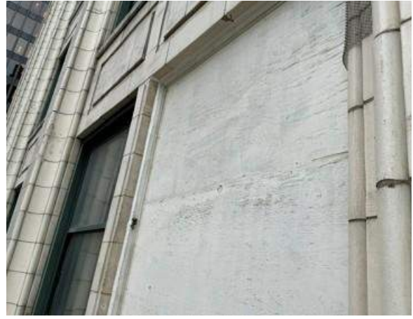
Photo 38. Existing plywood over window in good condition, scraped and repainted.
