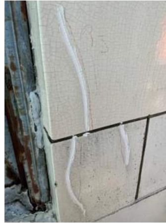
Photo 44. Typical route & seal repair.
