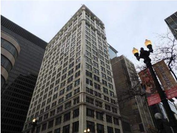
Photo 1. Overall elevation of the east and south façade.
