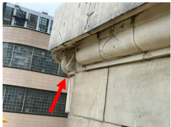
Photo 6. Previously removed water table piece at the northeast corner of the building, cracks routed and sealed.
