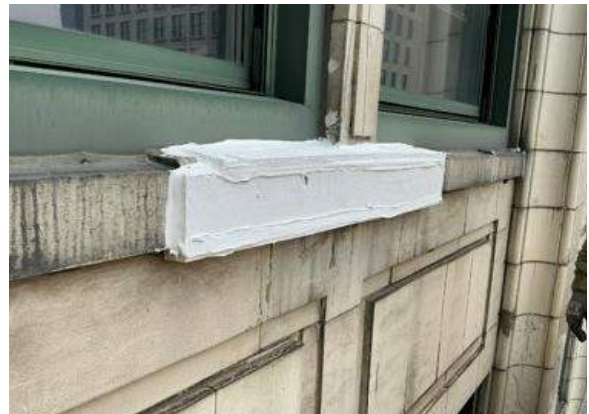
Photo 34. Typical plywood covering at removed terra cotta sill unit.
