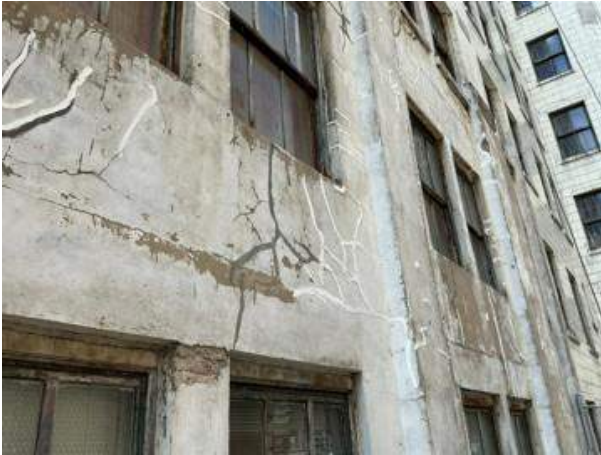
Photo 43. Typical cementitious parge coat sealant repair at north elevation.
