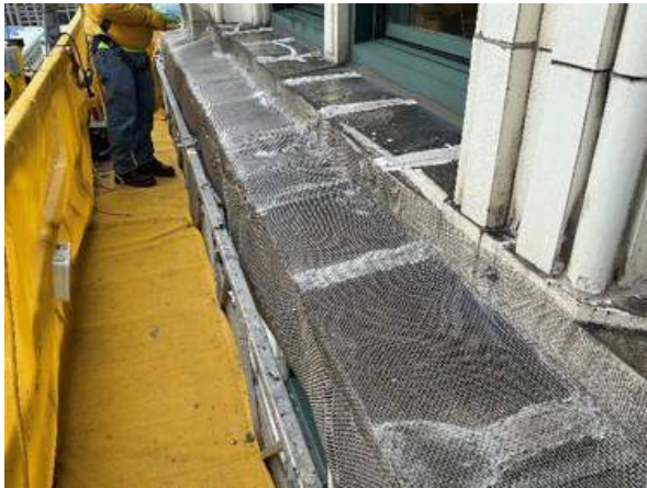
Photo 31. Previously installed mesh at the east elevation water table.
