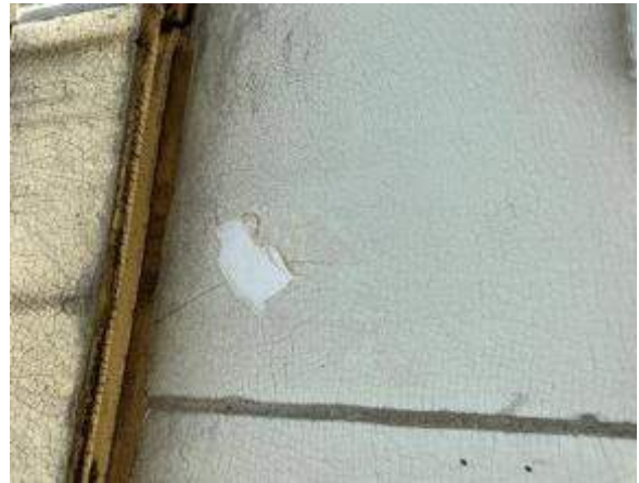
Photo 32. Typical sealant repair at spalled glaze.
