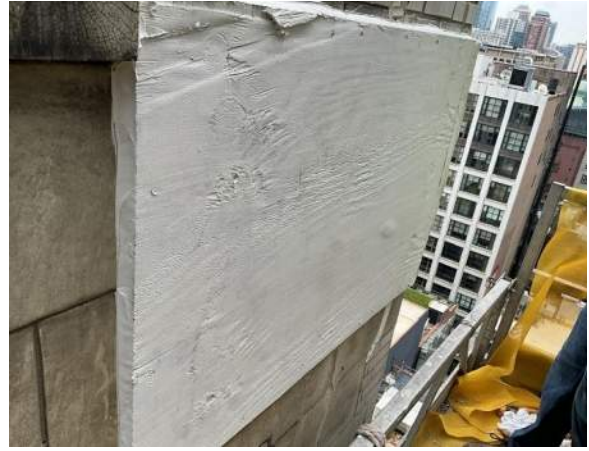
Photo 50. Plywood cover at removed water table corner pieces at west elevation, 18 th floor.
