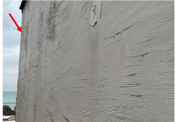
Photo 20. Existing plywood covering at the north elevation parapet.
