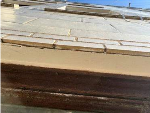
Photo 37. Existing steel at the window heads, cleaned and recoated with a corrosion-inhibitive coating.
