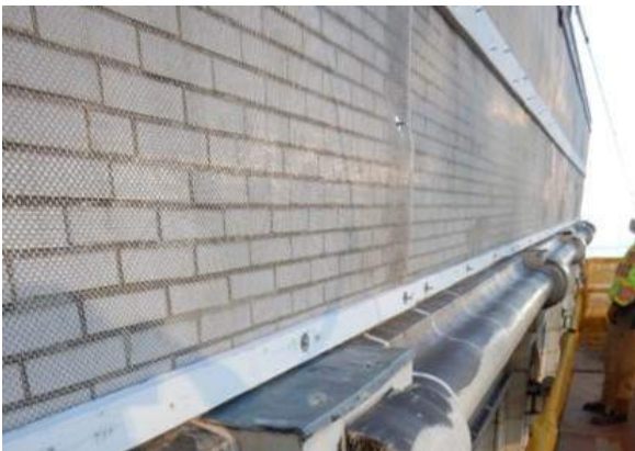
Photo 3. Typical cornice throughout east and north elevations.
