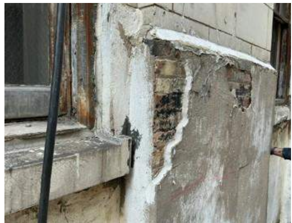
Photo 42. Typical unsound cementitious parge coat removal and sealant installation at north elevation.
