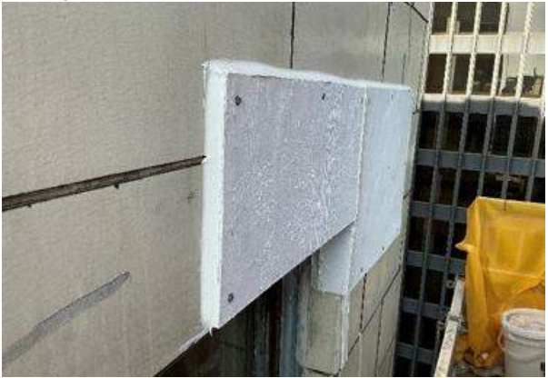
Photo 39. New plywood coverings over removed unsound material.
