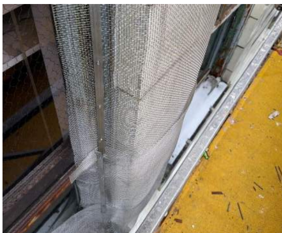
Photo 35. Typical stainless steel mesh installation.
