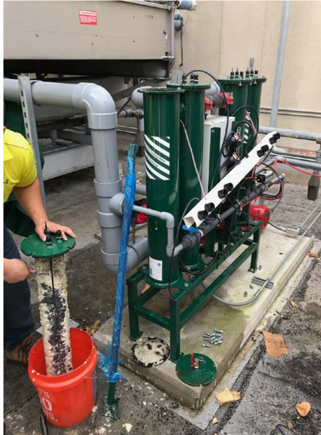
Figure 1. Scraping scale off the reactor rod of the electrochemical water treatment system.
