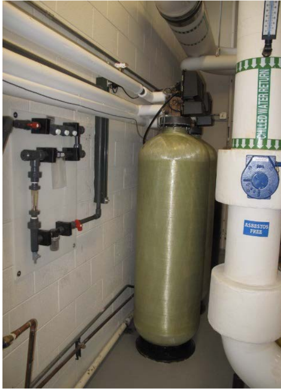
Figure 3. Brine tank of the salt-based ion exchange system
