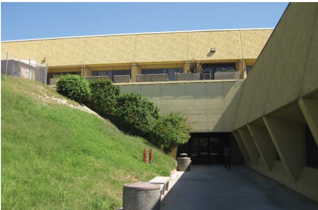
Image 17: A secondary building entrance on the west facade.
