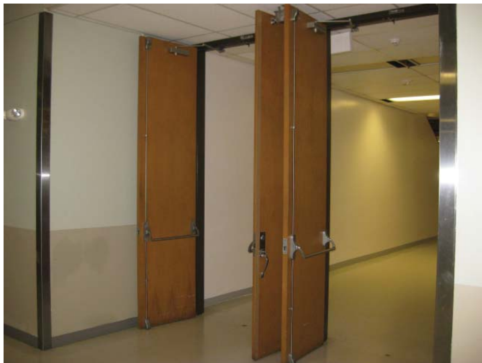
Image 25: Typical original interior flush wood doors on the first floor.
