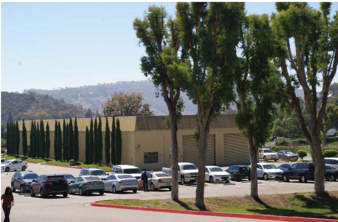
Image 19: A detached storage and maintenance building to the west of the loading area. This building was constructed at the same time as the main building, but it does not share the same architectural detailing.
