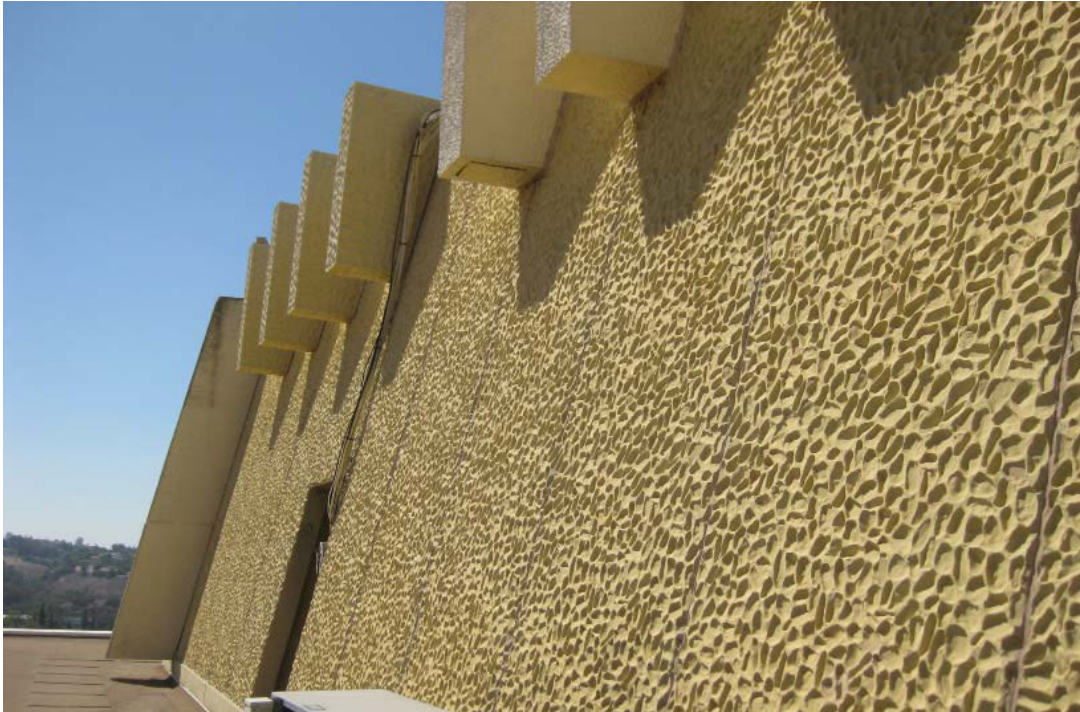
Image 42: The sixth floor roof. Textured fiberglass fins have been added to conceal some of the added equipment on the upper edge of the roof.
