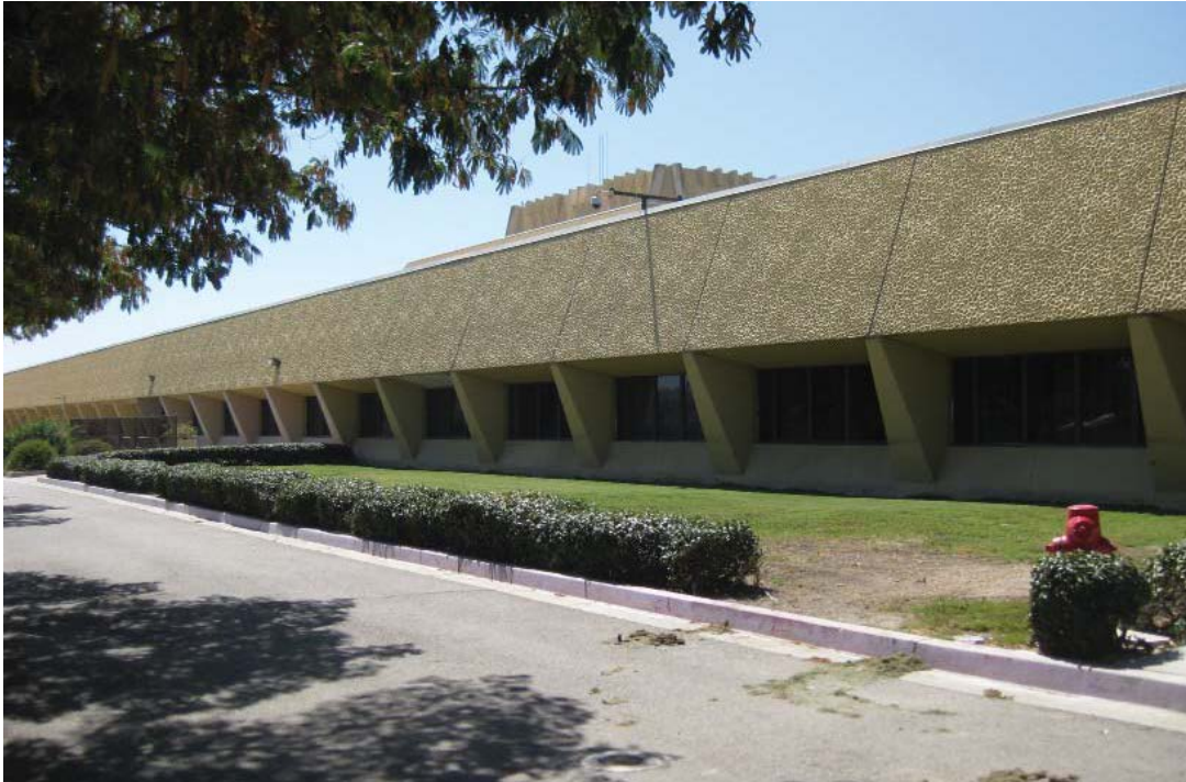
Image 12: The east facade looking southeast.
