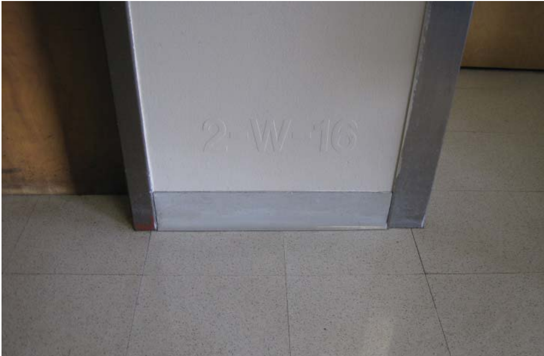
Image 30: A numbered structural column. The numbers corresponds with the original drawings and can be found on structural columns throughout the building.
