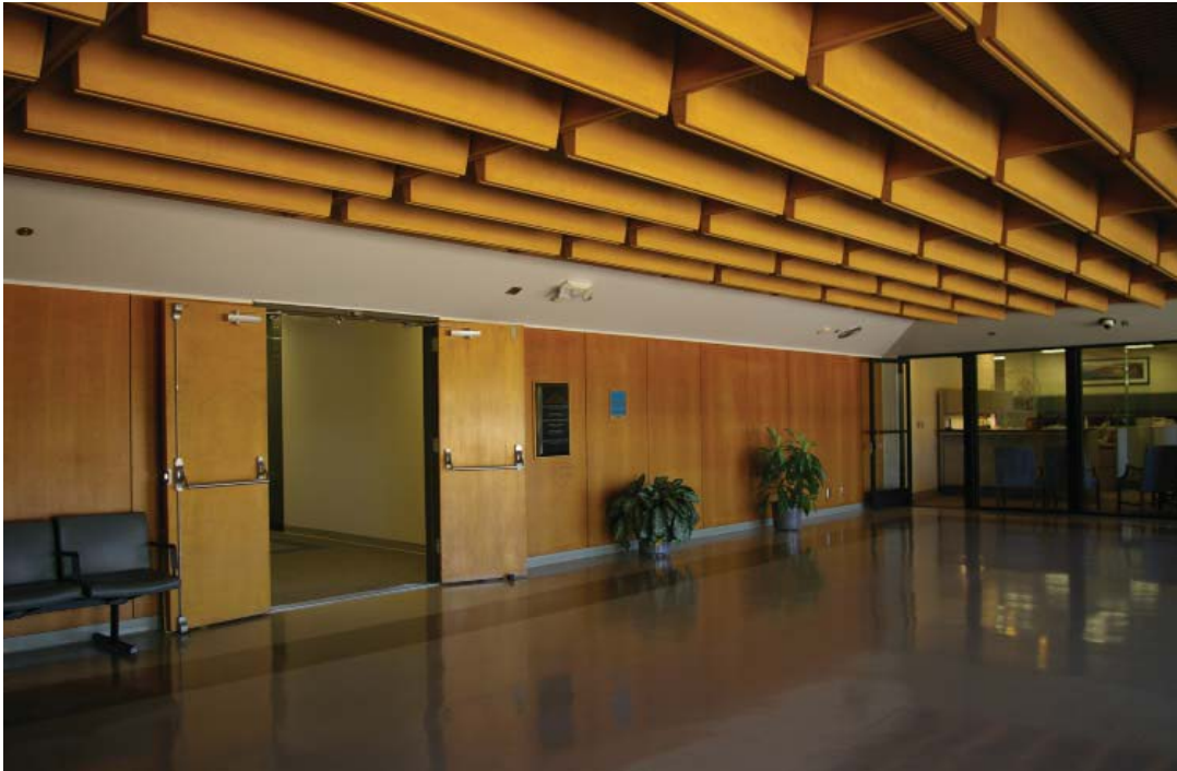
Image 40: The original main lobby on the fourth floor. This space features original wood wall paneling and a decorative wood ceiling finish.
