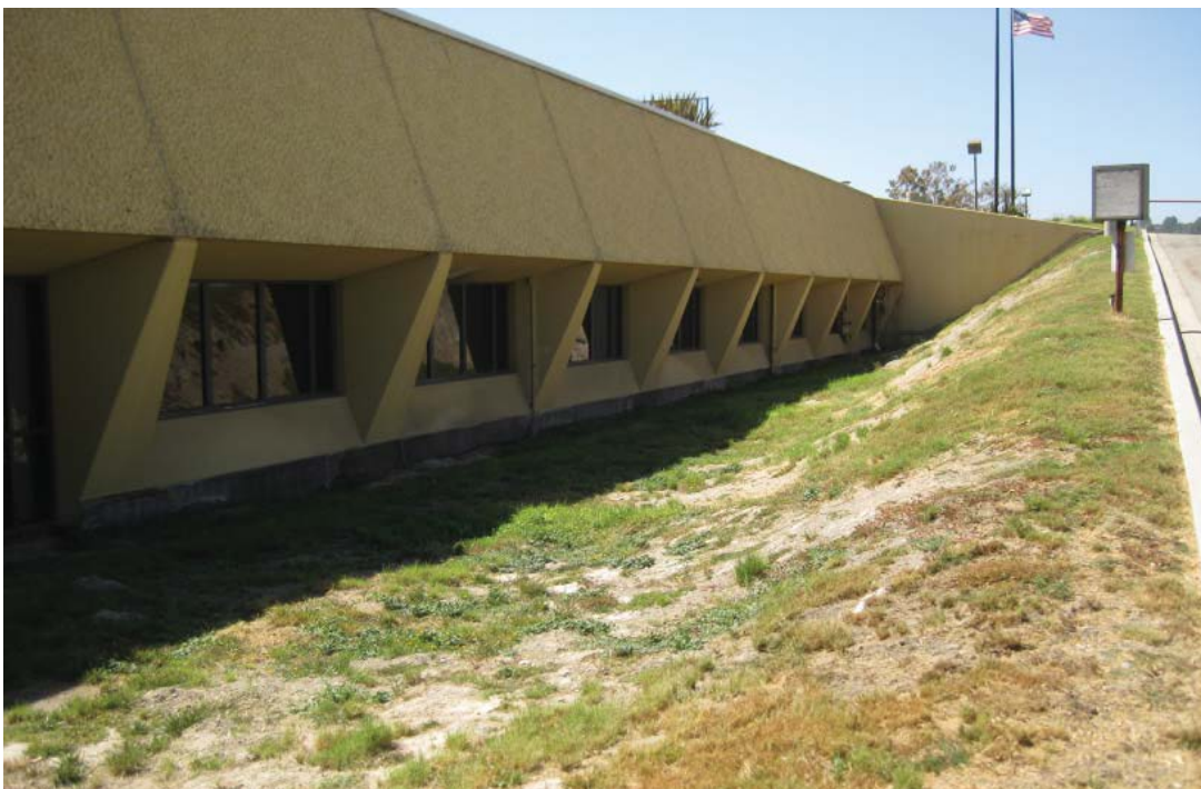
Image 11: The north wall of the third floor looking west.
