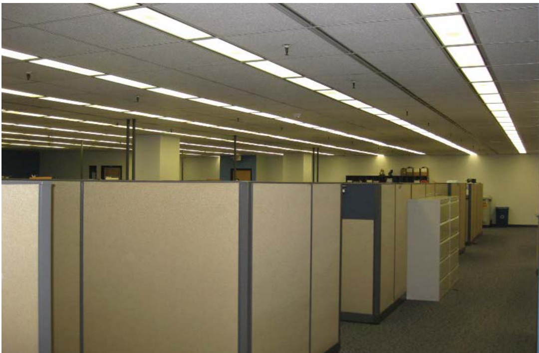
Image 39: A typical office area on the third floor. The ceiling appears to be original but other finishes and fixtures have been replaced.
