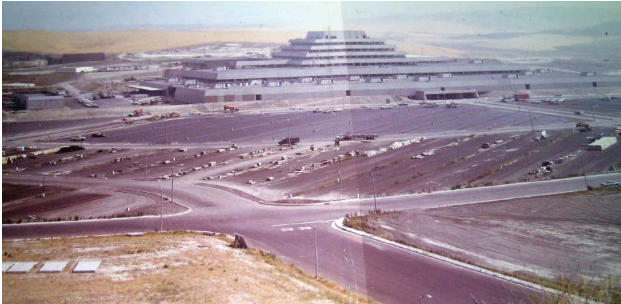
Image 6: The Chet Holifield Federal Building looking northeast ca. 1970s. This early color photo shows the original gray color of the exterior. (Source: General Services Administration)
