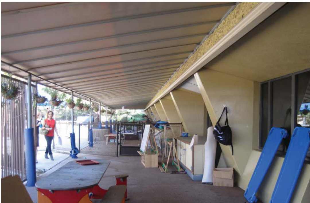
Image 37: The child care center on the third floor. A new sheet metal shade canopy has been added on the original exterior wall.
