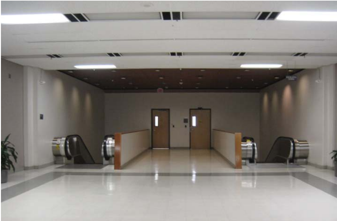
Image 34: The escalators on the second floor. The suspended ceiling and wood ceiling finish are original.
