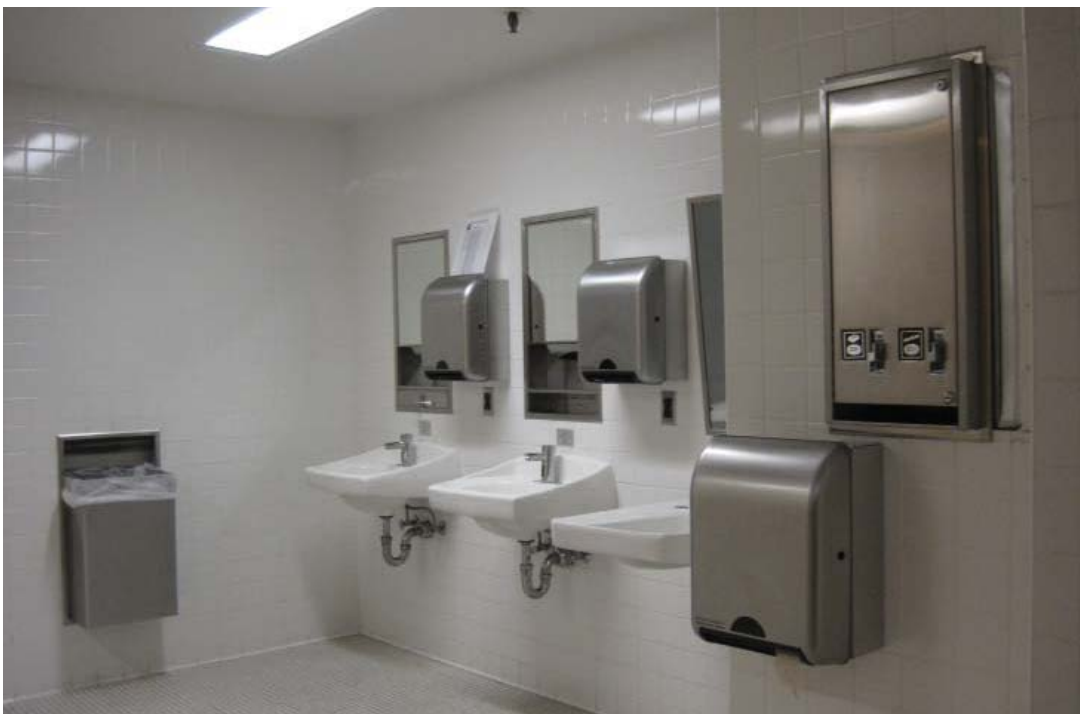
Image 33: A typical restroom on the second floor. Finishes, fixtures, toilet partitions, and accessories have been replaced.
