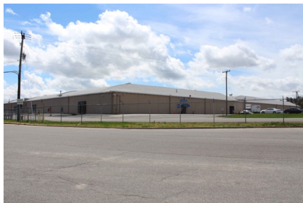
GSA Warehouse Property (VDHR ID: 029-5876), facing SE along Metropolitan Center Drive (Source: EHT Tracerics, Inc.)
