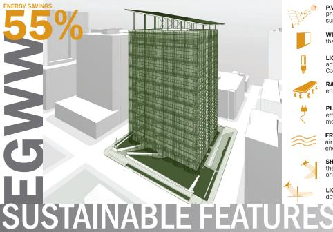
**P.V. PANELS** - The renovation of the EGWW building includes 13,000 sf of solar photovoltaics on a 25,000 sf canopy which also doubles as a water collection surface. The solar array is expected to produce 200,000 kWh of energy annually.
