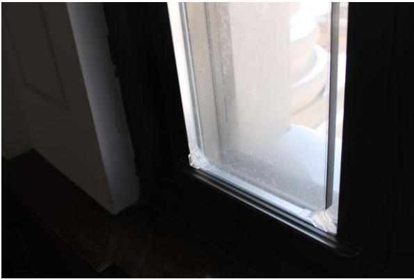
(e) There is a small gap between the window panel and the overall frame.
