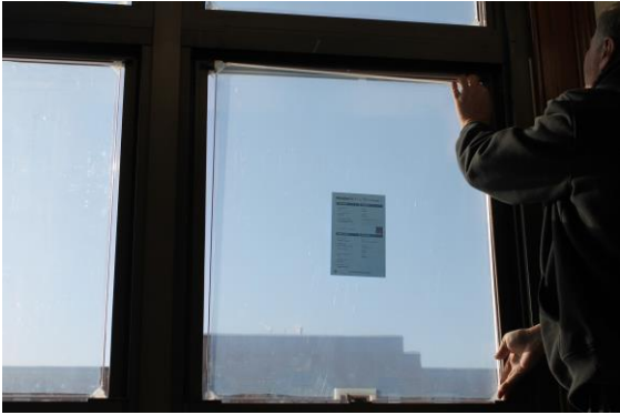
(b) Window panels around the window lock in a first-floor office (May 1, 2023).
