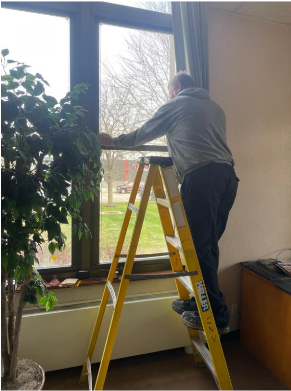
(c) Window insulation panel above the window is removed.
