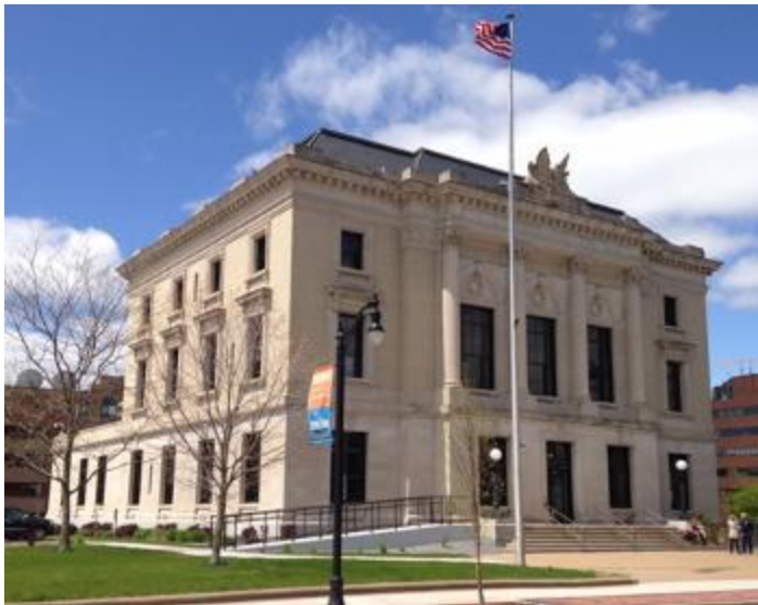
Figure 4. Exterior of the Eau Claire Courthouse.
