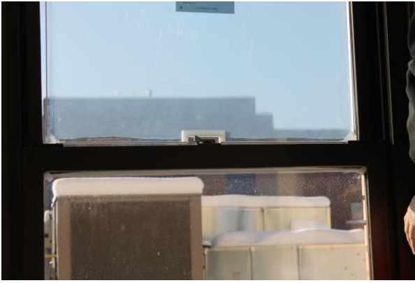
(a) Window lock would strike the panel above if the window opened.
