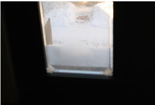
(a) Condensation on the windows in the second-floor courtroom.
