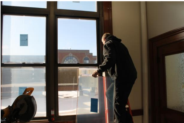
(a) Corner mounts are placed in the corner of each window lite.
