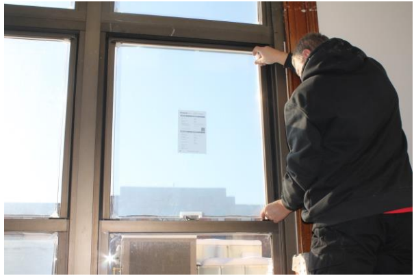
(d) Installer presses the insulation against the window mounts.
