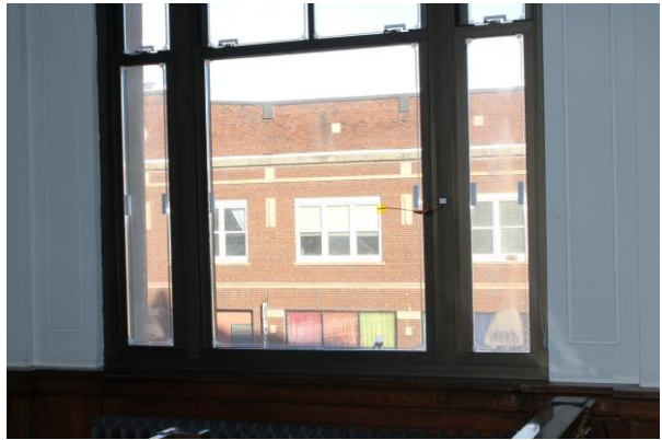
(f) Panel mostly disappears when viewed at a reasonable (>5 ft) viewing distance from the window.
