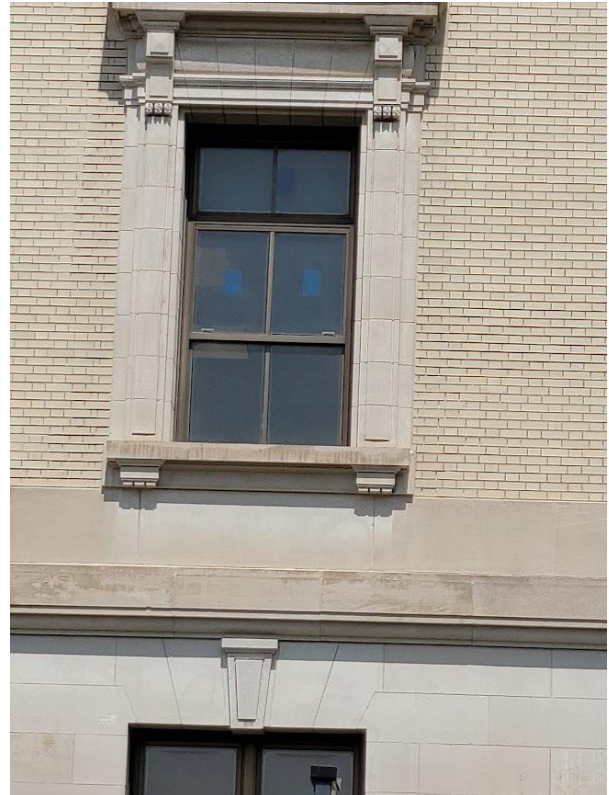
(b) Exterior photograph with a construction sticker visible (May 15, 2023).
