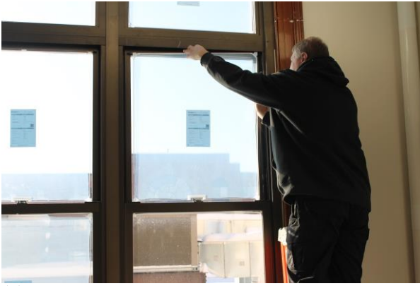
(c) Installer places a panel on the corner mount attachments.
