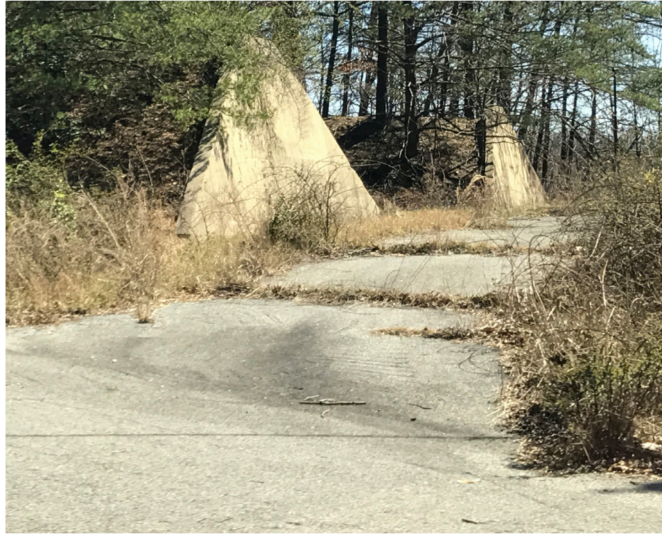
4 Concrete retaining walls for explosives magazines (removed)
