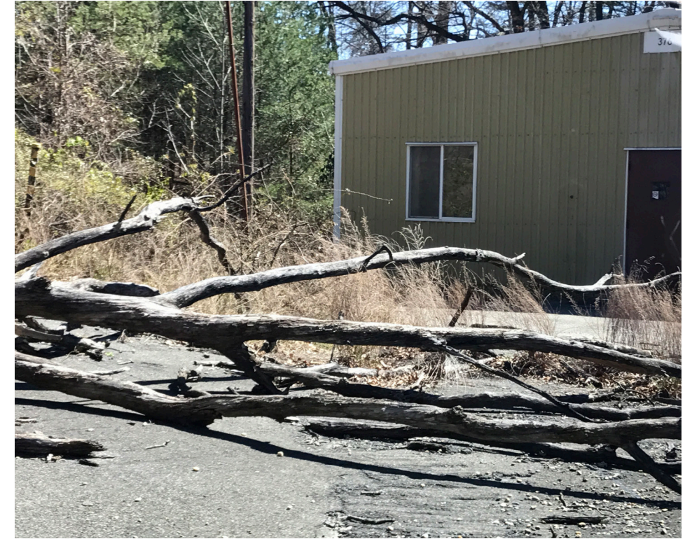
6 Former Air Blast Field Lab
