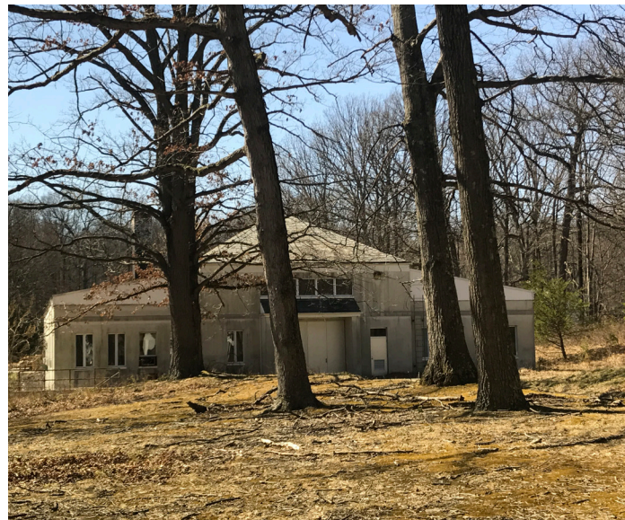
Former Magnetic Research Facility
