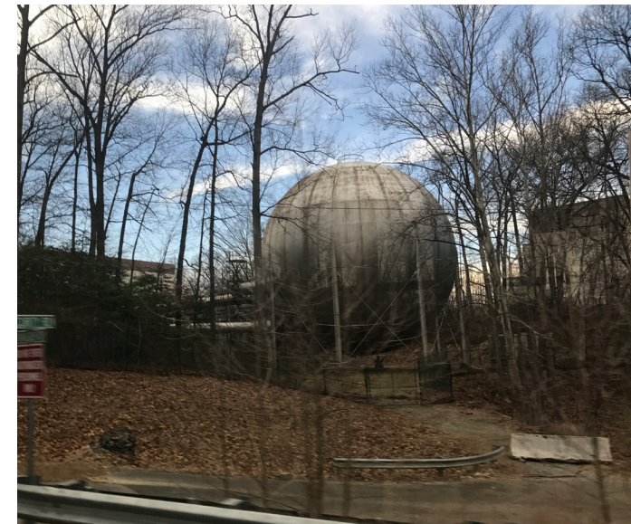
Current AEDC Wind Tunnel Facility
