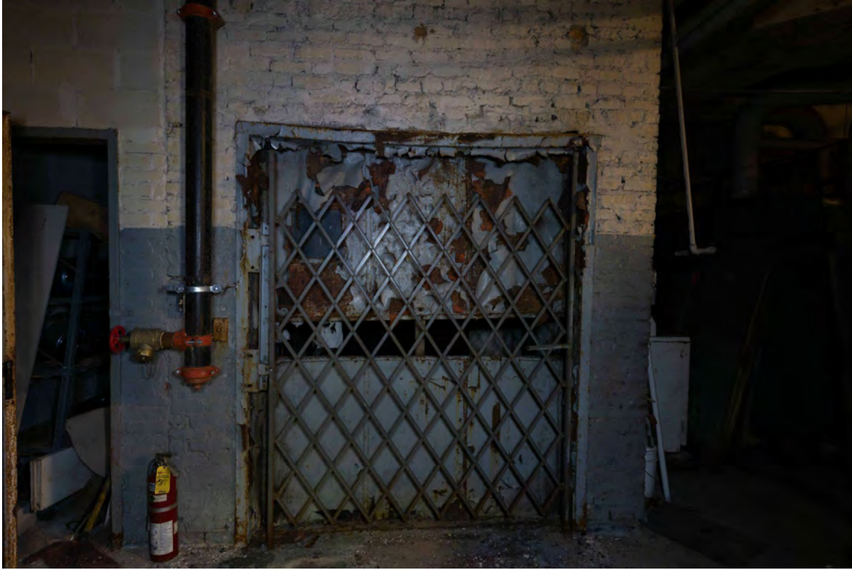
Lower Level 2 Freight Hoistway Opening
