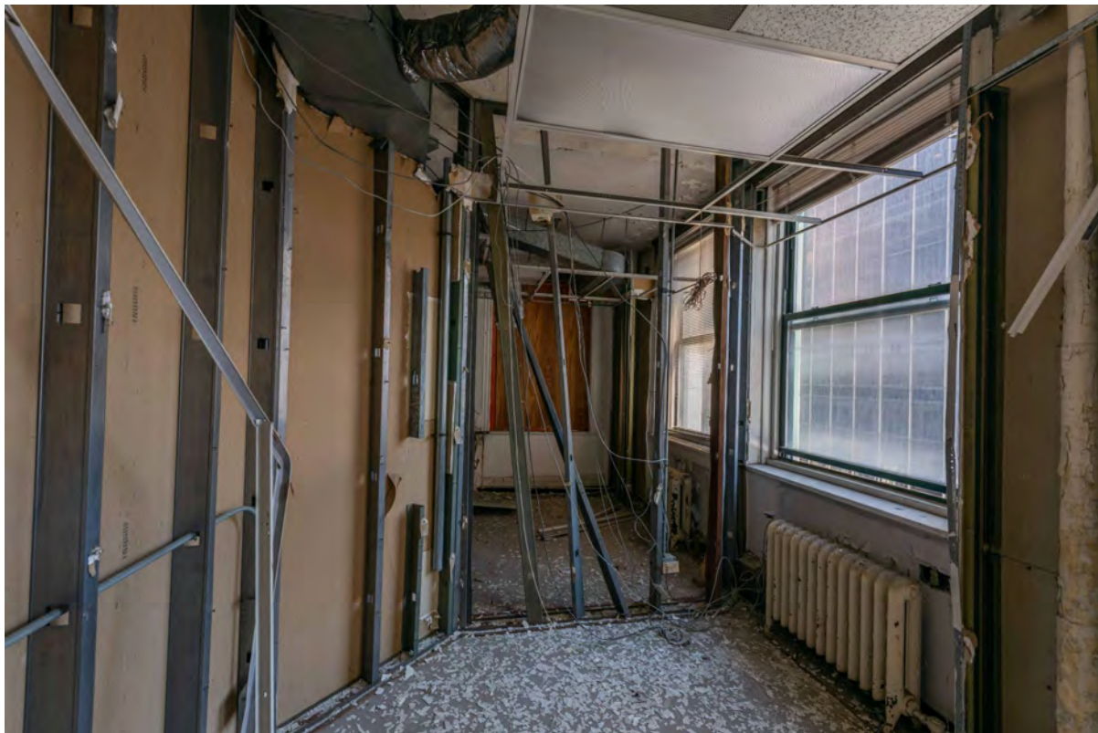
Level 6 Office Space Level 6 Freight Elevator Hoistway
