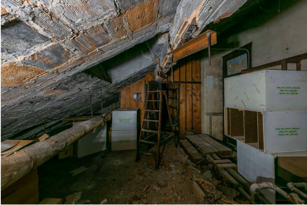
Level 22 Under Roof
