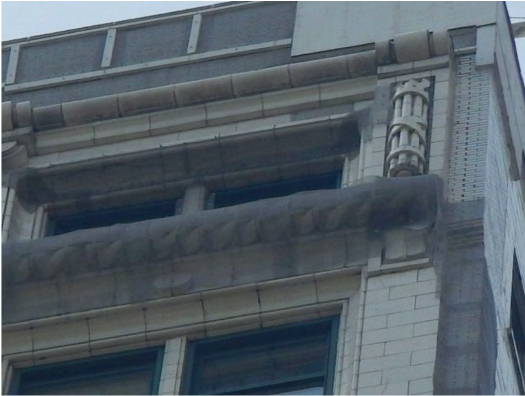
Overview of mesh installed at water table and building northeast corner
