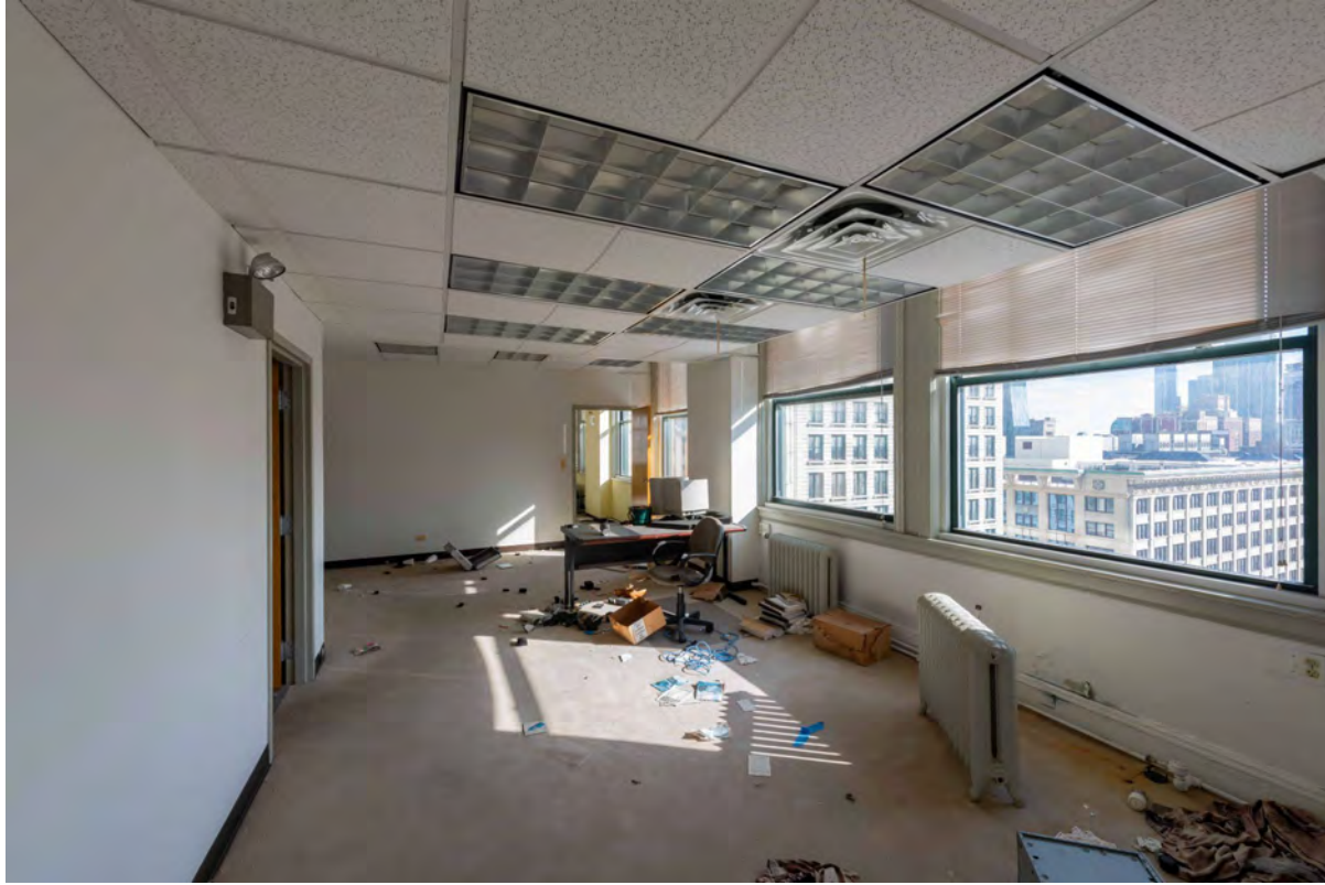
Level 16 Office Space
