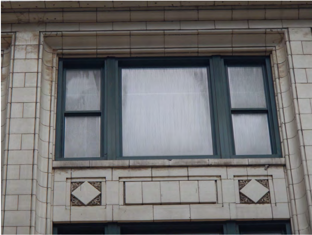
Overview of terra cotta spandrel and Chicago style window
