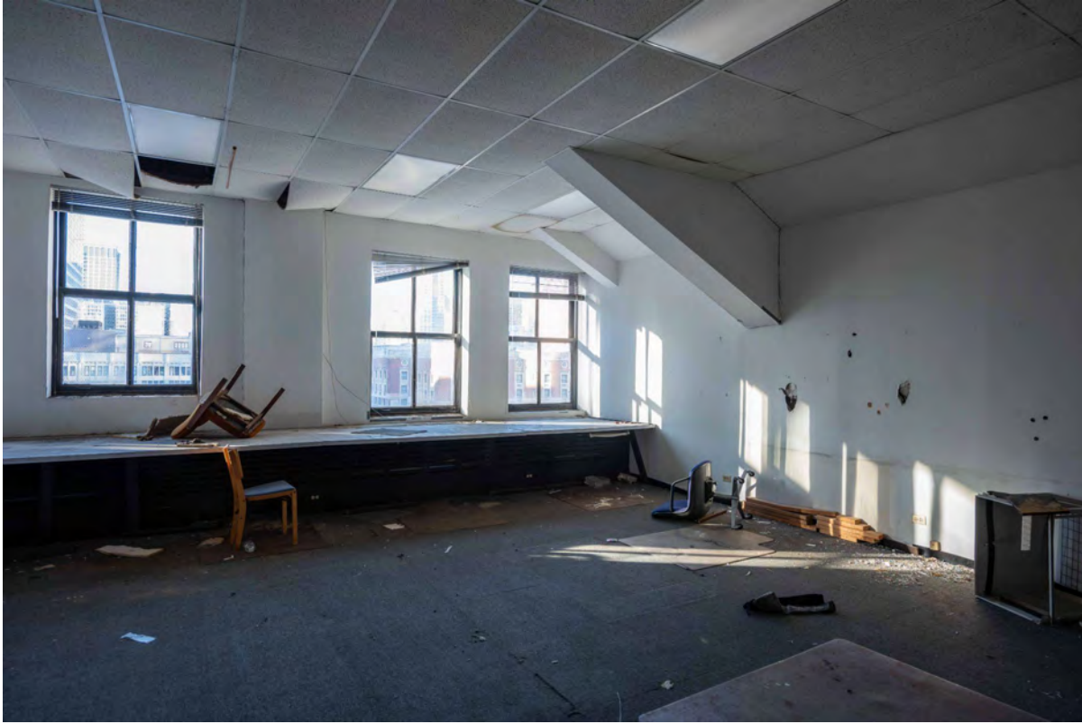
Level 22 Office space
