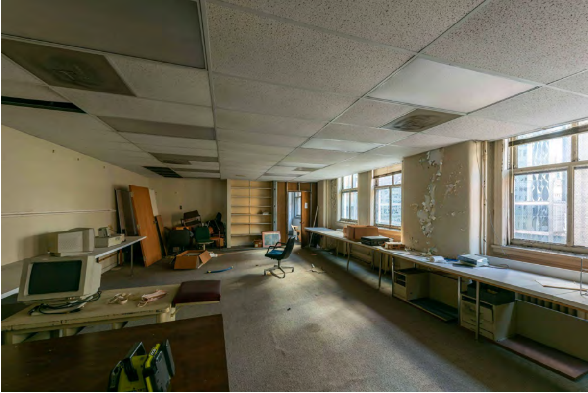
Level 15 Office Space
