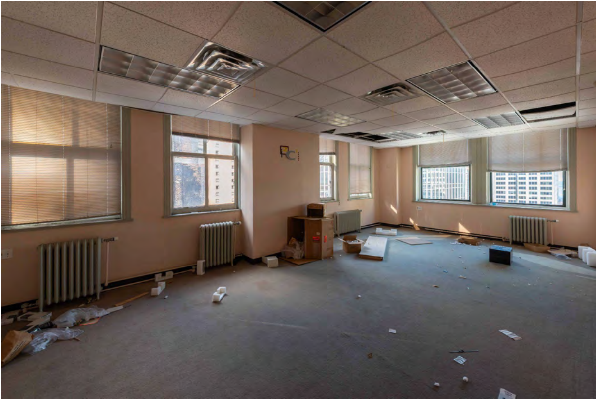
Level 16 Office Space
