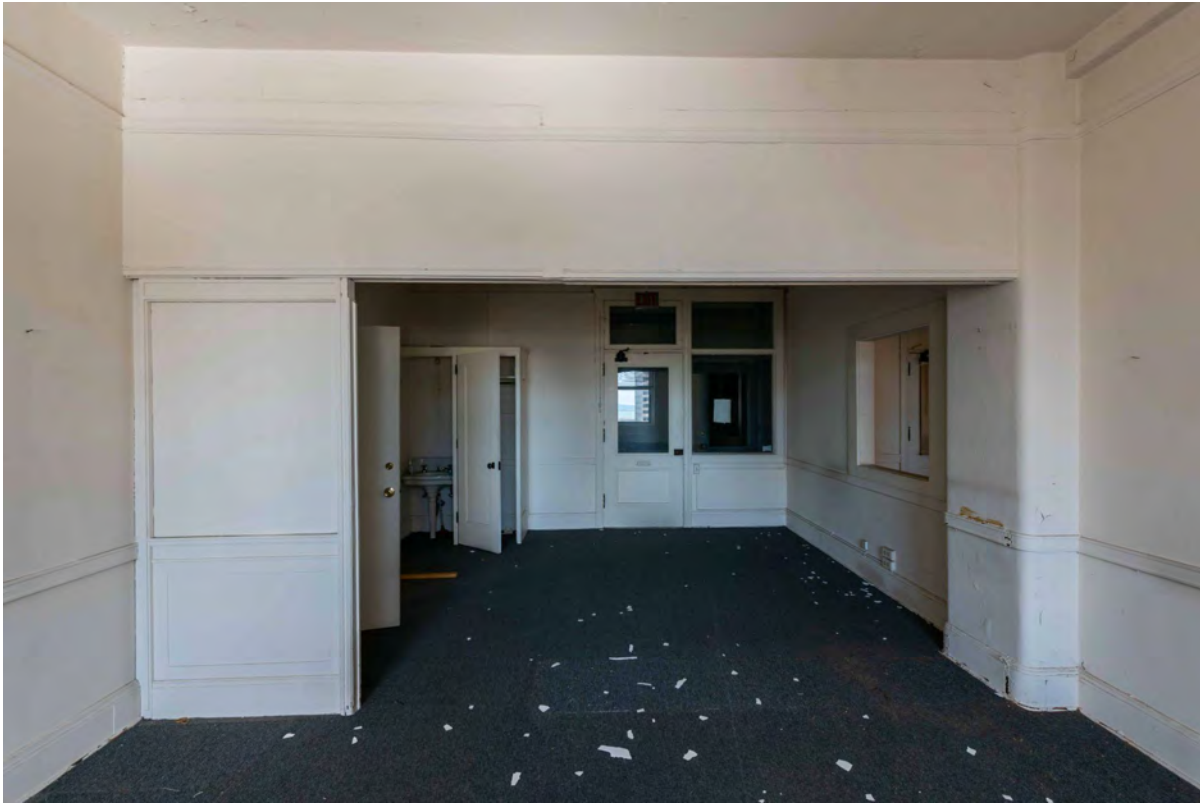
Level 13 Office Space
