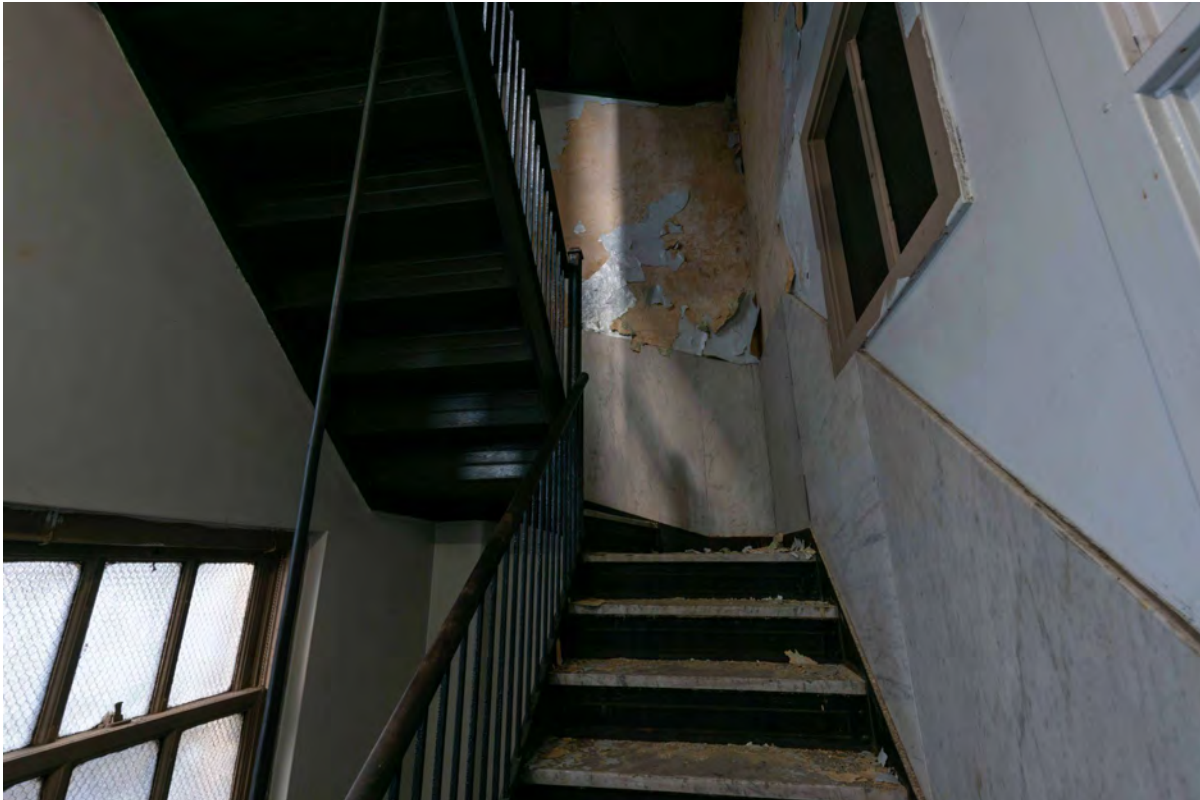
Level 15 going up to 16 West Stair
