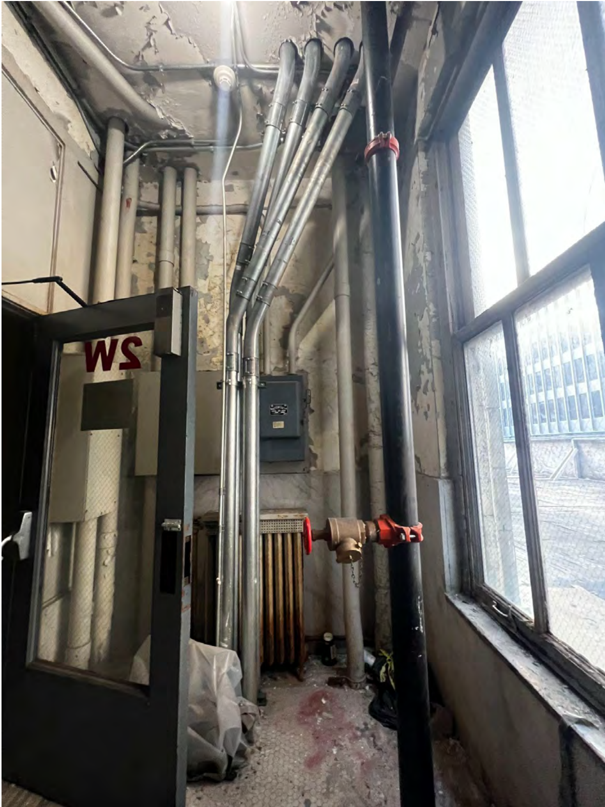
2nd Floor Stairwell: Existing riser to upper floors
