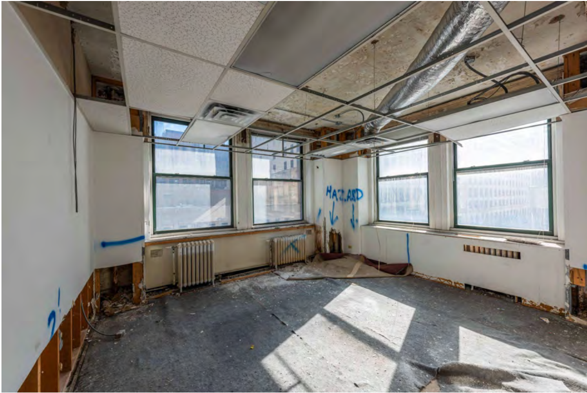
Level 5 Office Space
