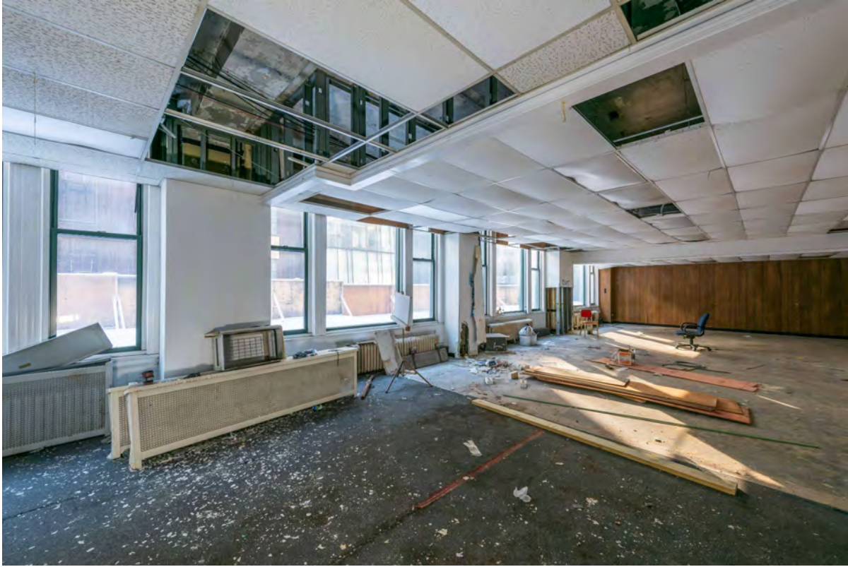
Level 2 Office Space
