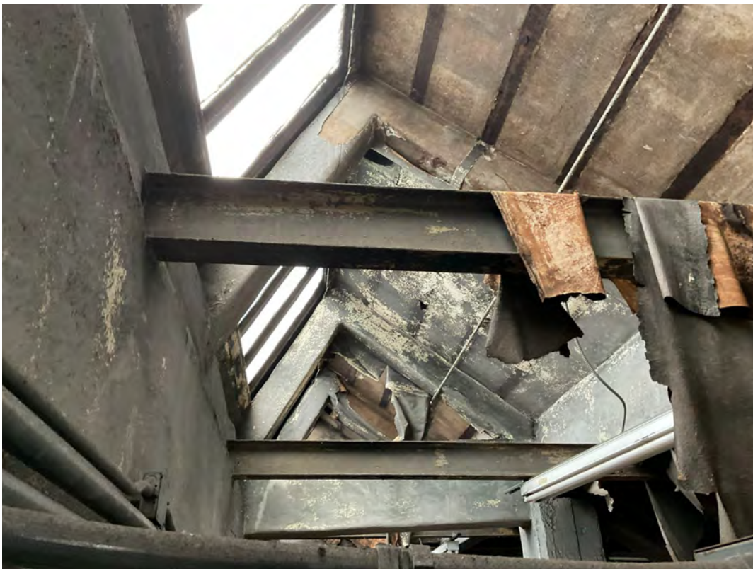
Roof structure: Structural support at glass skylight
