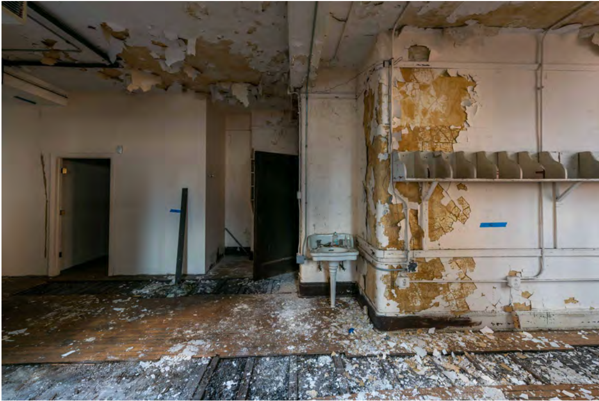
Level 4 Office Space
