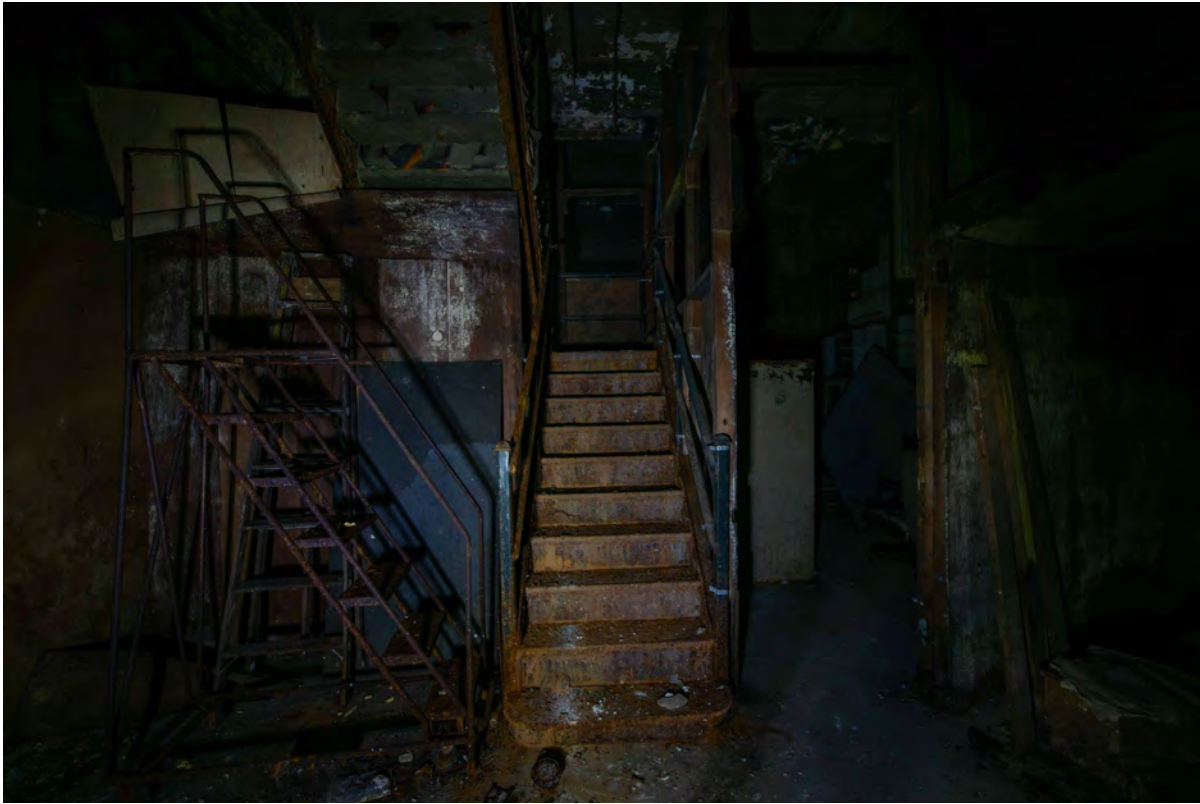
Lower Level 2 Stair
