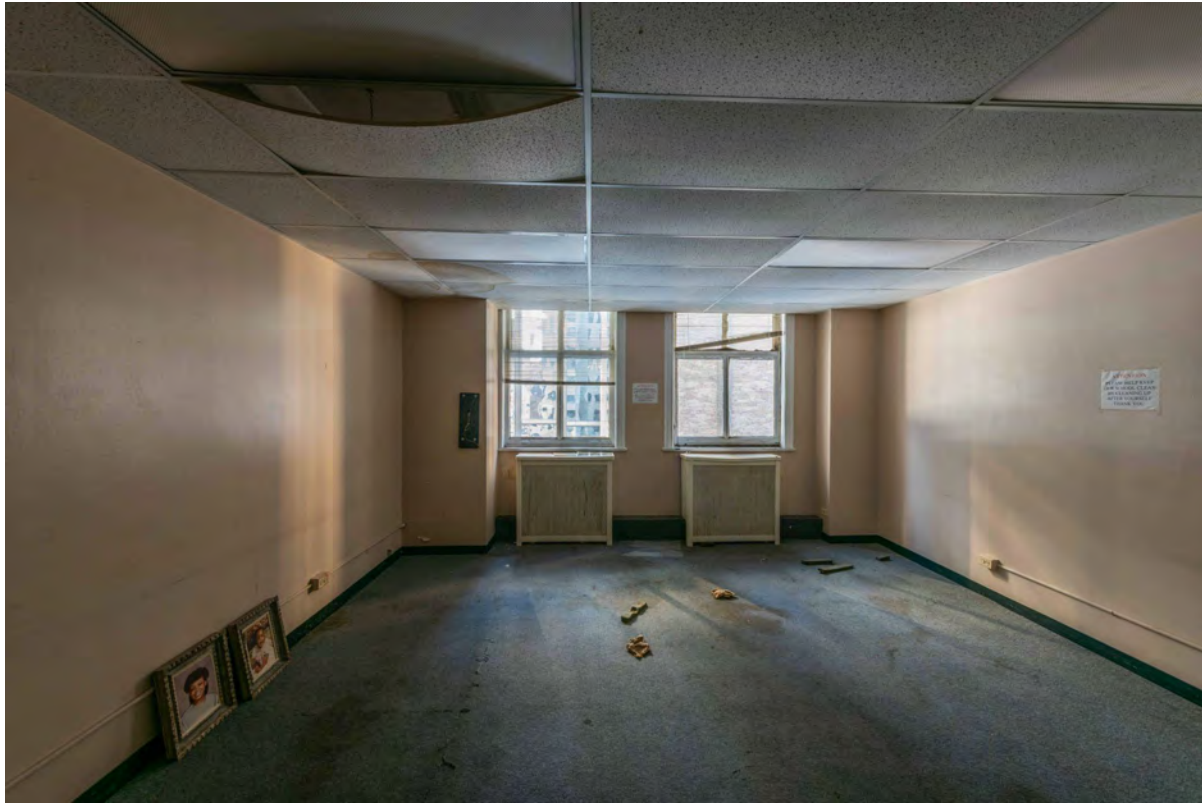
Level 7 Office Space
