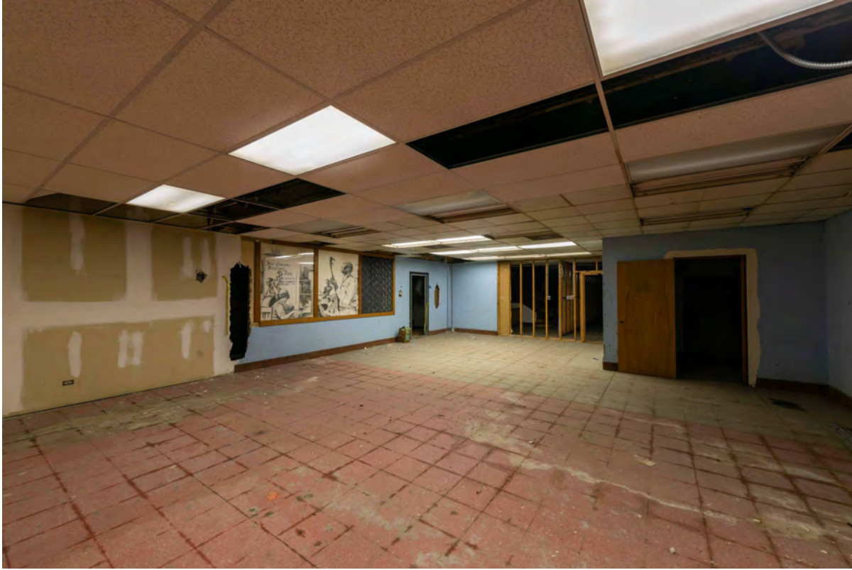
Lower Level 1 Former Restaurant Area
