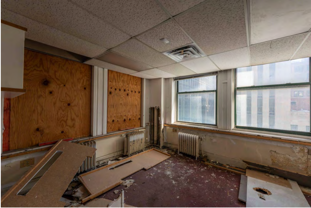
Level 5 Office Space
