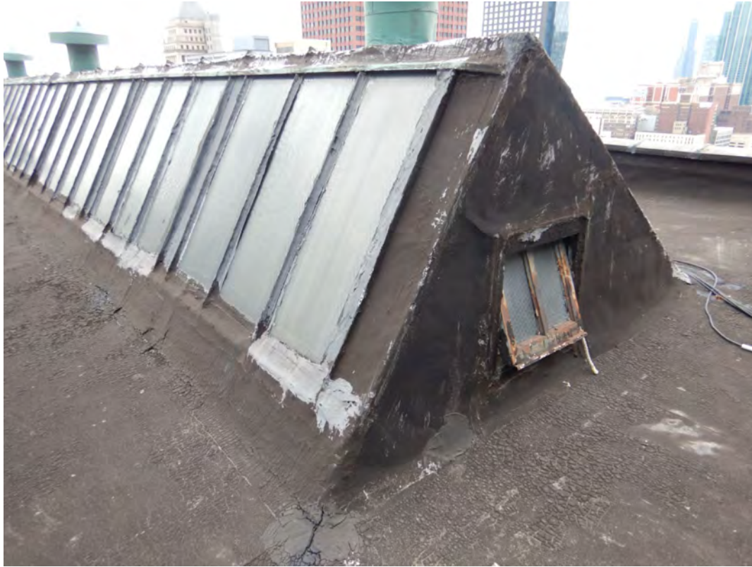
Skylight structure on upper roof, north elevation
