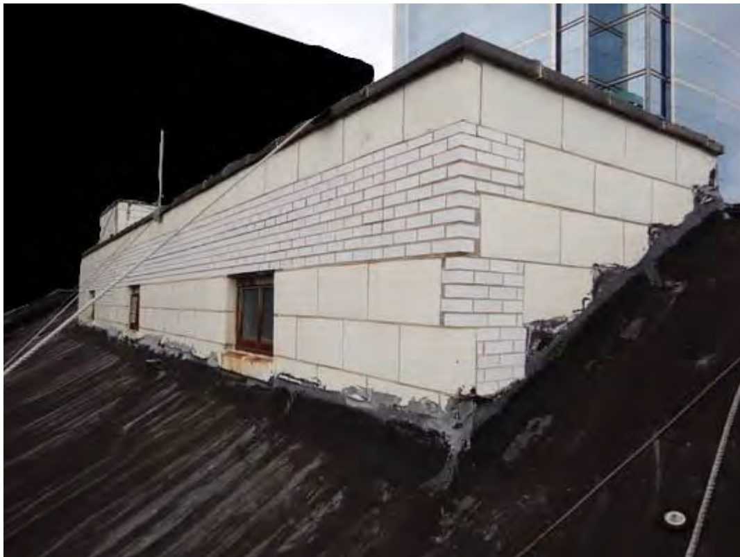
Temporarily repaired interior parapet structure
