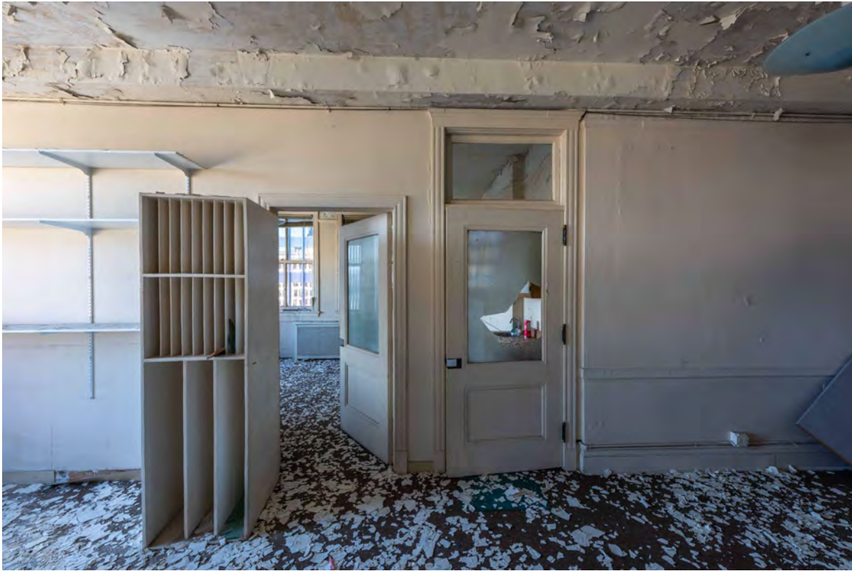
Level 19 Office Space
