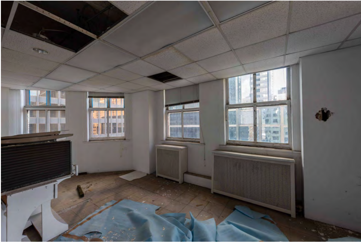
Level 14 Office Space
