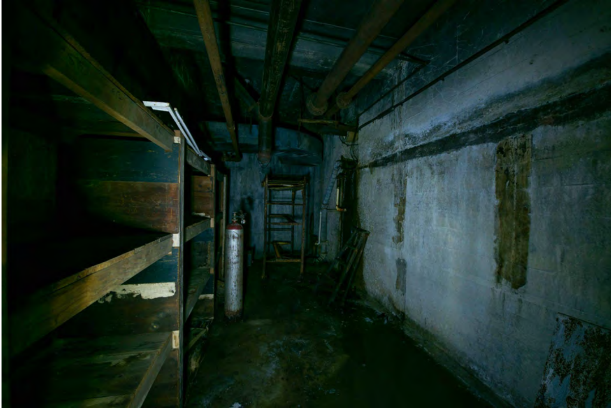
Lower Level 1 Storage Room
