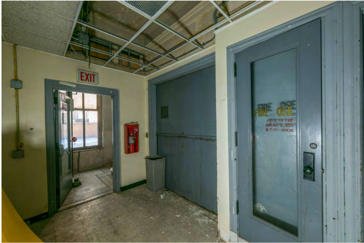
Level 2 Freight Hoistway and West Fire Stair
