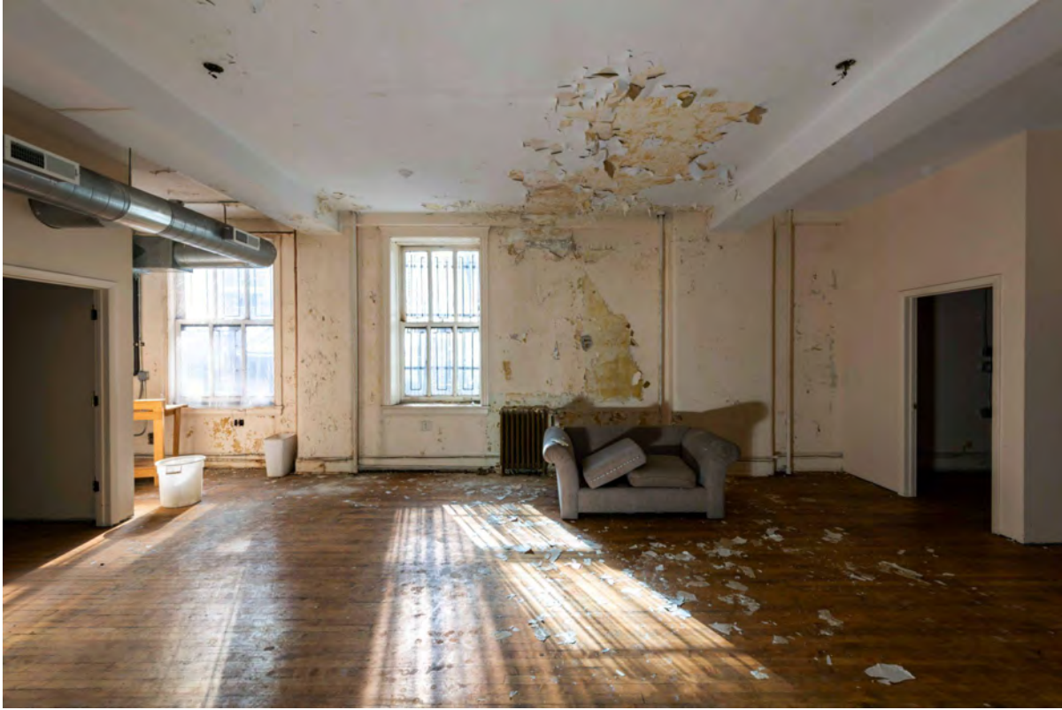
Level 4 Office space
