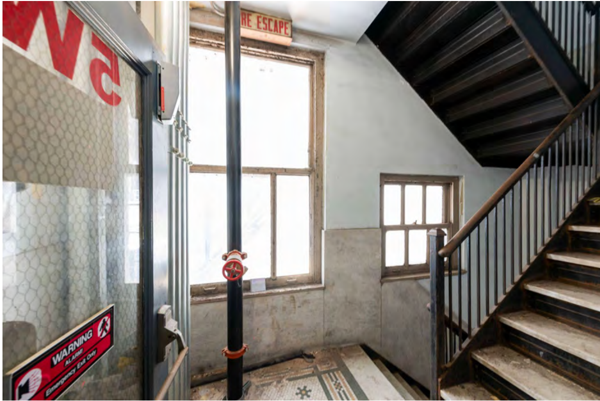
Level 5 West Fire Stair
