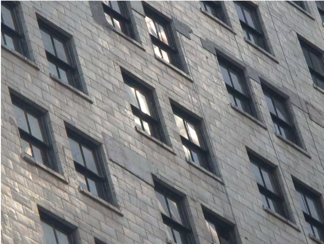
Overview of north elevation with previous stabilization efforts
