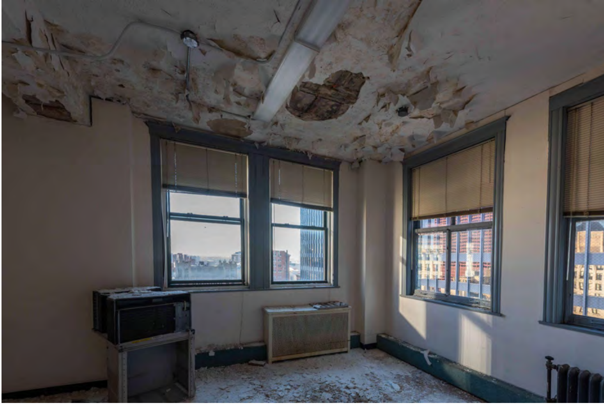
Level 21 Office space
