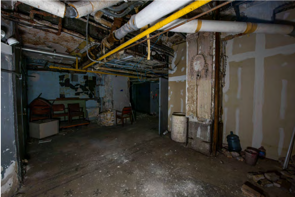
Lower Level 1 Plaster Detail Remanent
