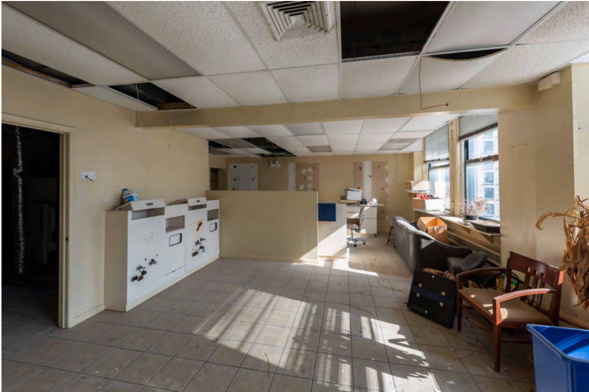
Level 12 Office Space
