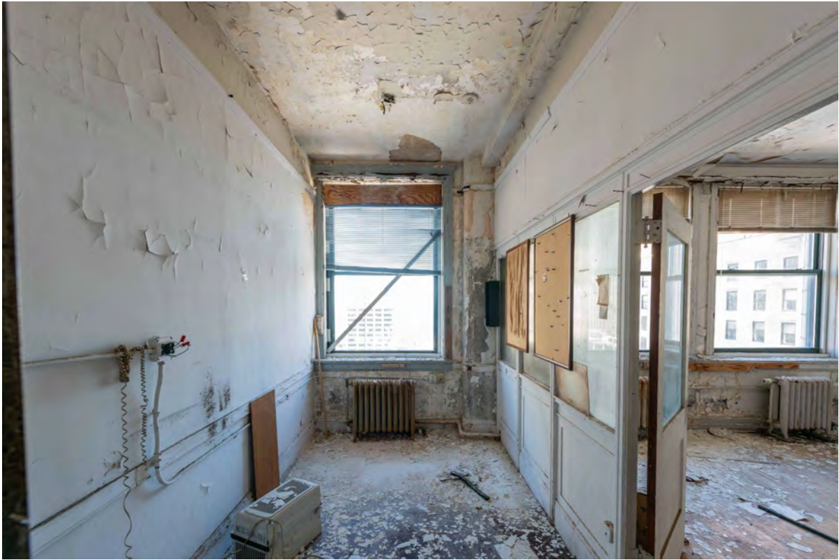
Level 20 Office Space
