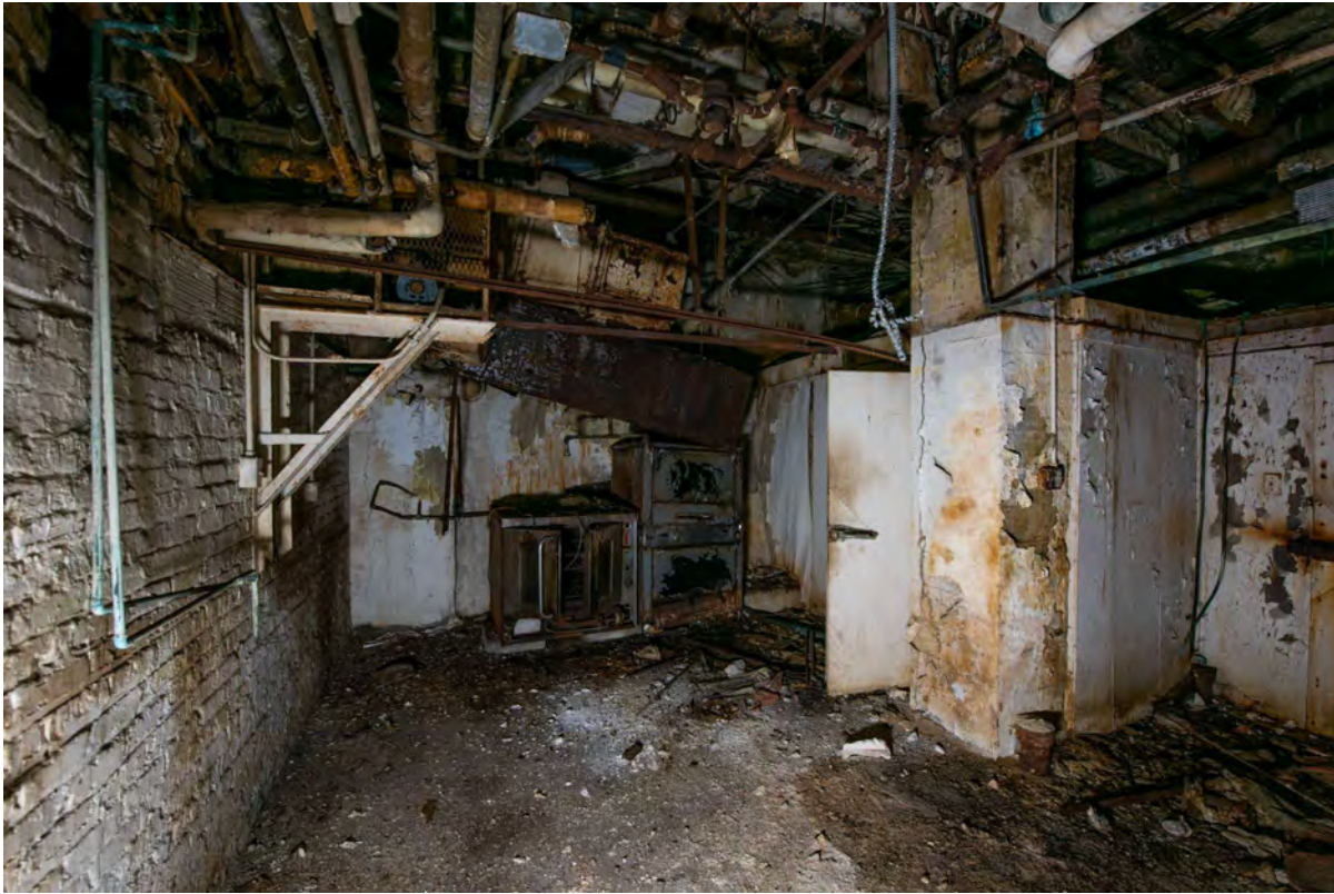
Lower Level 1 Former Restaurant Kitchen
