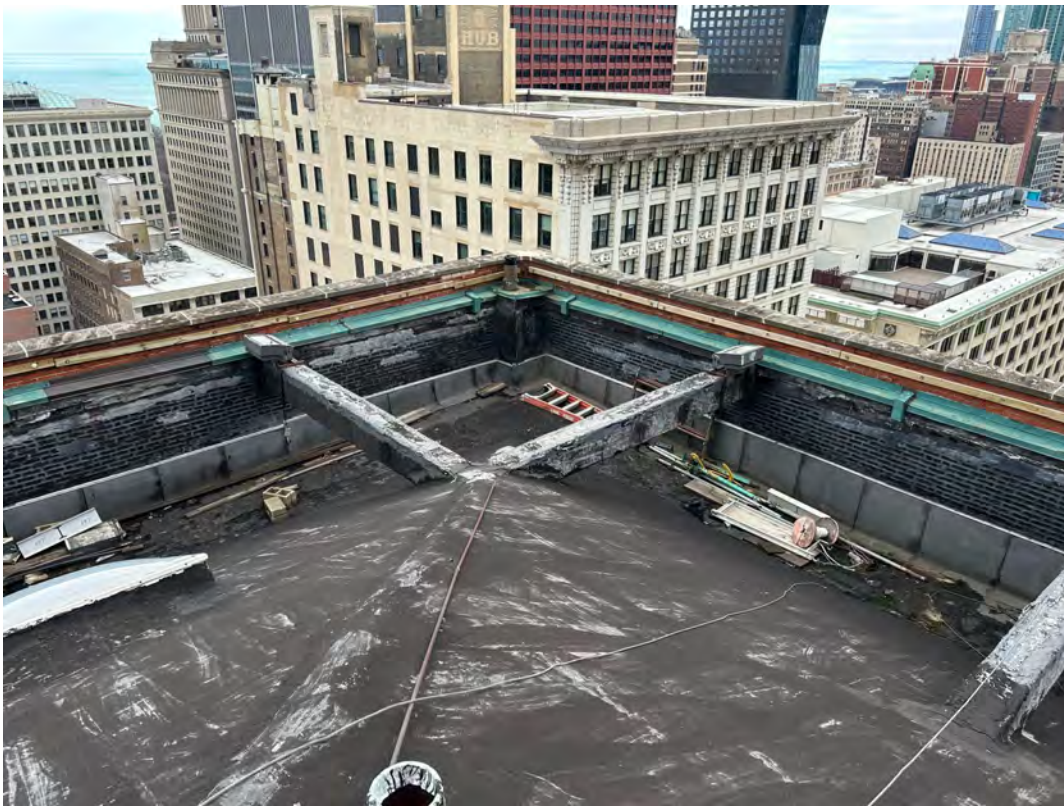
Southeast roof corner
