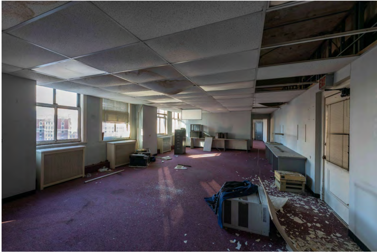
Level 21 Office Space
