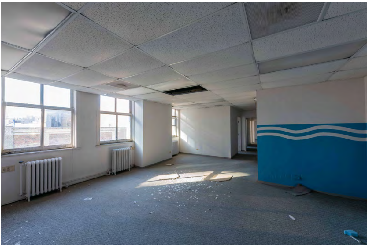
Level 19 Office space
