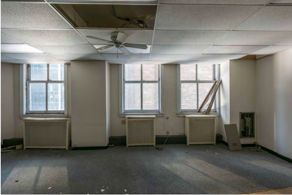
Level 8 Office Space
