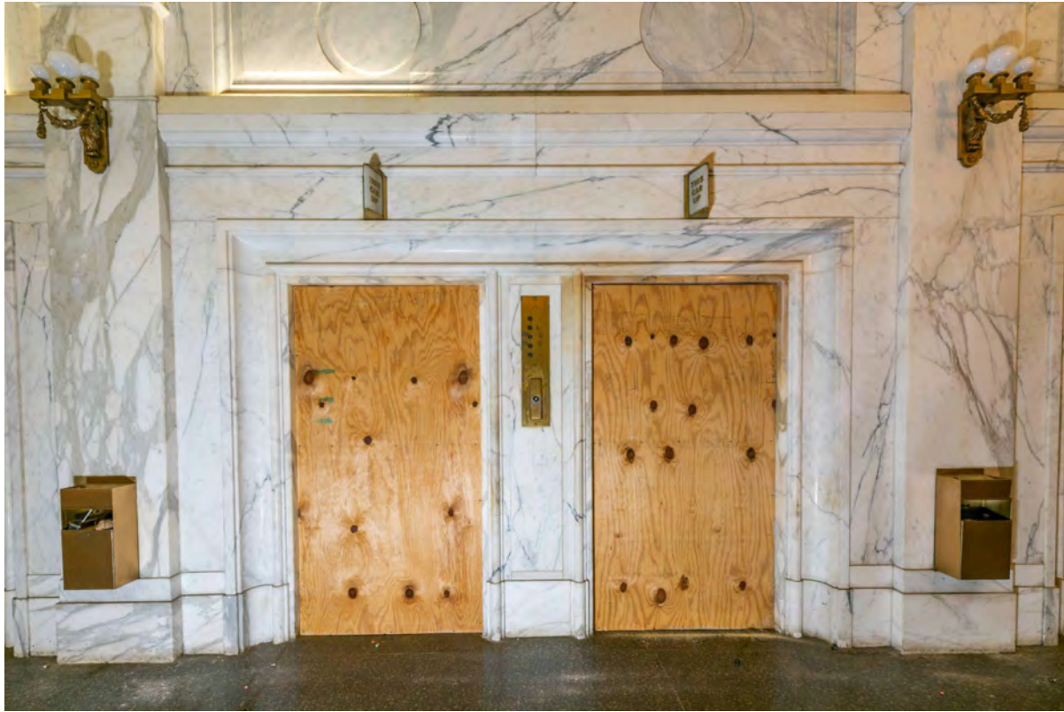
1st Floor Main Lobby Hoistway Openings
