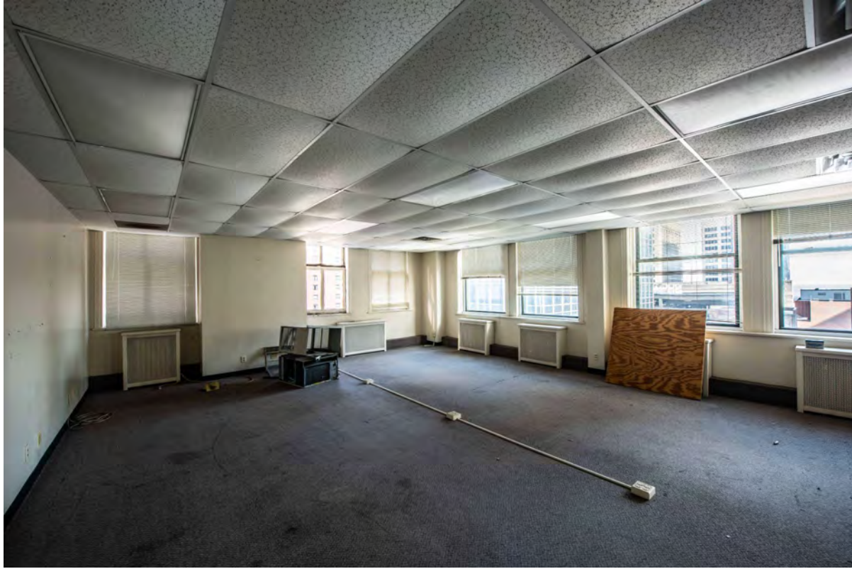
Level 11 Office Space
