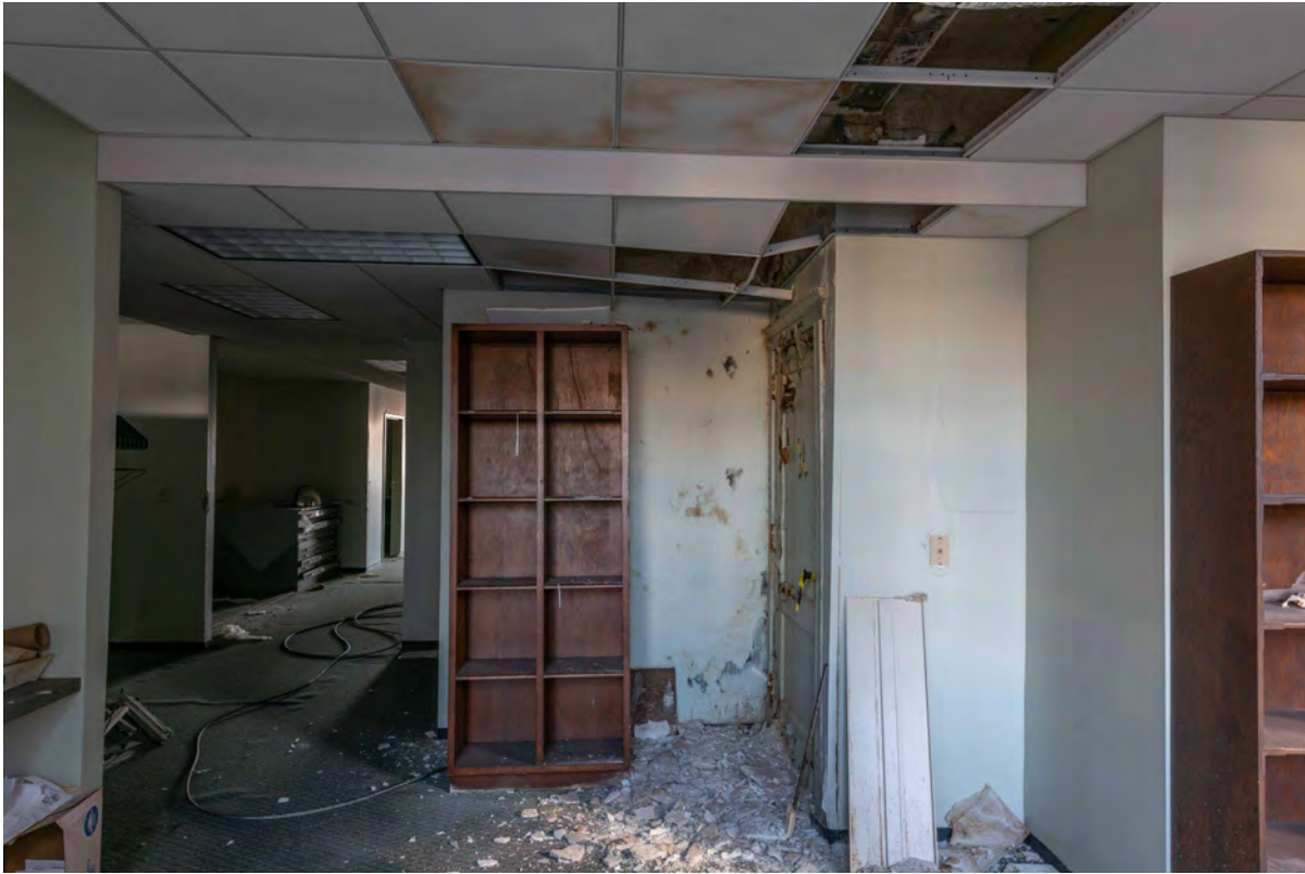
Level 18 Office Space
