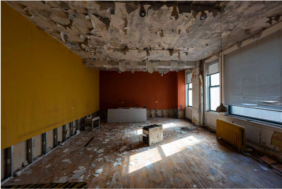
Level 4 Office Space
