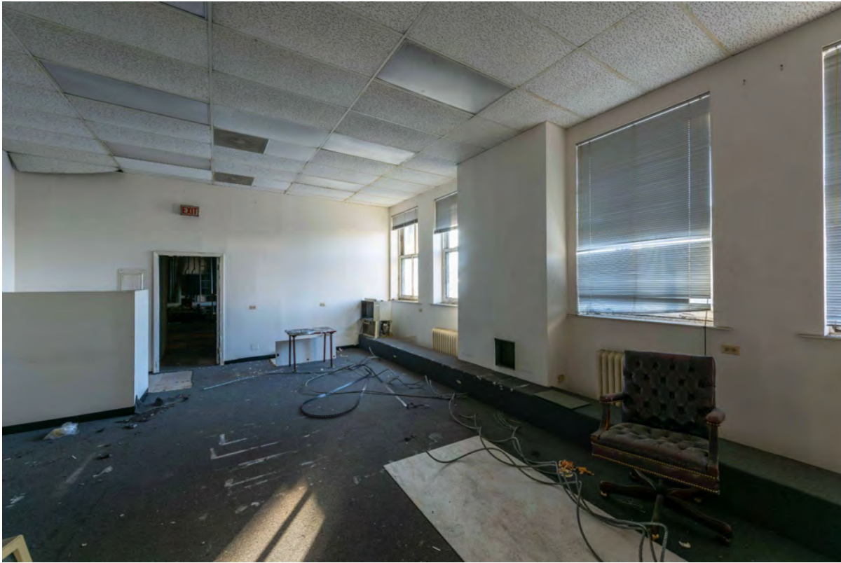
Level 22 Office Space
