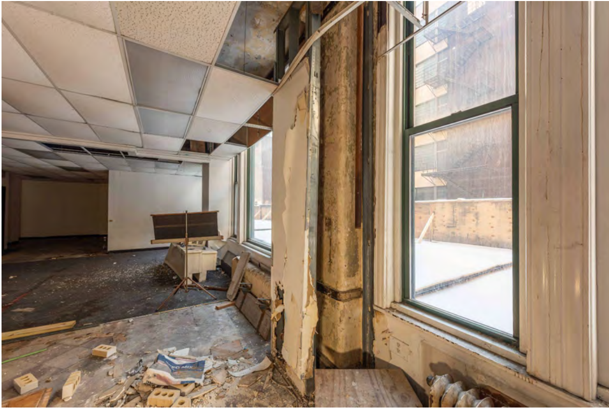
Level 2 Office Space
