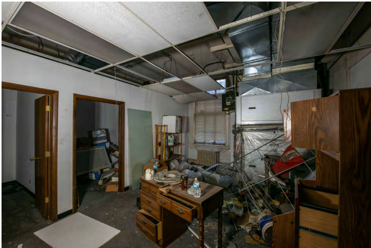
Level 3 Office Space
