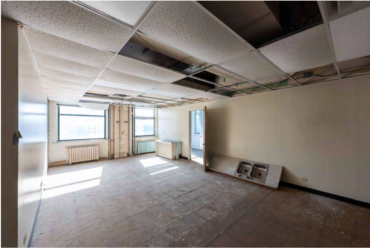
Level 11 Office Space
