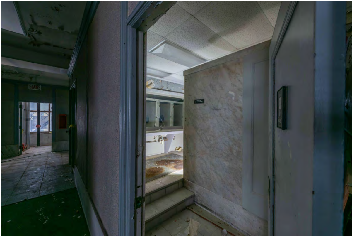
Level 6 Restroom. Note 2 Steps Up.
