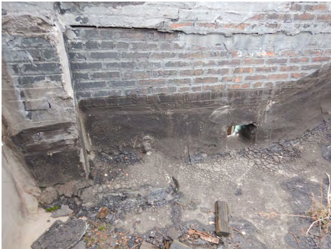
Through wall scupper at southeast roof corner in west elevation
