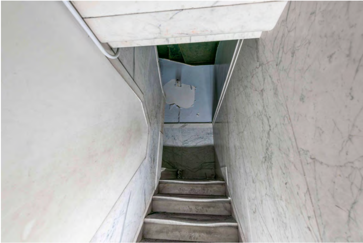
Stair from Level 1 Up to Level 2
