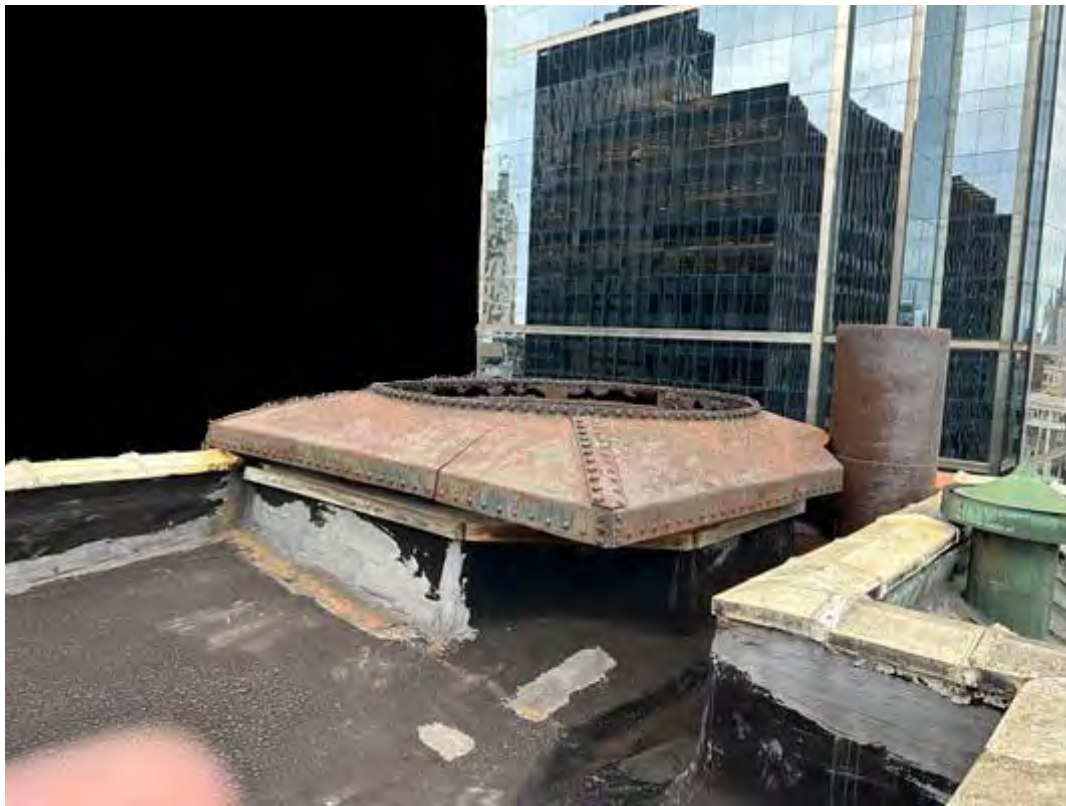
Penthouse roof with terra cotta coping
