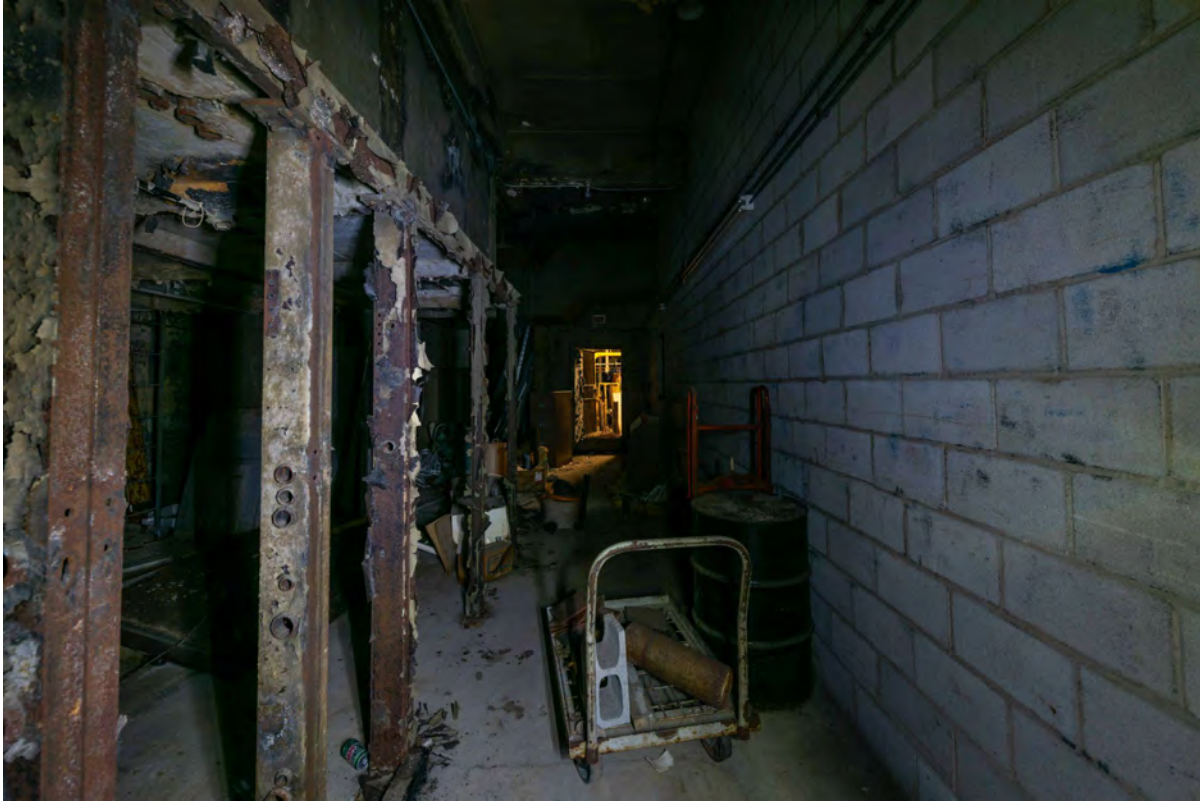
Lower Level 2 Corridor
