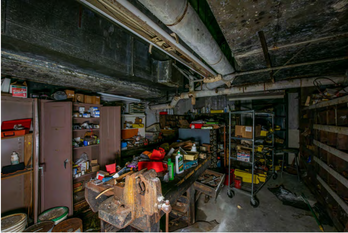
Lower Level 1 Typical Maintenance storage Space
