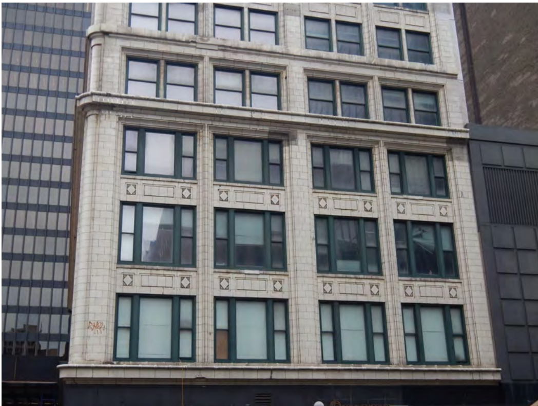
Overview of belt course and water tables at lower floors
