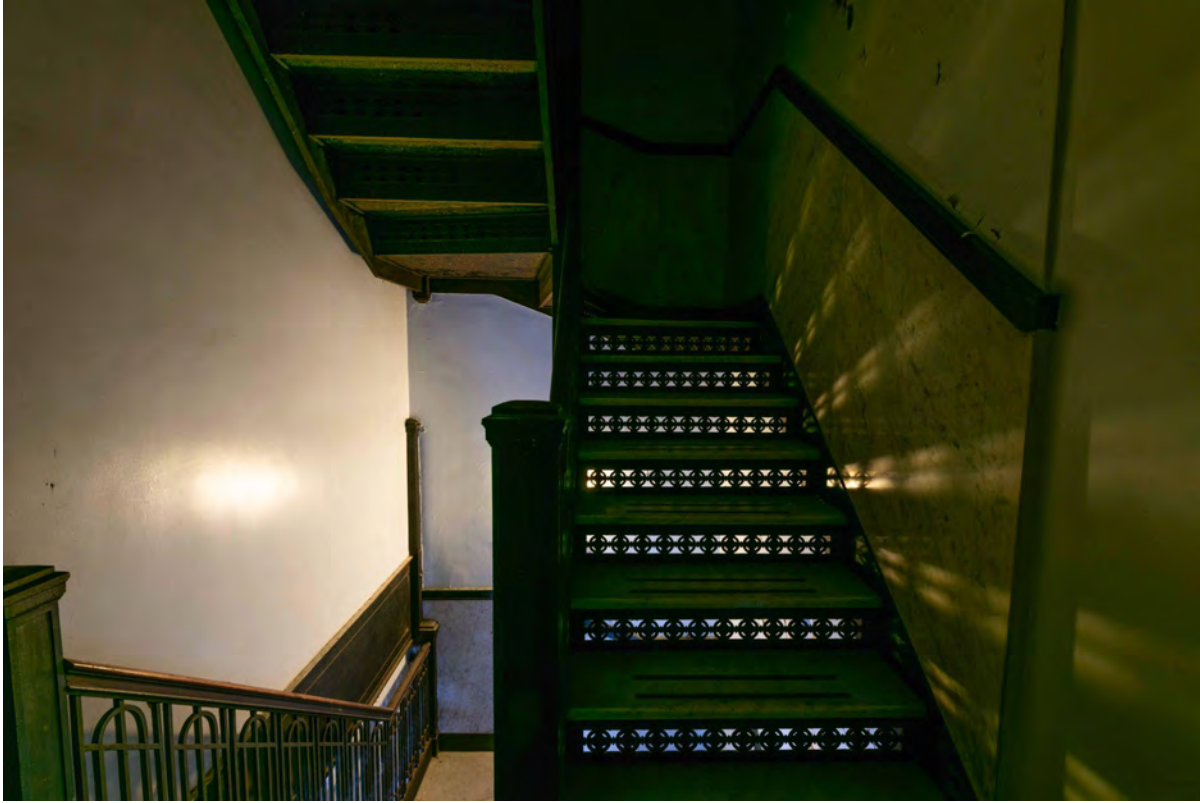
Level 7 East Stair
