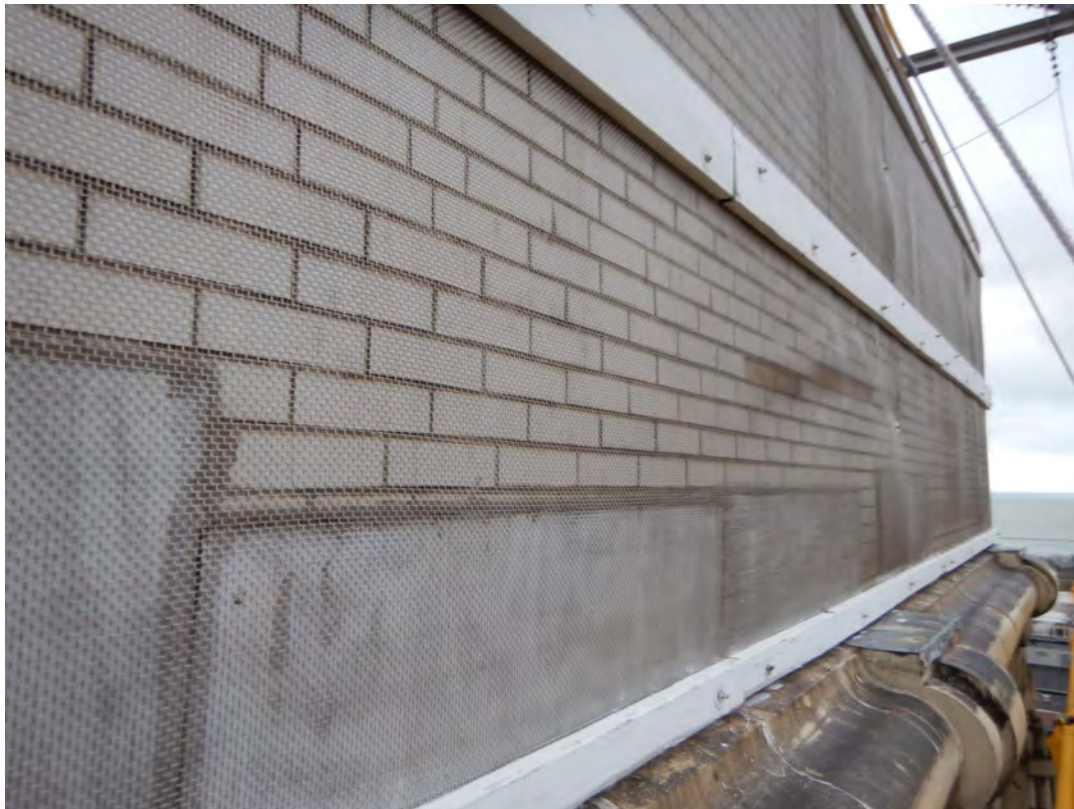
Overview of parapet wall with wood 2x and steel mesh
