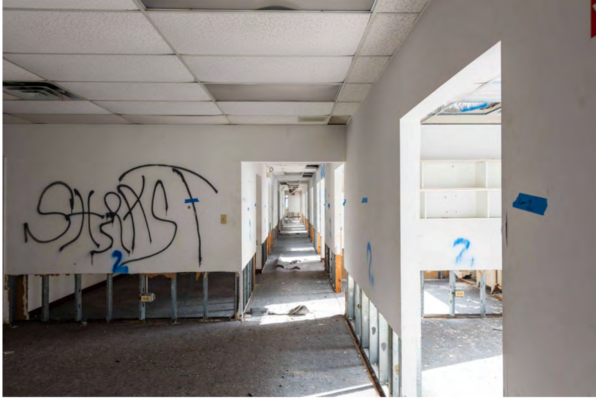
Level 5 Office Space
