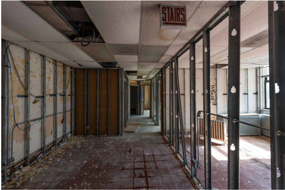
Level 8 Office Space
