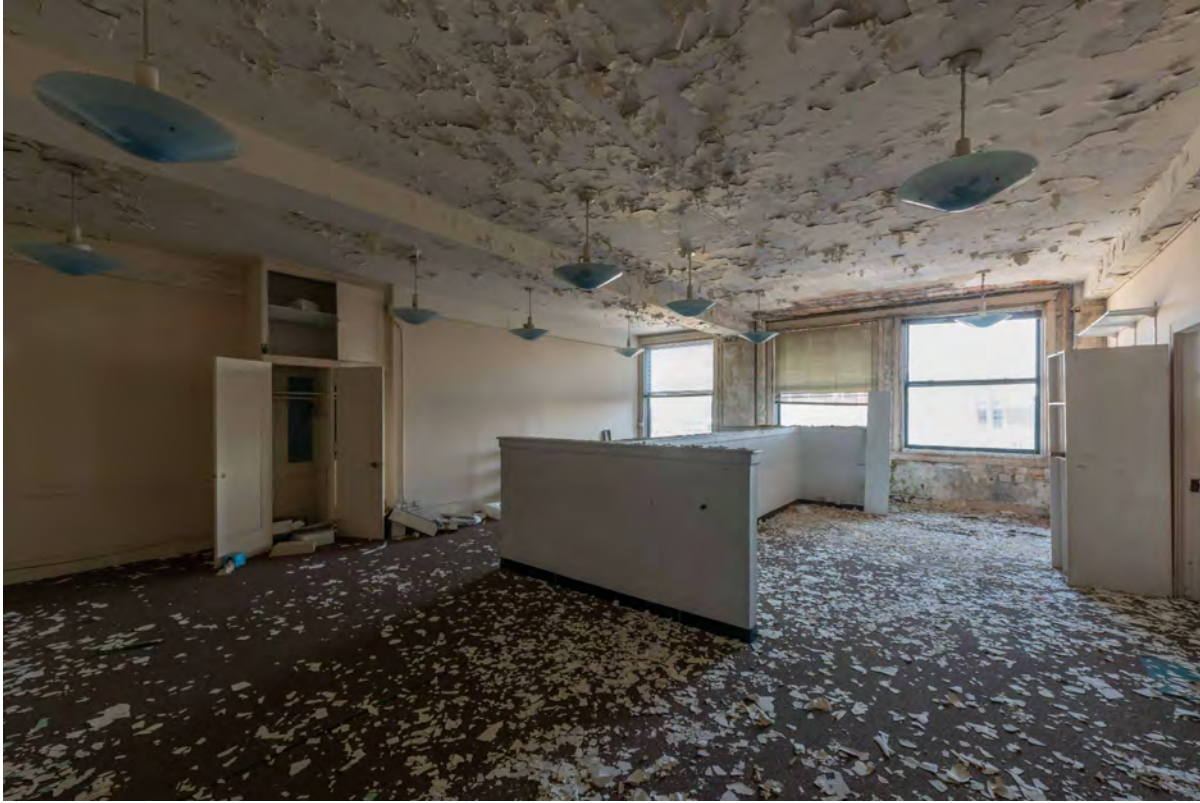
Level 19 Office Space
