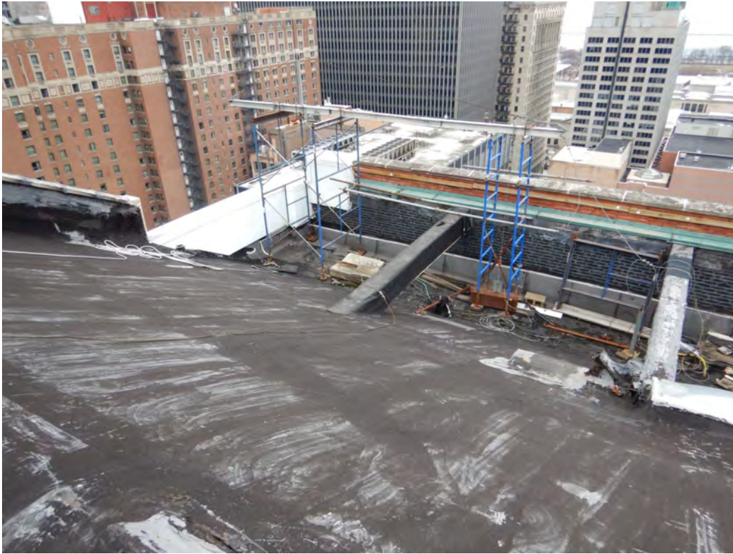
Northeast roof corner, parapet with white sheet metal enclosure
