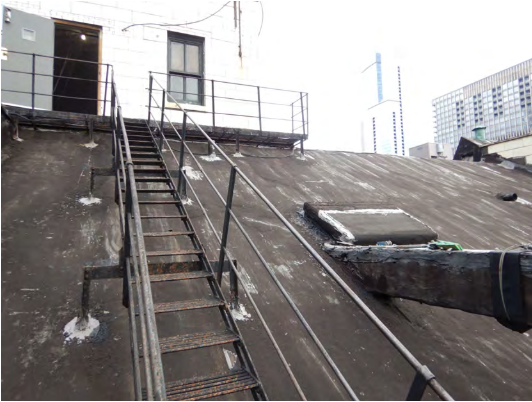
Steel stair structure to lower roof
