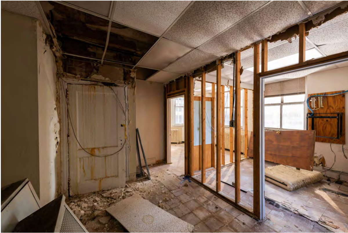
Level 8 Office Space
