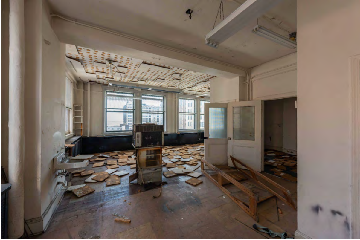
Level 13 Office Space
