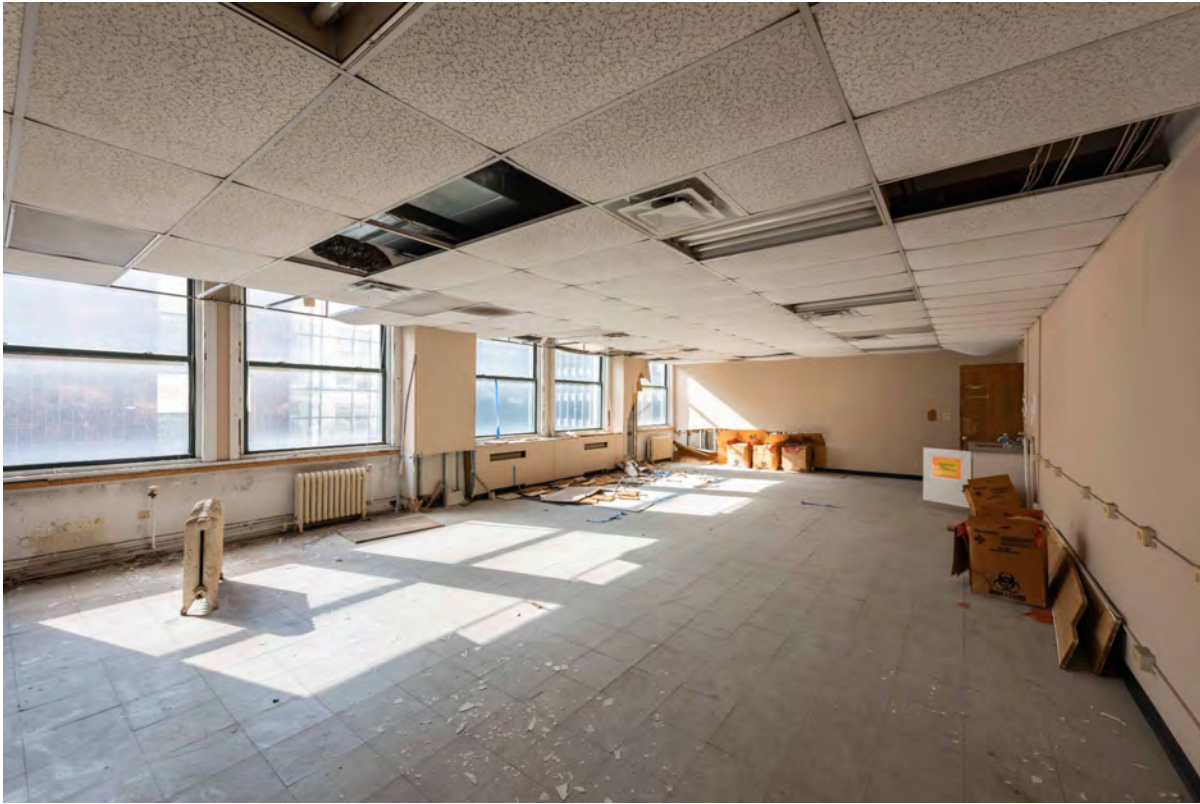
Level 6 office Space
