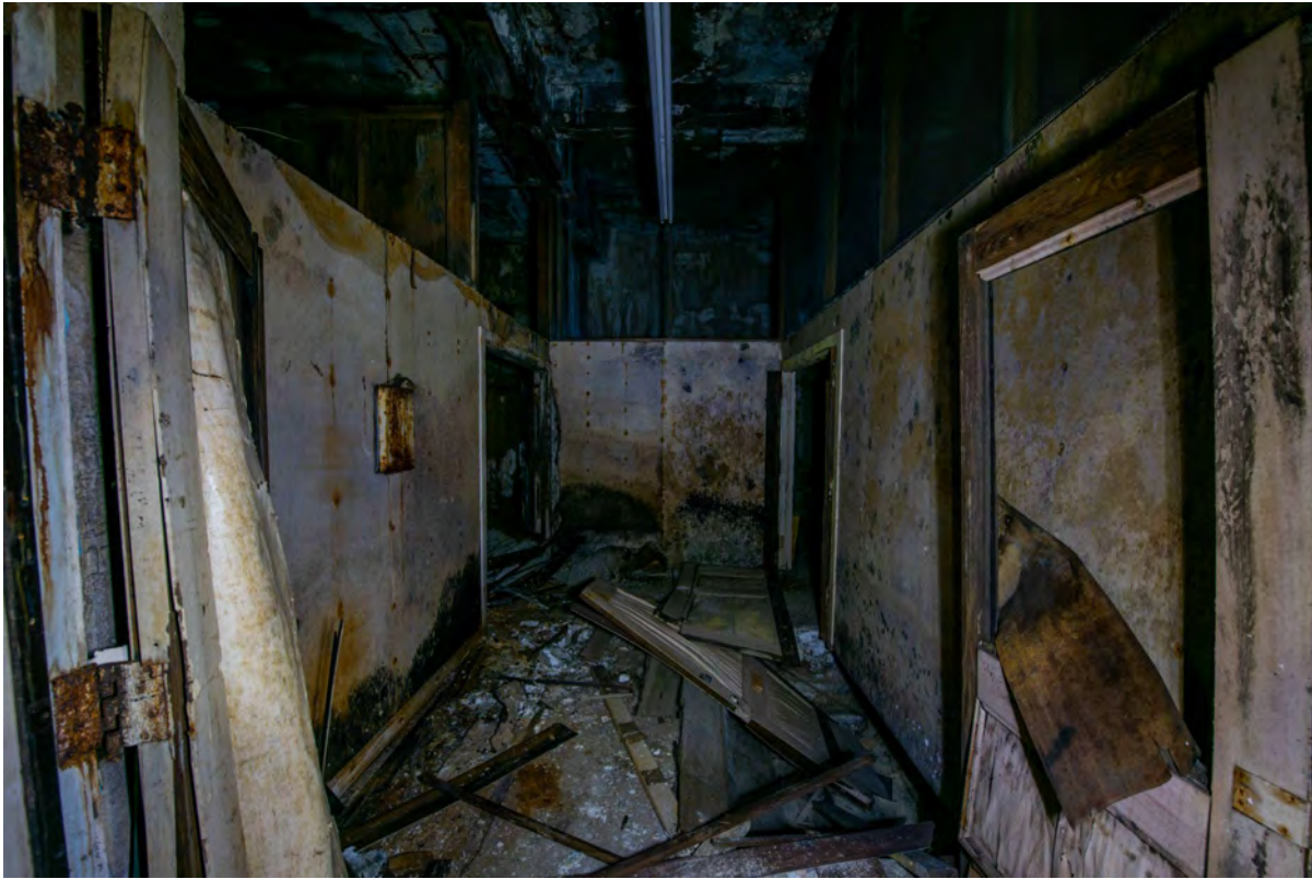
Lower Level 2 Corridor
