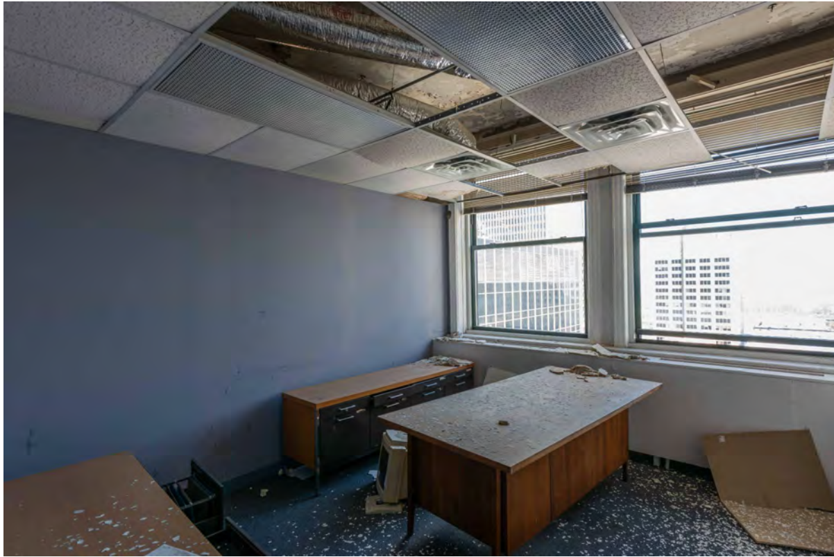
Level 16 Office space
