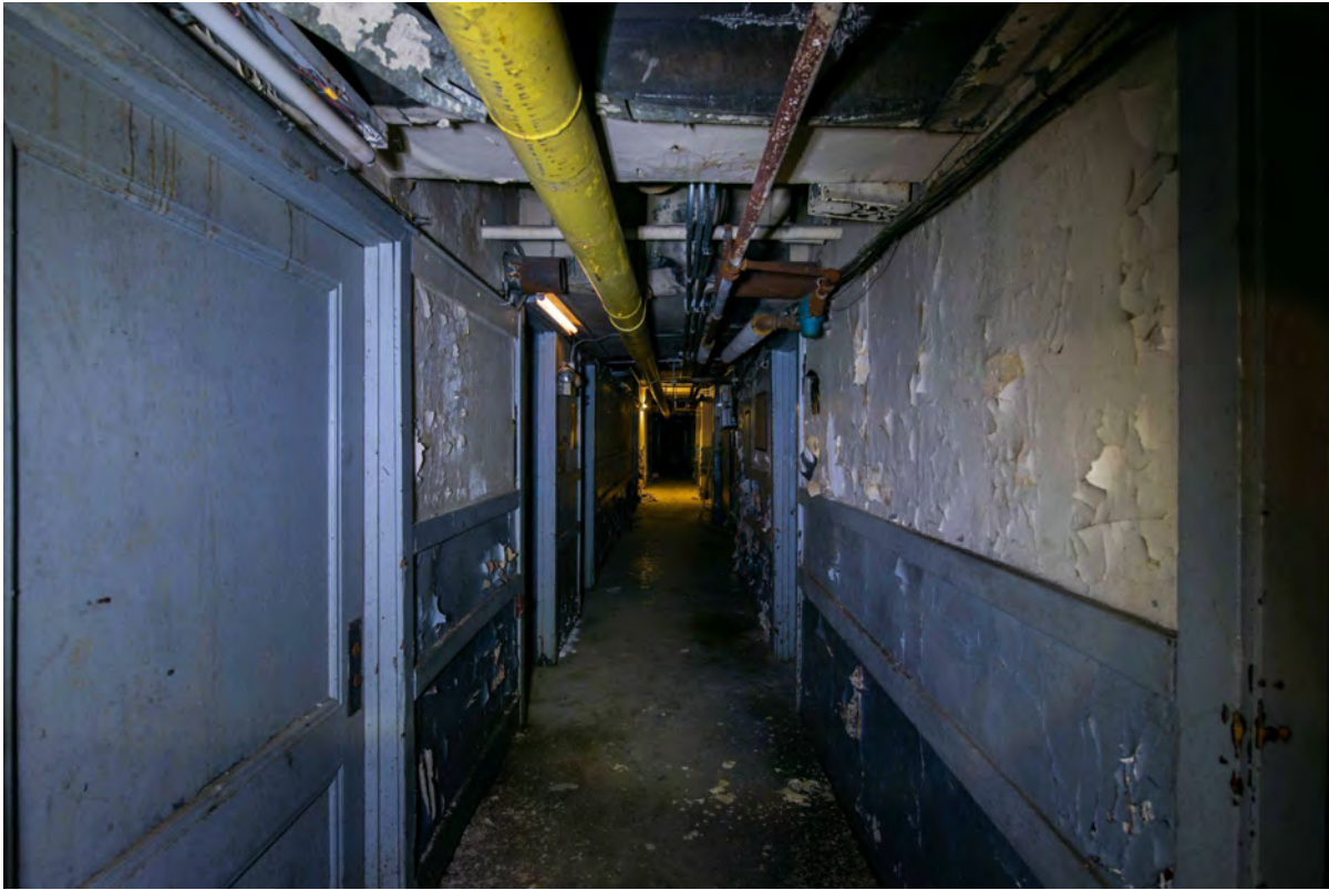
Lower Level 1 Typical Corridor
