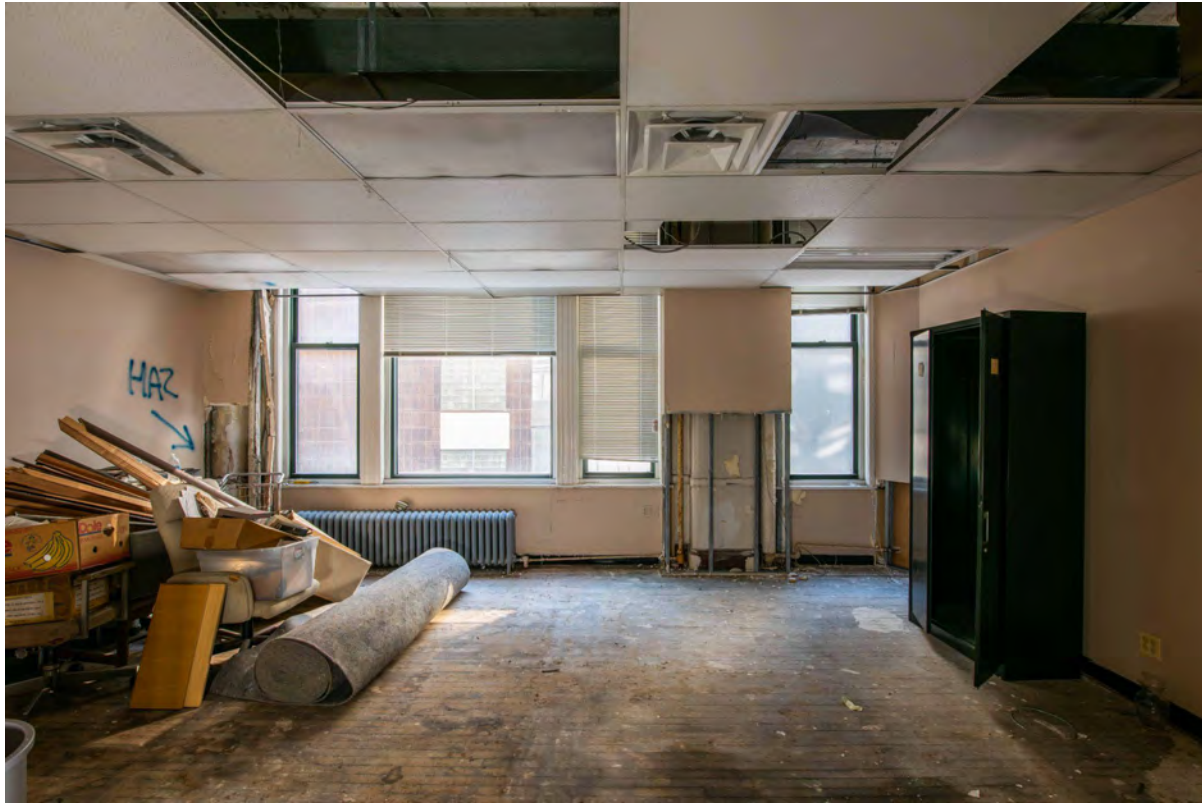
Level 3 Office Space
