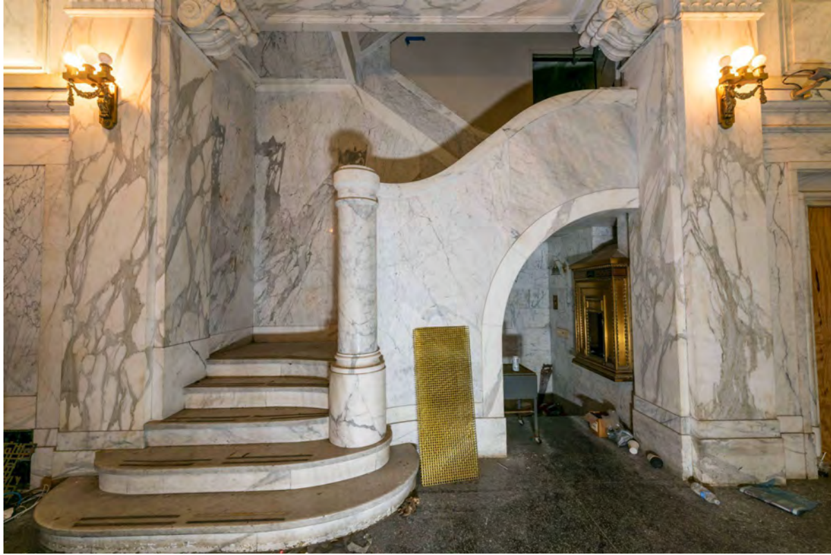
1st Floor Main Lobby Stairs Up and Down
