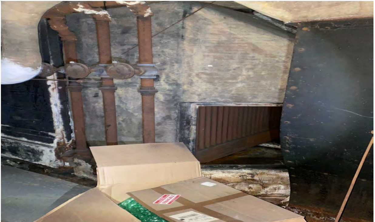
Basement 2 - Existing AHU
