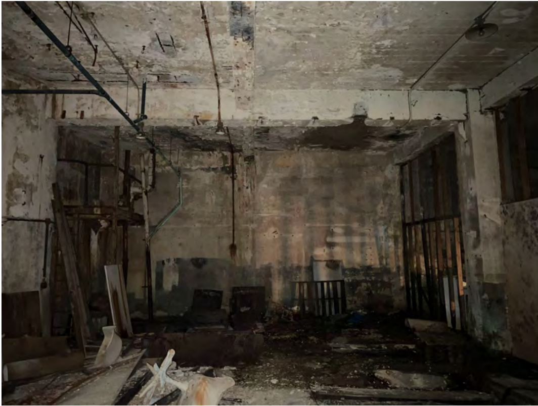
Middle basement slab from below: Slab and encased framing
