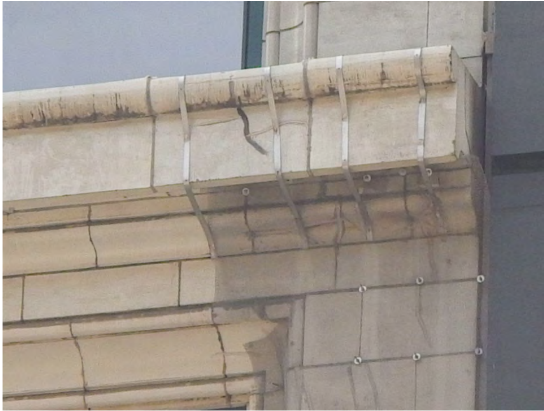
Overview of steel straps and mesh installed at water table
