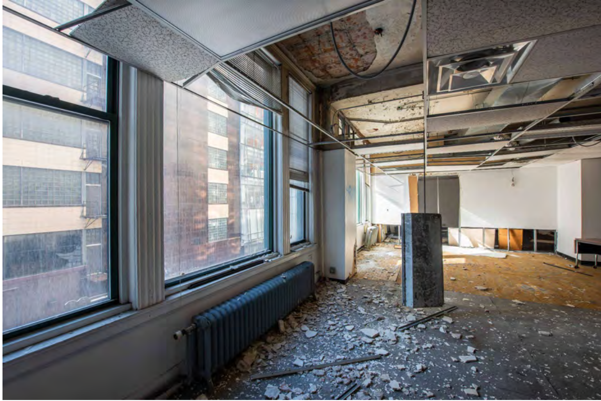
Level 3 Office Space
