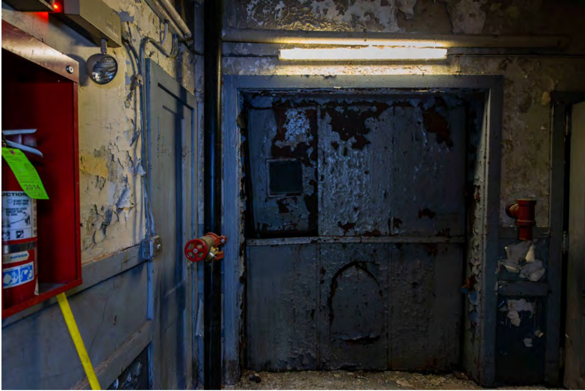
Lower Level 1 Freight Elevator Hoistway Opening
