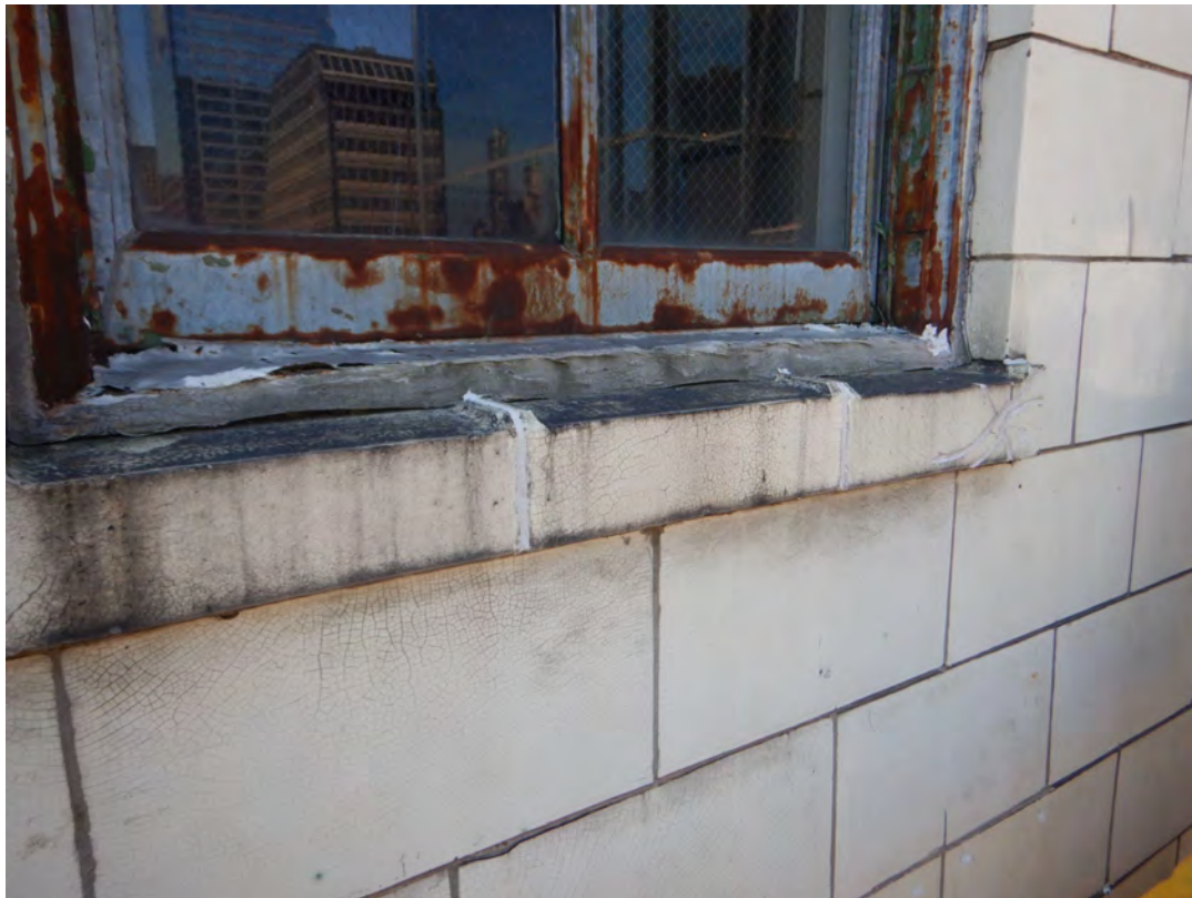
Overview of typical steel window sill
