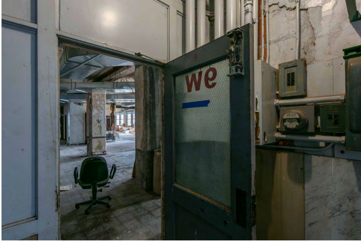
Level 9 West Stair
