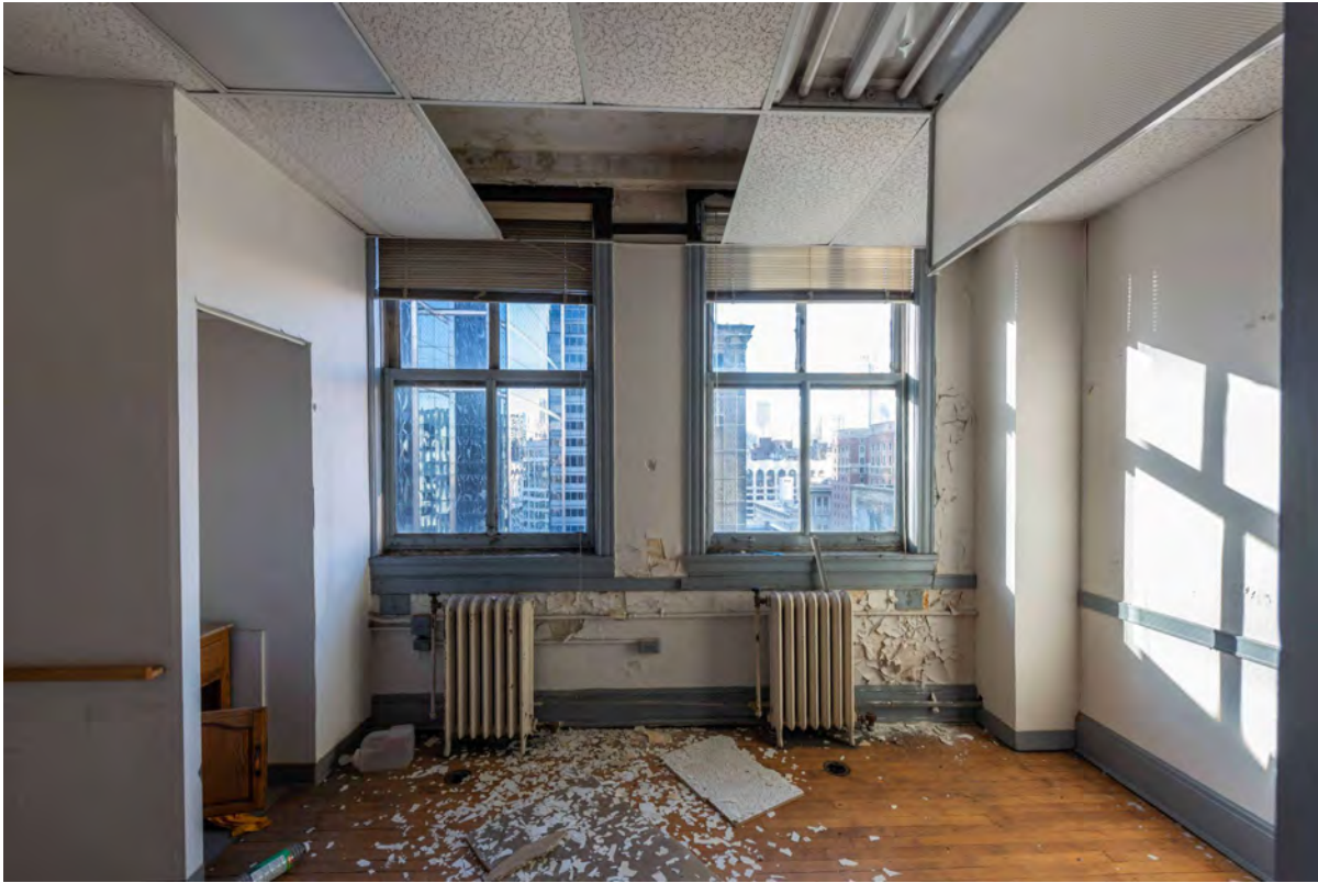
Level 20 Office Space
