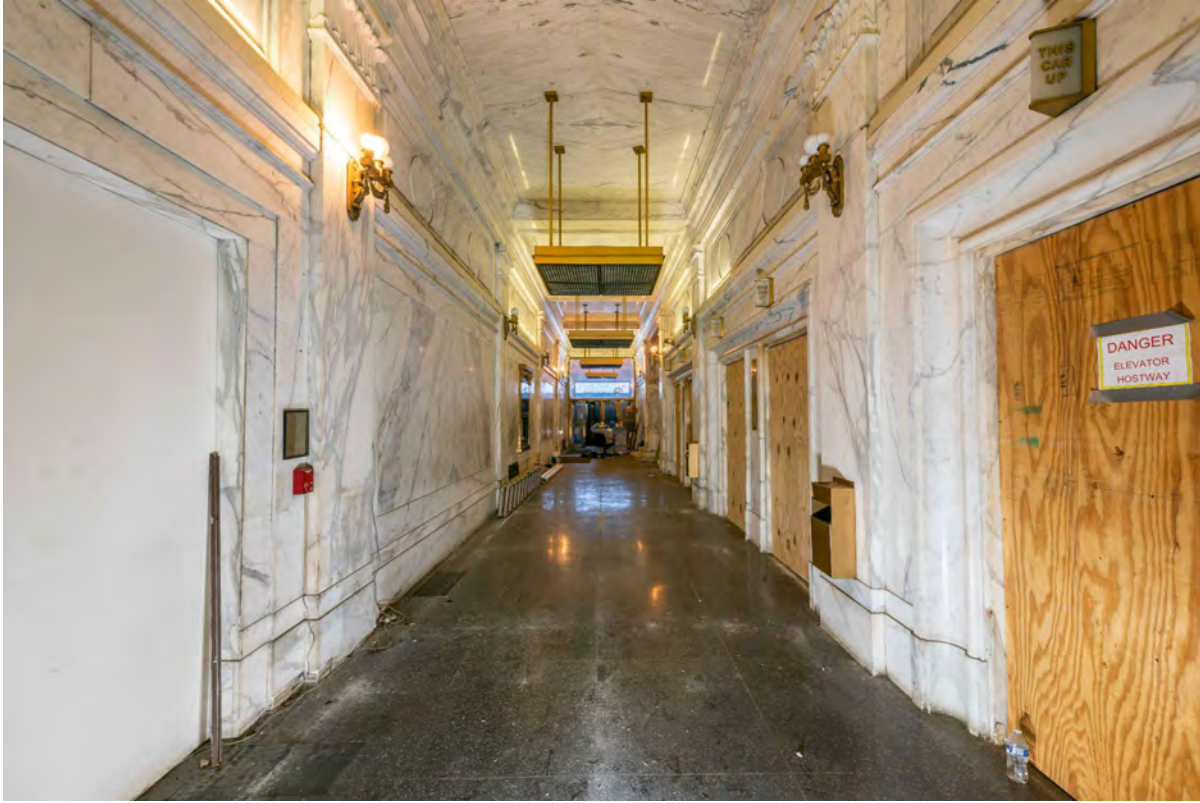
1st Floor Main Lobby Looking East
