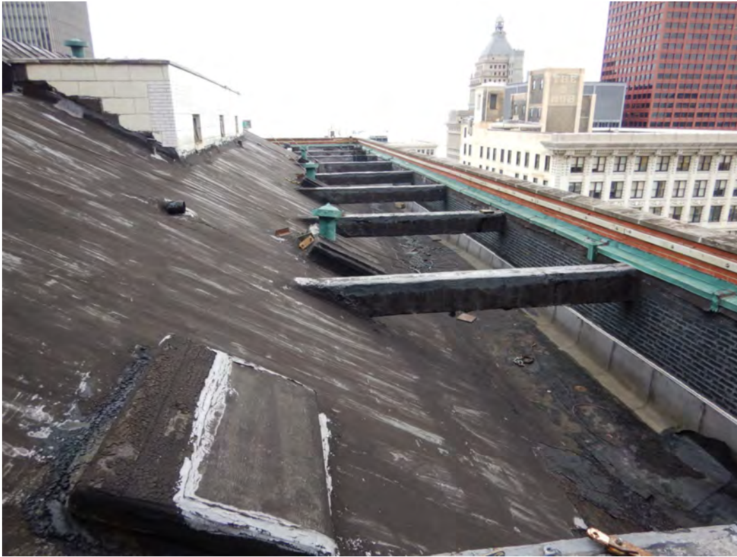
Looking east along south parapet
