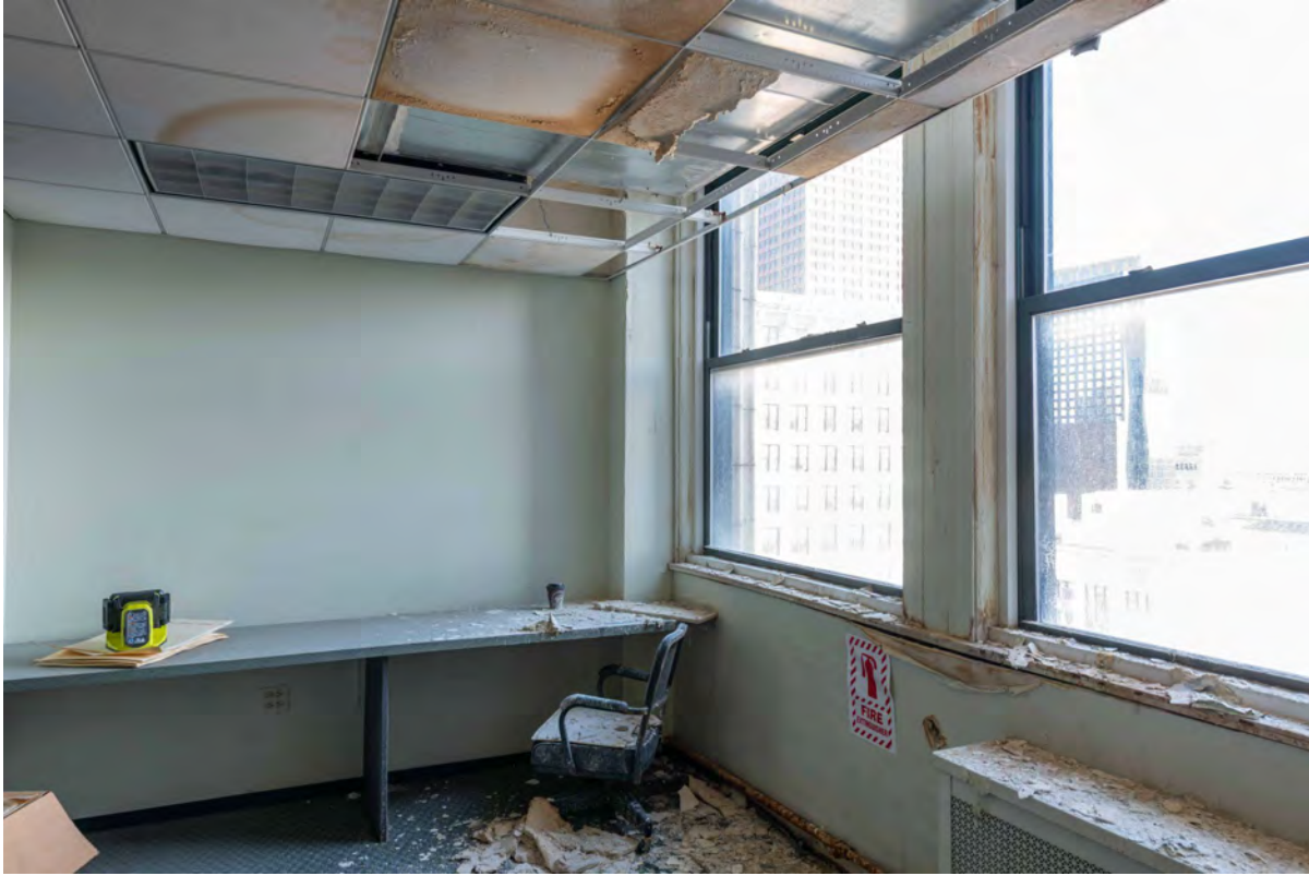
Level 18 Office space
