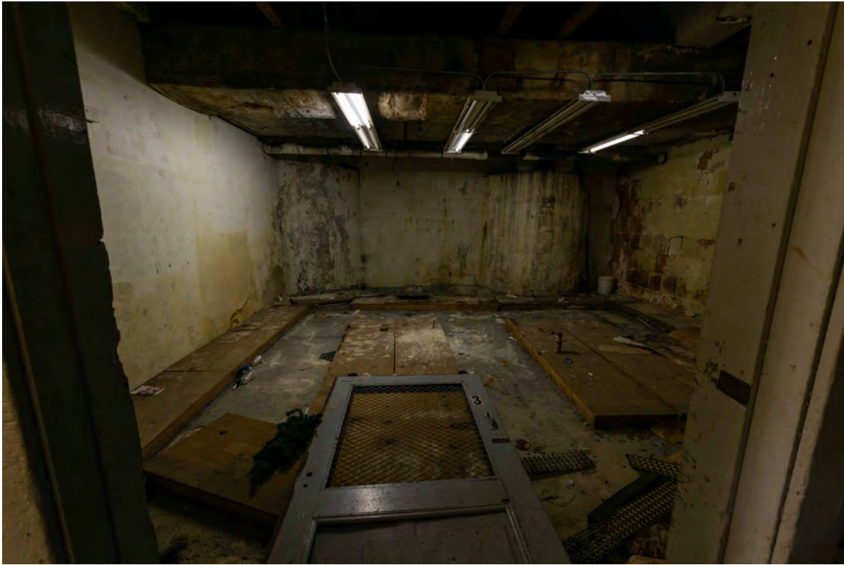
Lower Level 1 Empty Room
