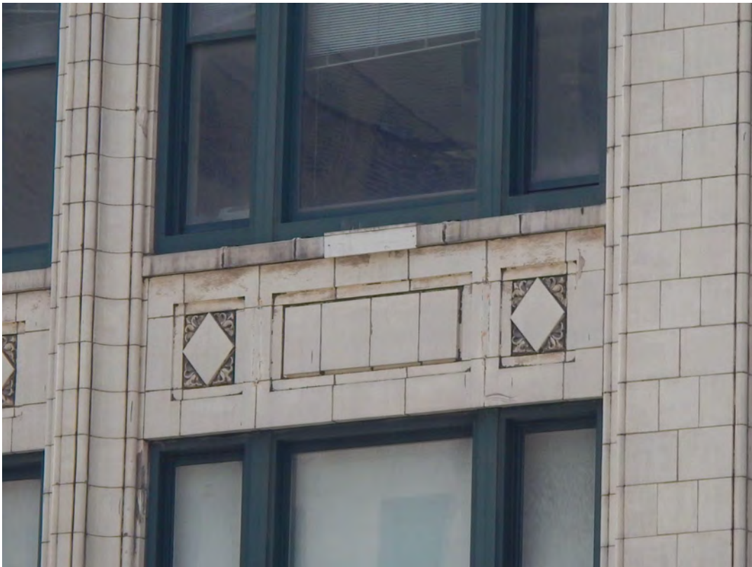
Overview of terra cotta spandrel with previous stabilization effort
