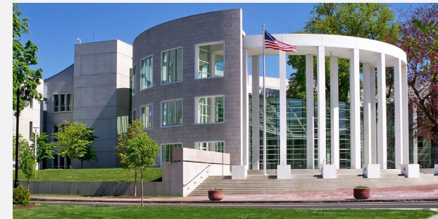
Photos of recently built U.S. Courthouses ( Top to Bottom ): San Antonio, TX | Nashville, TN | Springfield, MA
