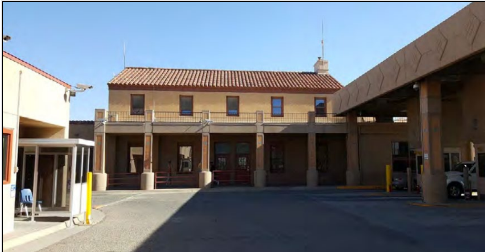
Figure A-5. Historic Main Building – West Facade
