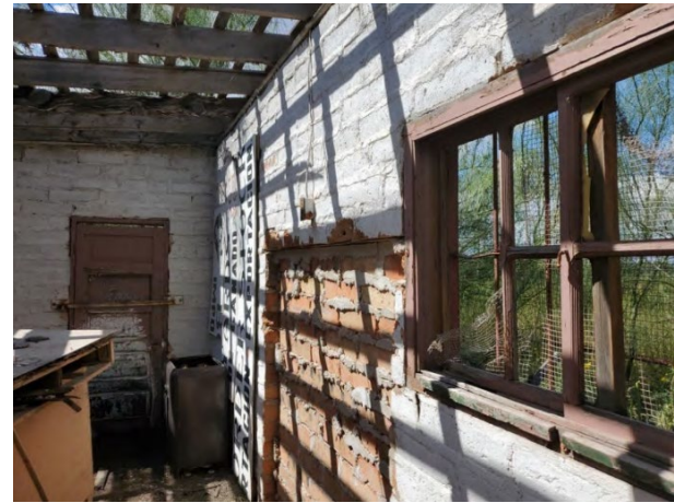
Interior of Cattle Operation Building
