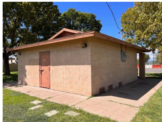
Rear and northern façade
