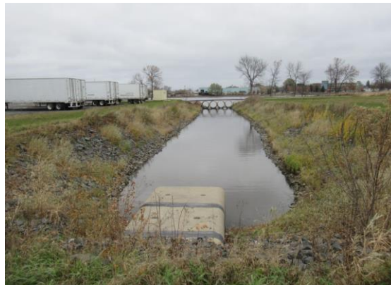
Figure C-6. First Creek, Looking Towards Rainy River
