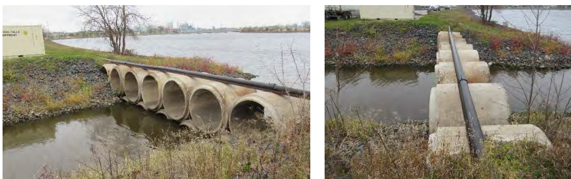
Figure 3.3-3. Leachate Line Crossing First Creek, Near Rainy River
