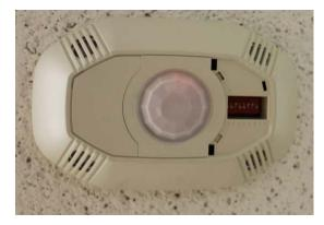
Figure 23 Image of Building 1219, Open Office, Ceiling-Mounted Occupancy Sensor
