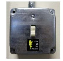
Figure 24 Image of Building 1219, Open Office Manual Switch and Reminder Sticker
