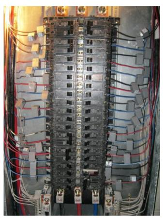
Figure 74 Wireless current sensors installed in an electrical panel in Building 1219
