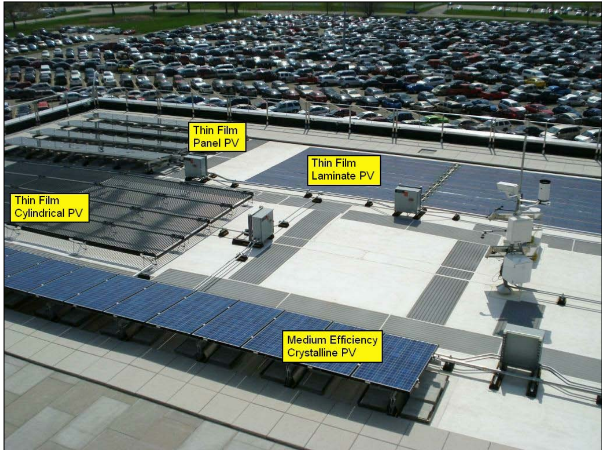
Figure 2: Four Laboratory PV systems at the Bean Federal Center
