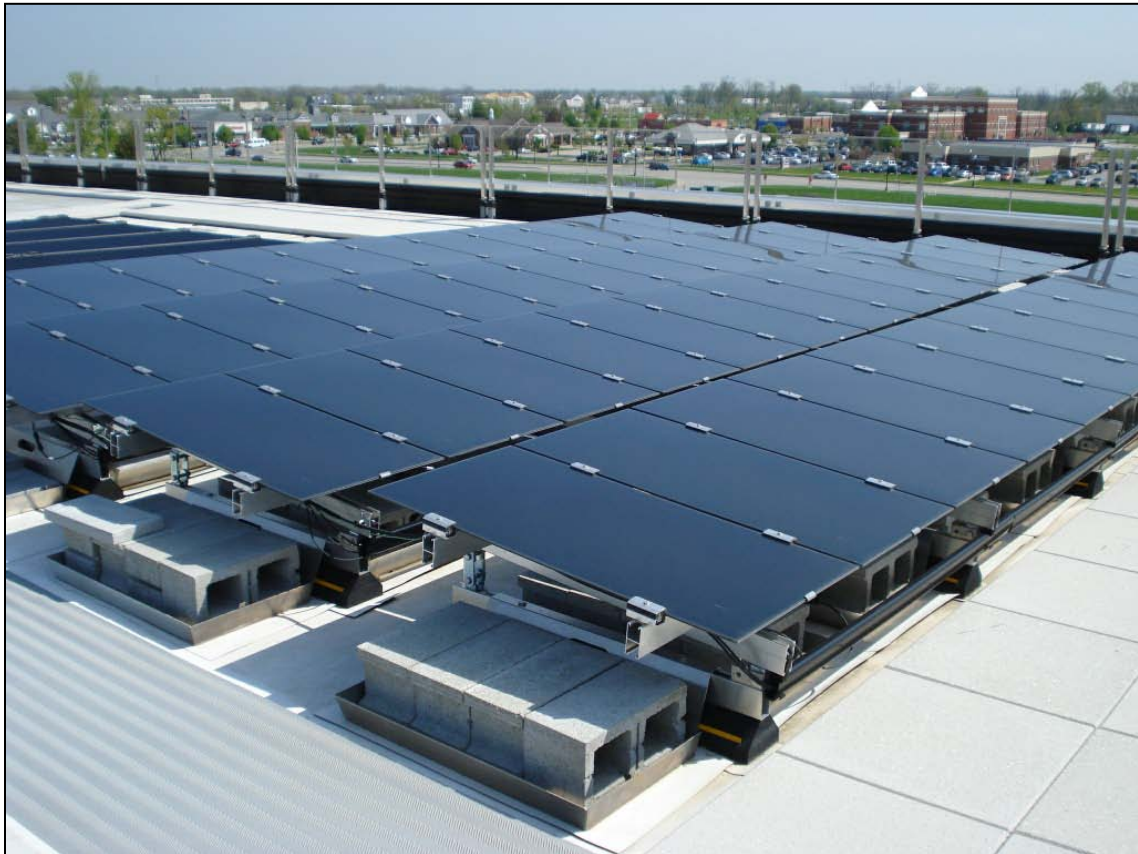
Figure 8: Thin-film CdTe Panel PV Array, Laboratory PV systems, Bean Federal Center
