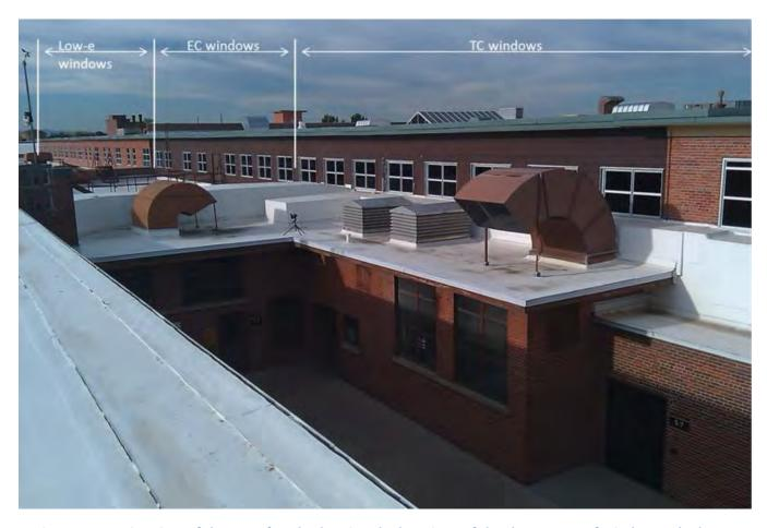
Figure 2: Exterior view of the west façade showing the locations of the three types of windows. The low-e windows were installed in 2005. The electrochromic windows were installed in June 2011. The thermochromic windows were installed at the end of August 2011.
