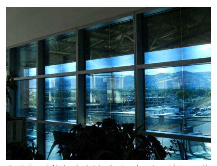
Figure 32: Photograph of the electrochromic window a few minutes after starting to switch. We were unable to obtain images of the windows switching at the Denver Federal Center, but images taken at the National Renewable Energy Laboratory's Research Support Facility [20] illustrate the variation in coloration while switching.
