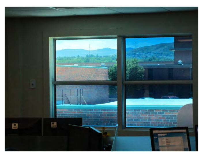
Figure 31: Photograph of an electrochromic window in the perimeter zone during Phase II illustrating the slight differences in tint level between adjacent window panes.
