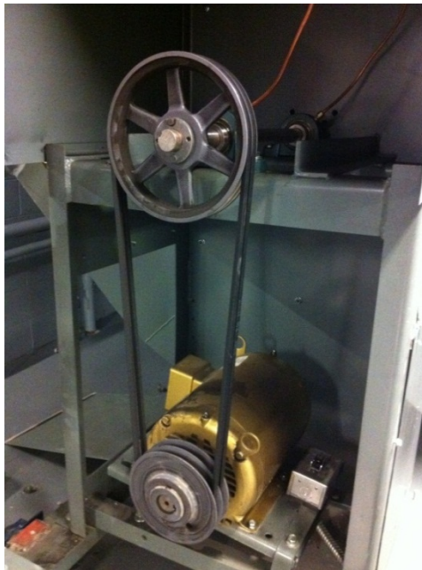
Figure 3 – CV exhaust fan with two standard V-belts. Image Credit: Jesse Dean (NREL)
