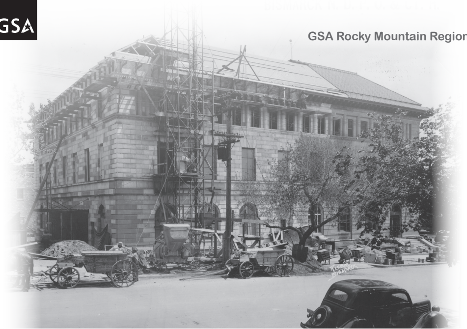
~ FEDERAL BUILDING ~ Bismarck, North Dakota
