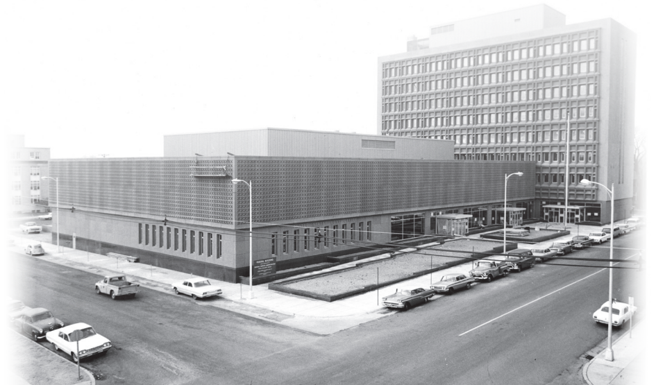
~ JOSEPH C. O'MAHONEY FEDERAL BUILDING/POST OFFICE ~ Cheyenne, Wyoming
