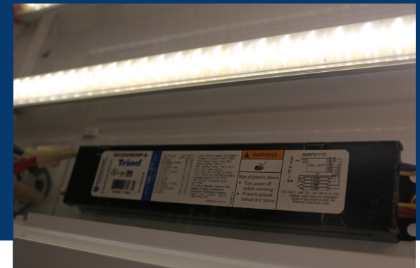
Type A TLED uses the existing ballast. Photo credit Michael Myer, PNNL
