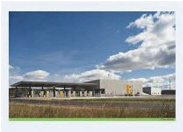
Illustration 10: The canopy has inspection booths and lanes underneath. The canopy is measured and assigned. The booths are measured separately and subtracted from the canopy square footage.
