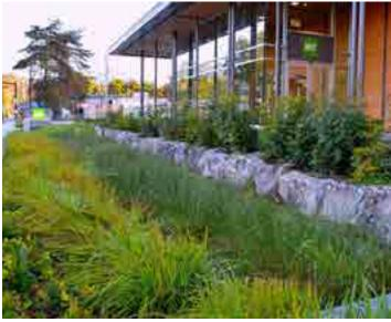
Micro-bioretention along building edges
