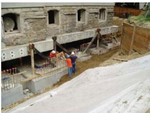
Exterior view of the Pioneer Courthouse being retrofitted with a base isolation system.
