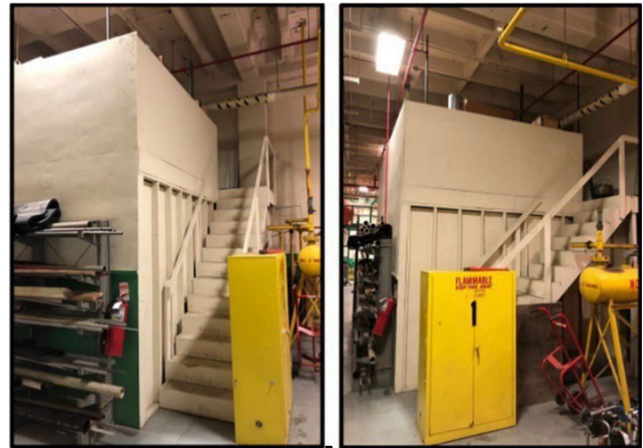
Photographs M1 and M2 Temporary mezzanines
