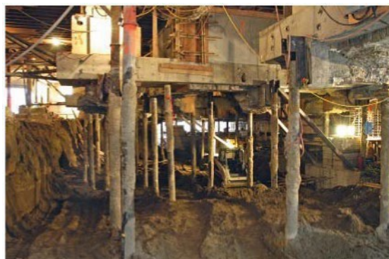
Interior view of the base isolation system being installed at the Pioneer Courthouse.
