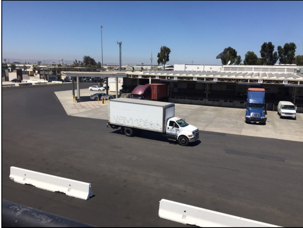
Figure 3.8-1. View of Existing Otay Mesa LPOE Commercial Import Building
