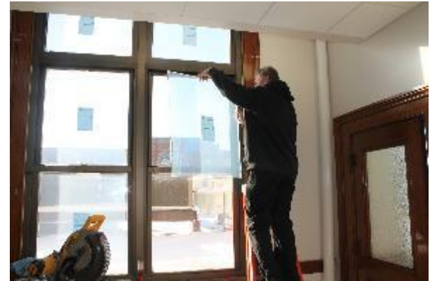
Window lites were pre-measured, and panels were fabricated to size.
