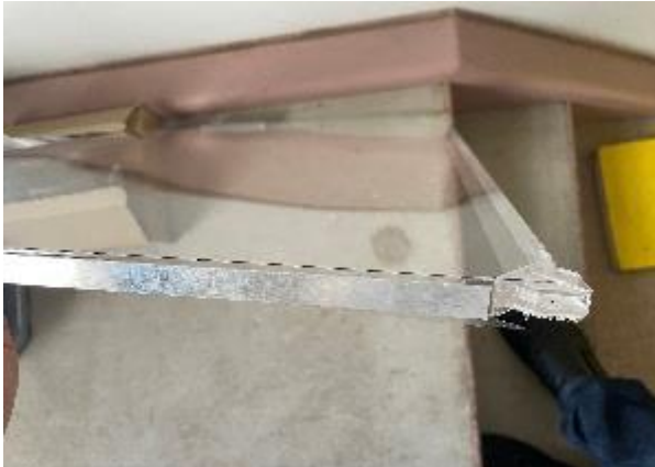
Corners of insulation panels have attachment devices.
