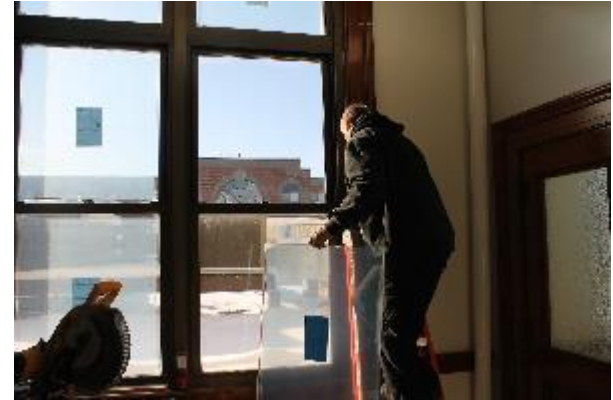
Corner mounts are placed in the corner of each window lite.
