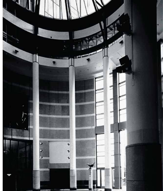
Oakland Federal Building, Oakland, CA
