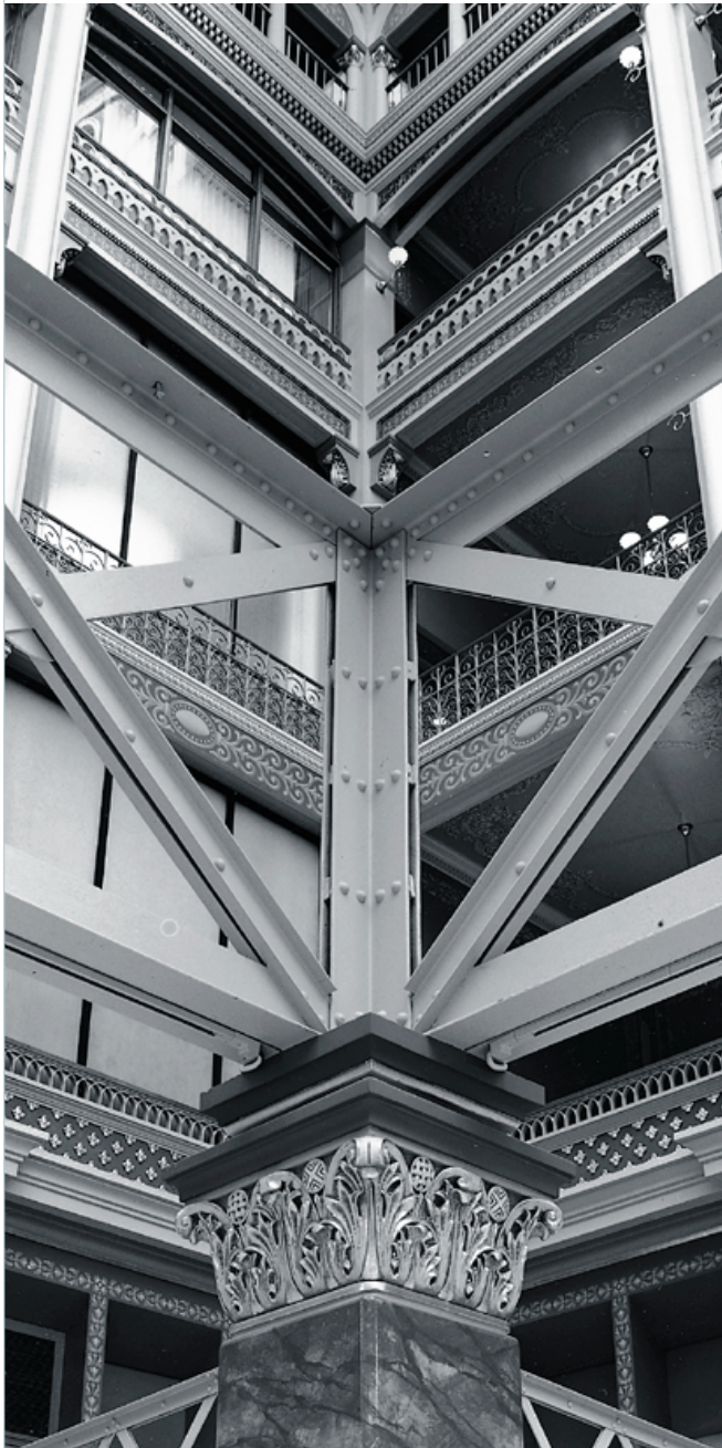
Steel bracing in the Milwaukee Courthouse
