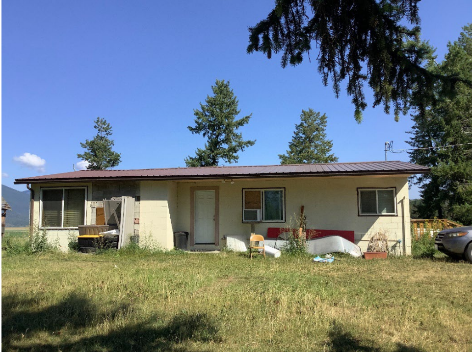
526 Figure 7. Primary façade of 147 Trading Post Road. View toward north.
