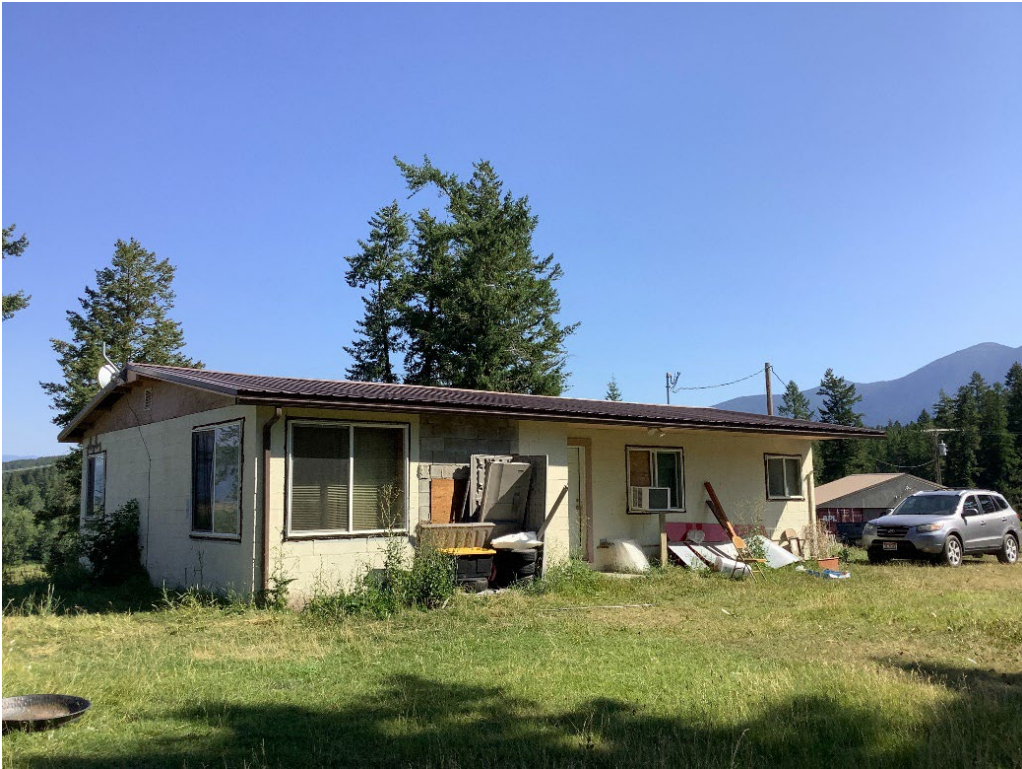
525 Figure 6. 147 Trading Post Road. Oblique view of south and west facing façades.
