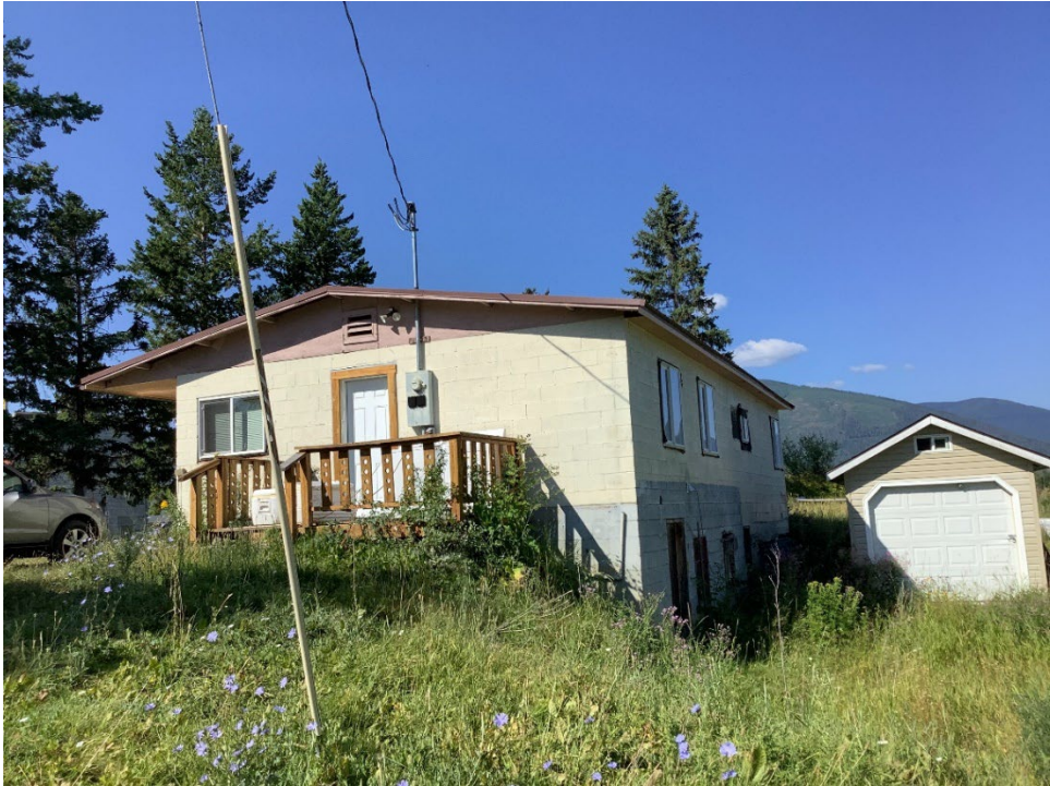
551 Figure 10. Detail of basement concrete block area of 147 Trading Post Road. Oblique view of east and 552 north facing façades. View toward southwest.
