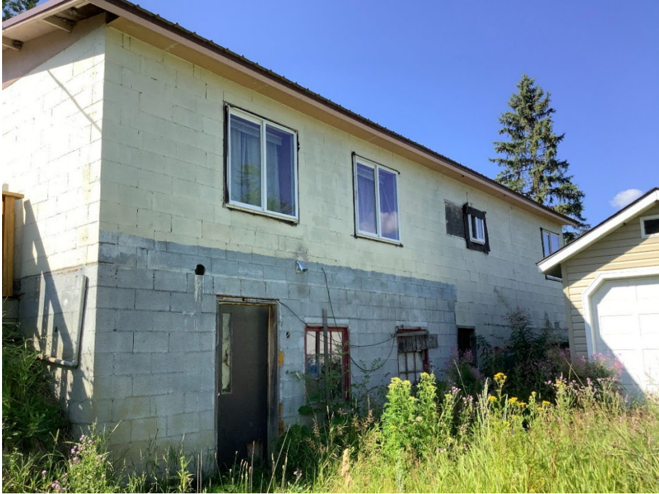
586 Figure 12. North facing rear façade of 147 Trading Post Road. View toward southwest.
