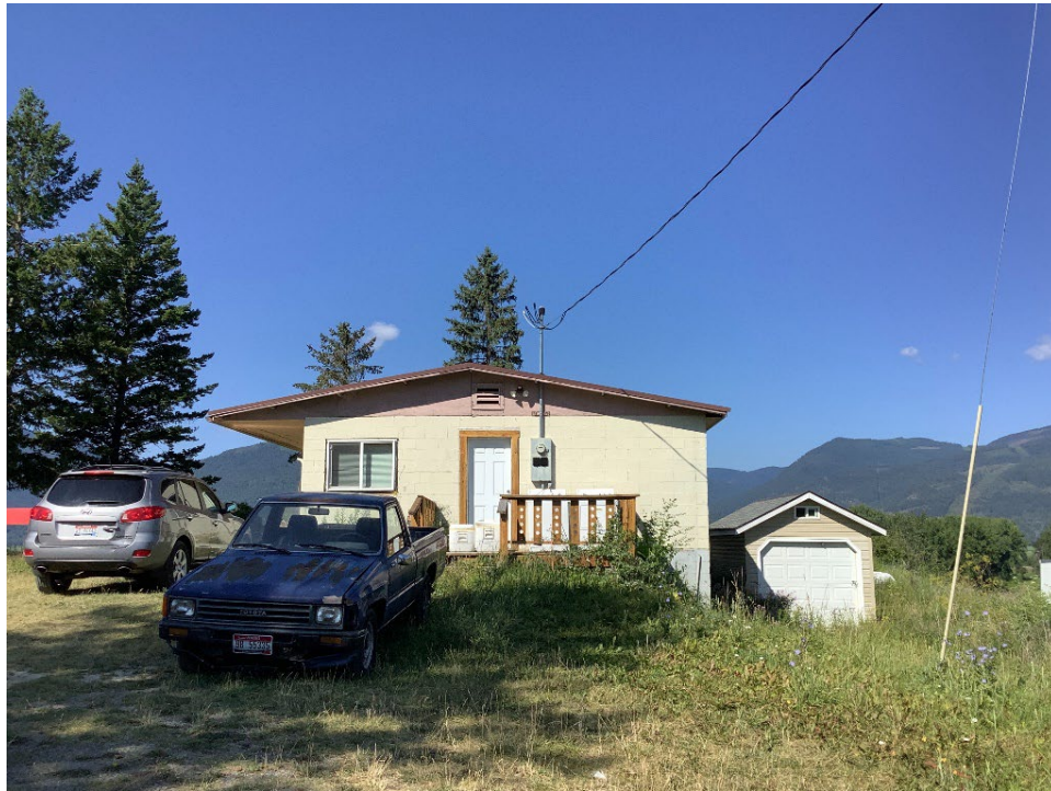
549 Figure 9. East facing façade of 147 Trading Post Road. View toward west.
