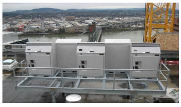
Inverter Platform Constructed by IES
