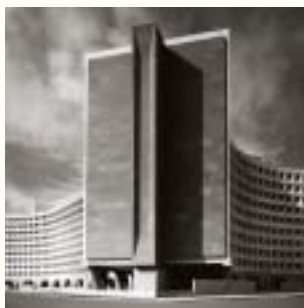
ROBERT C. WEAVER FEDERAL BUILDING U.S. DEPARTMENT OF HOUSING AND URBAN DEVELOPMENT WASHINGTON, DC 1965-1968 MARCEL BREUER
