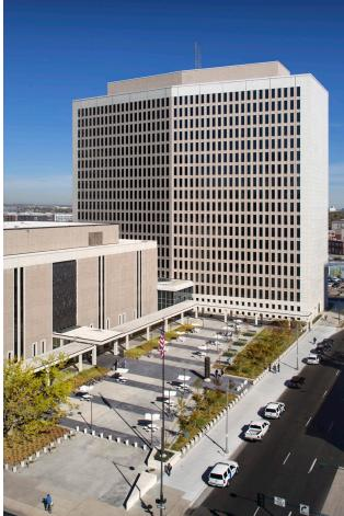
Other energy-saving improvements included increasing the R-value of walls behind the historic pre-cast panels, improving the thermal performance of windows and maximizing daylighting to much of the workspace. Daylighting improves thermal comfort which reduces the mean radiant temperature within a space.
